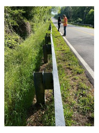
South bound - Reset 4 posts and reattach to existing Wbeam.
