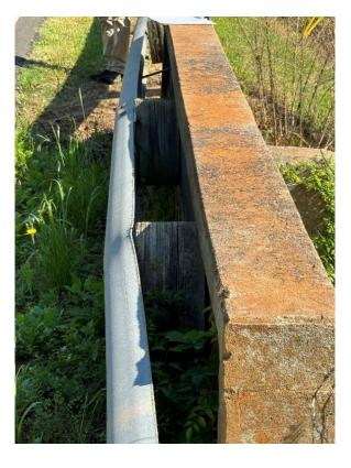
Make T-beam connections on all 4 corners of the concrete parapet of culvert headwall.
