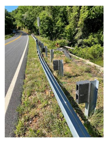
Remove & replace ±75 damaged W-Beam system. Reset 1 additional post. Replace an additional 4 offset blocks at various locations.
