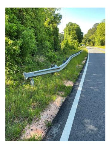
North bound departure end – Remove and replace guardrail departure, Type 1 and 25' section Wbeam system.
