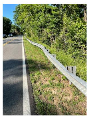
Sound bound - Replace 75' of damaged W-beam system.
