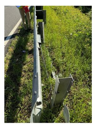
North bound approach - Reattach end section. Reset/replace second to last post.
