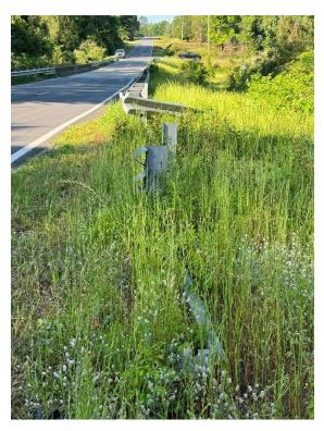
South bound approach - Replace approach terminal (type 12) of guardrail.
