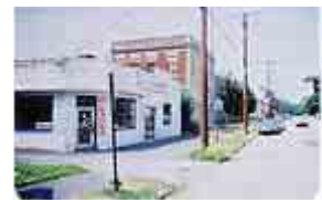
A former drycleaners. Such sites present high potential risk in any vapor intrusion
