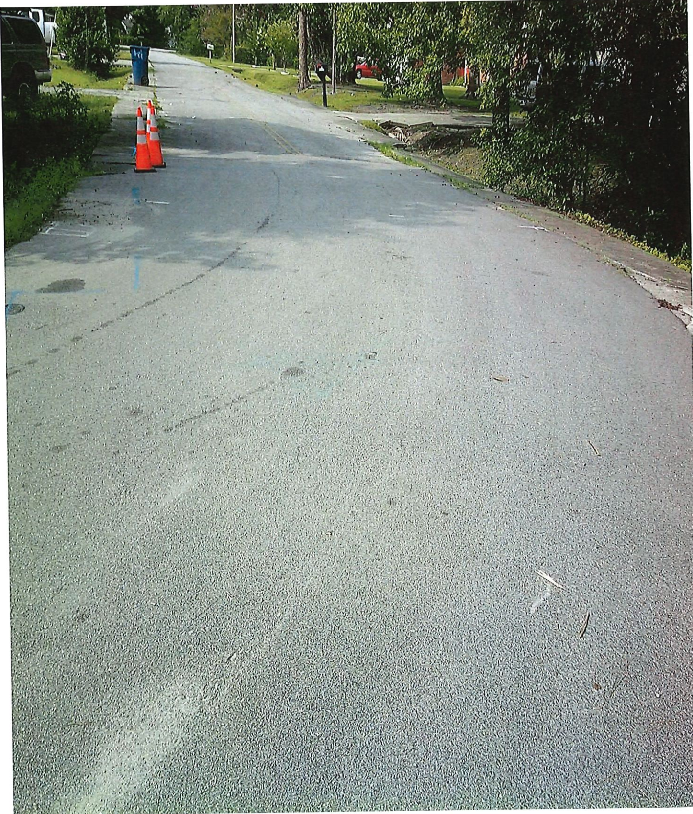
Figure 2: Picture of the work area:
