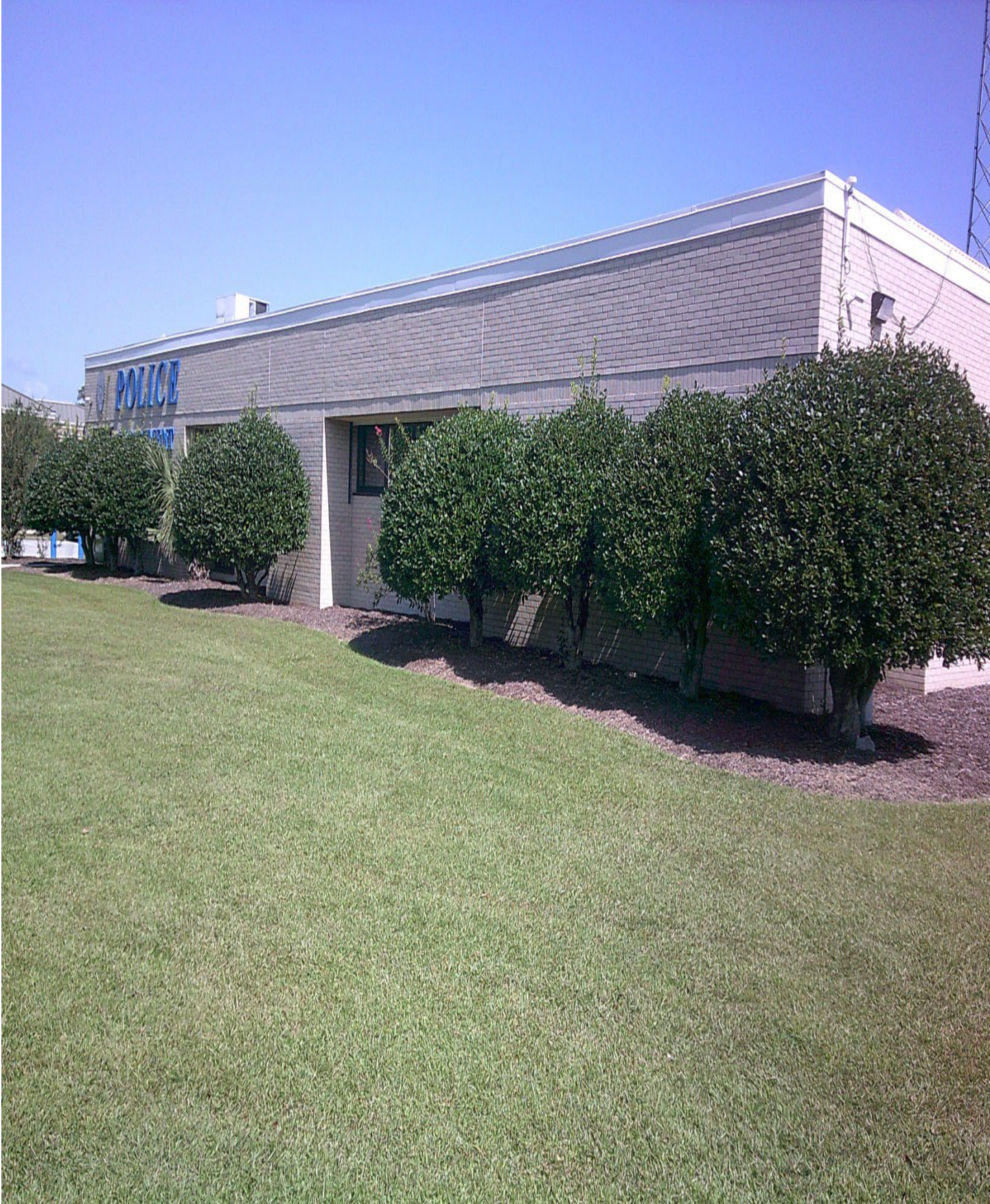
Figure 2: West Side of Building
