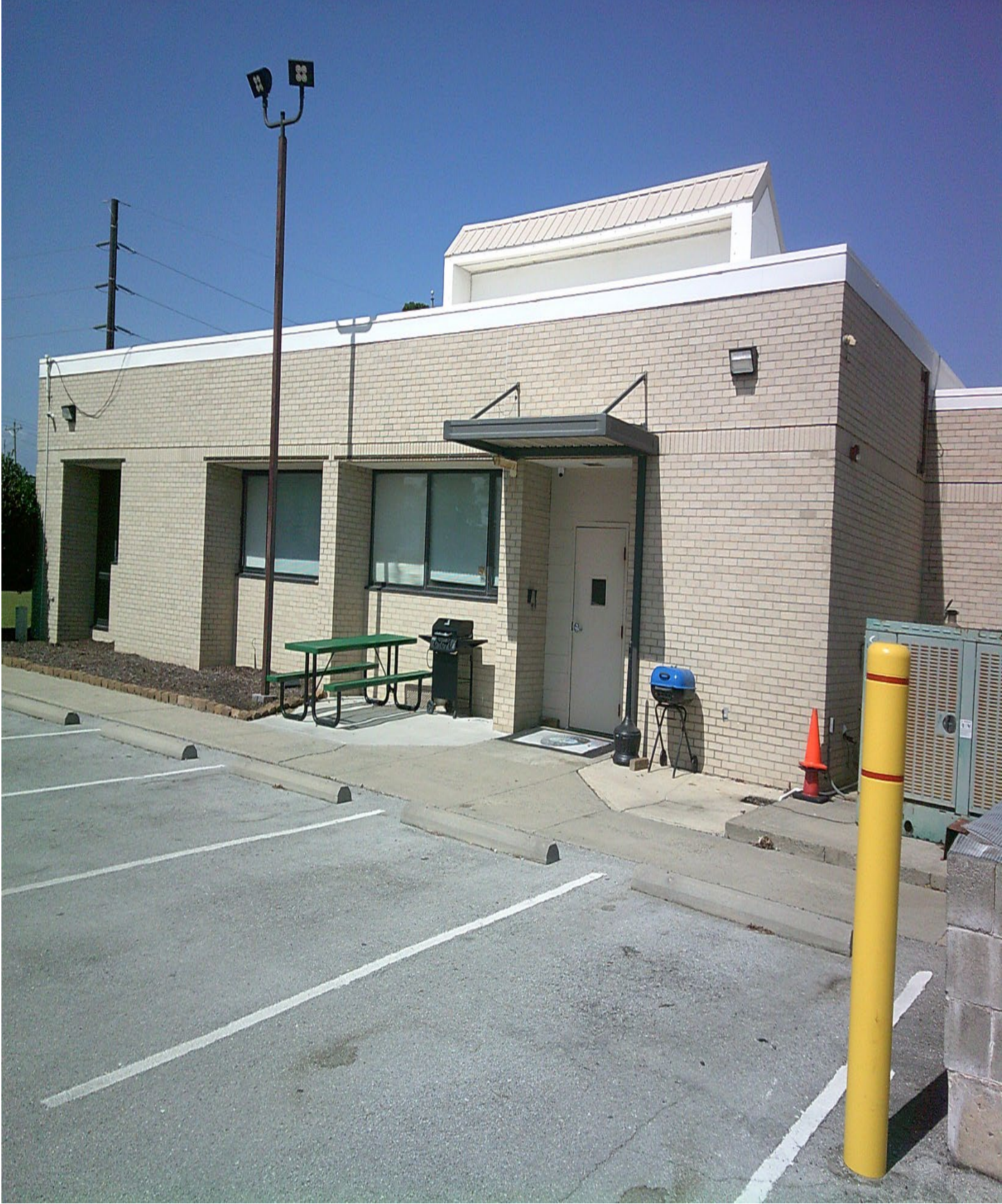
Figure 4: South Side of Building
