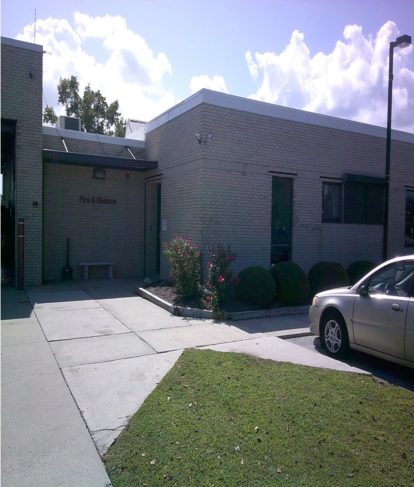
Figure 3: East Side of Building
