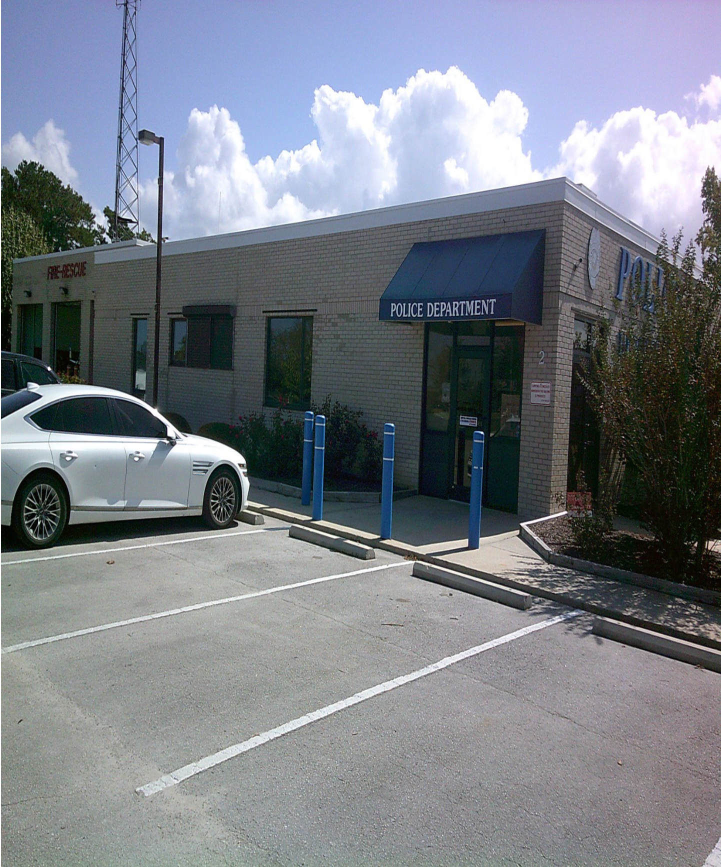
Figure 1: North Side / Front of Building
