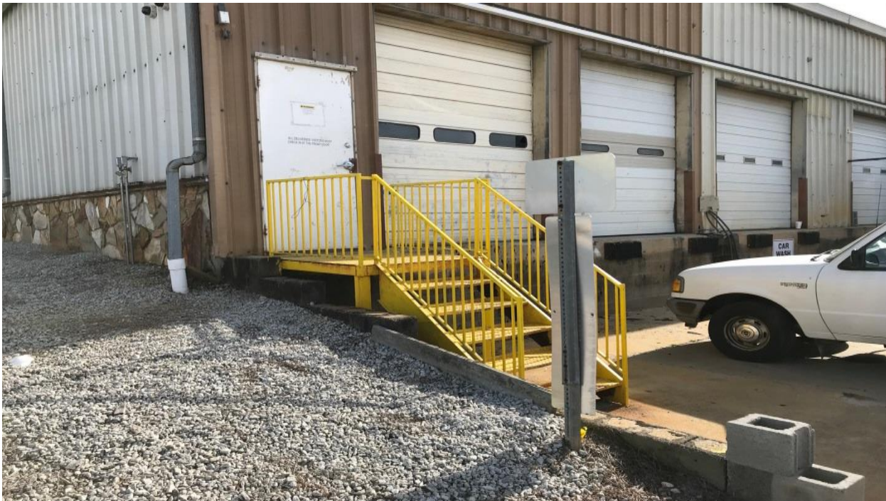
Paint Stairwells GDOT yellow
