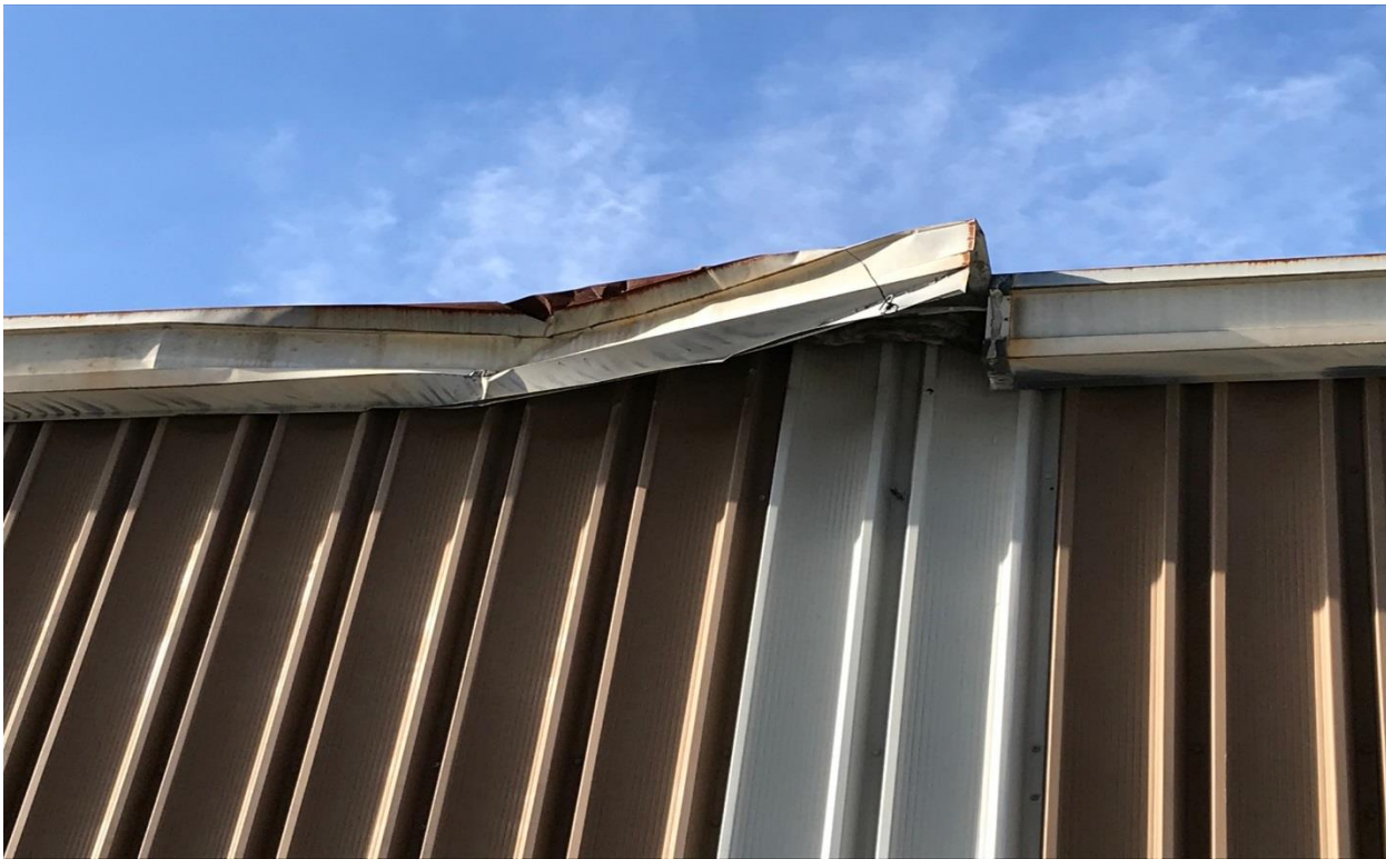
Replace Damaged Metal Framing
