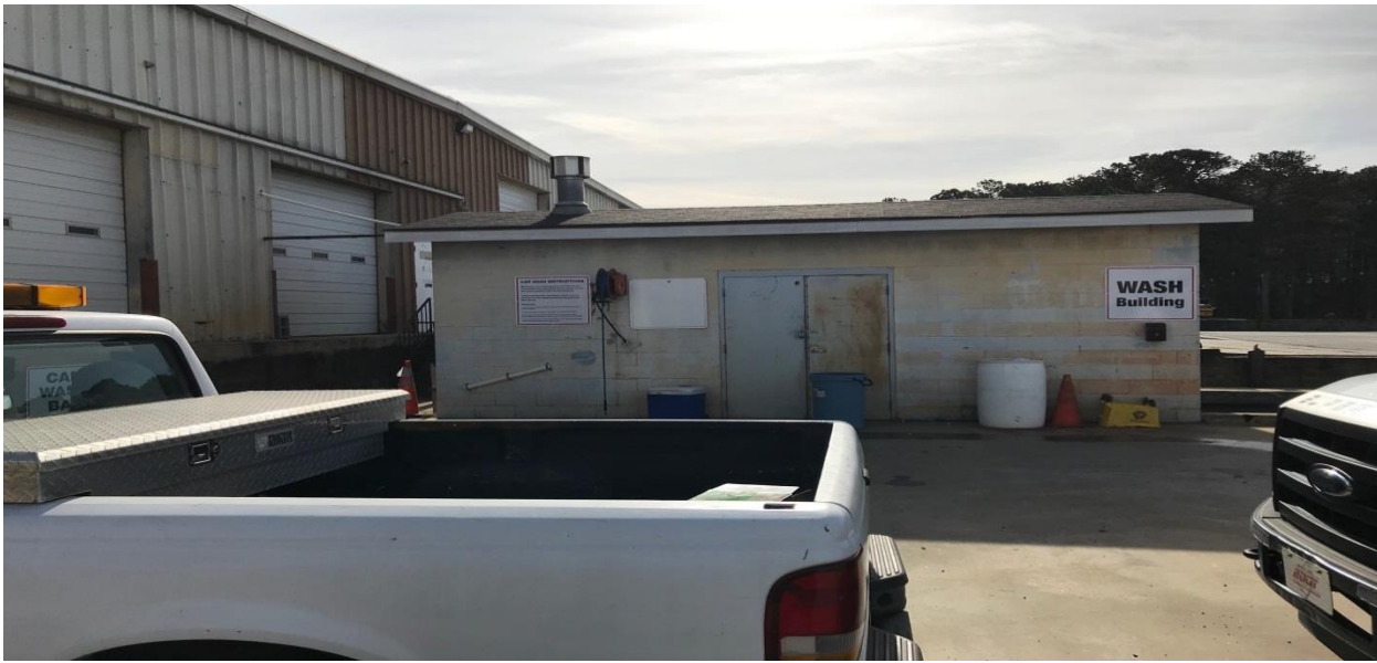
Clean and Paint Wash Building
