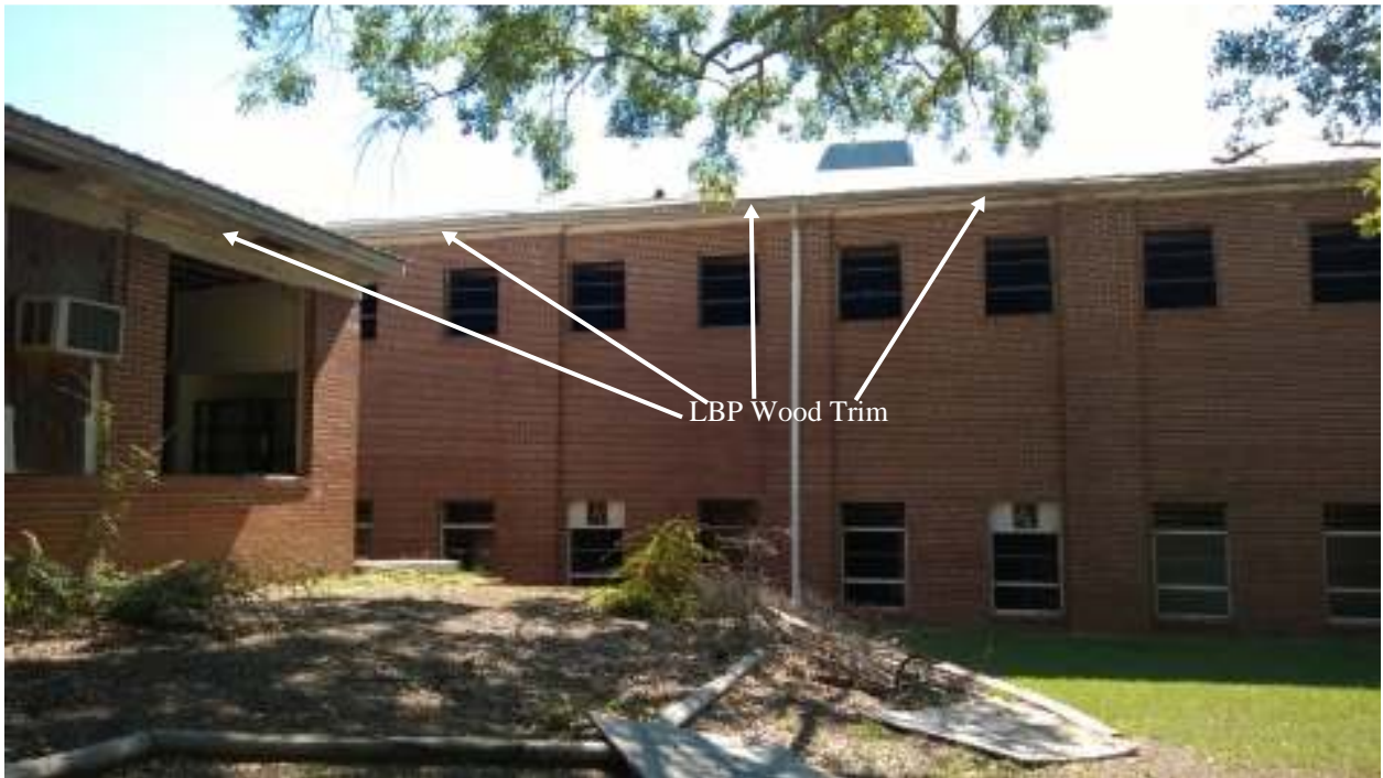
Photo #4: Exterior Side B of Bldg. 5010 LBP locations.
