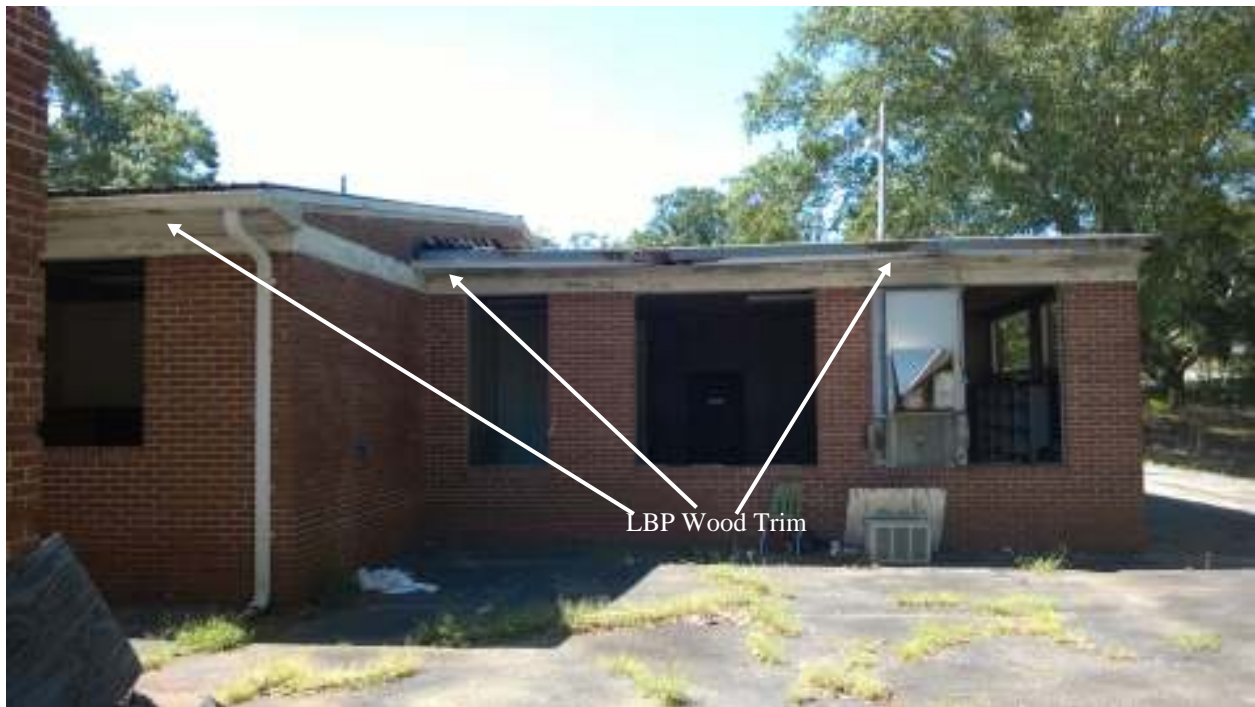
Photo #2: Exterior Side C of Bldg. 7010 LBP locations.
