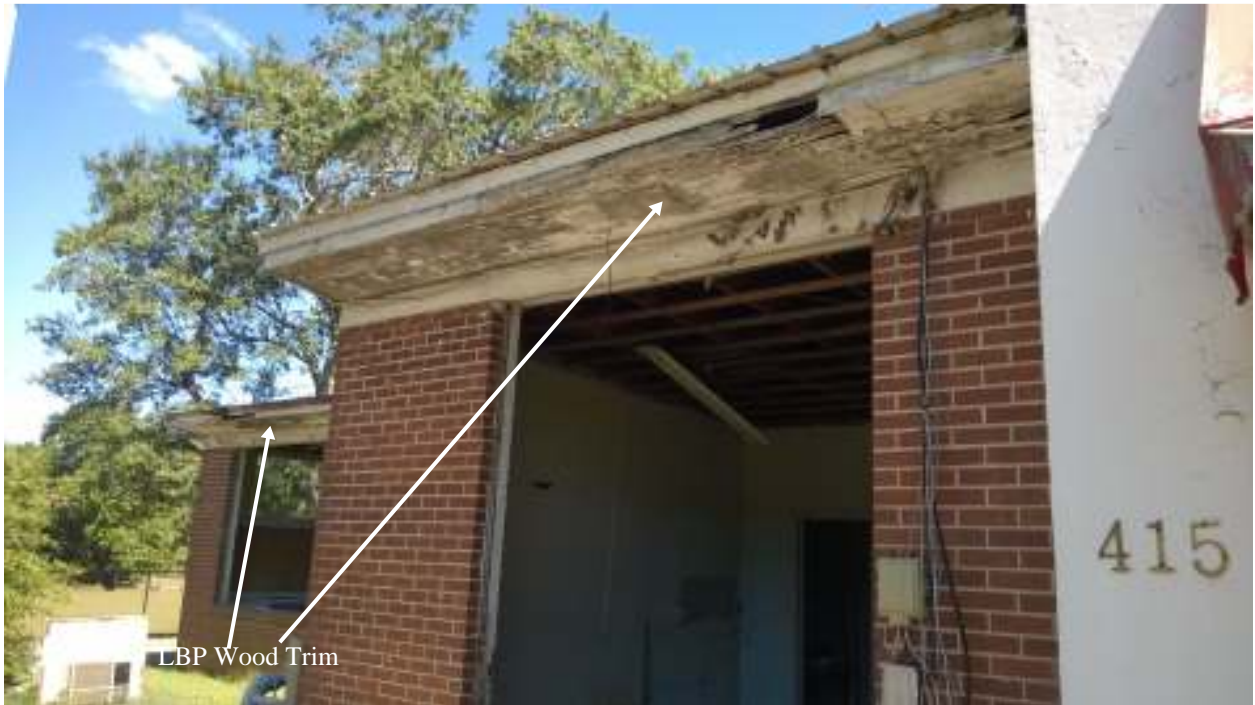
Photo #3: Exterior Side A of Bldg. 7010 LBP locations.
