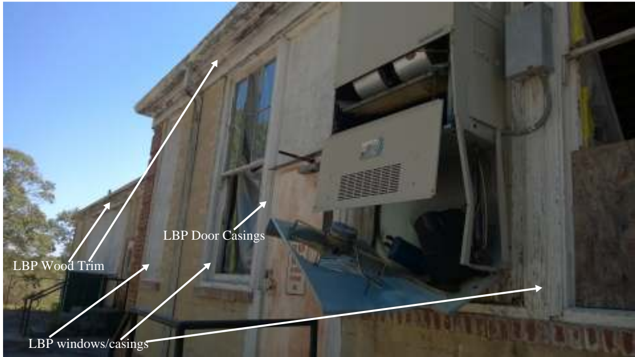
Photo #1: Exterior Side B of Bldg. 8010 LBP locations.
