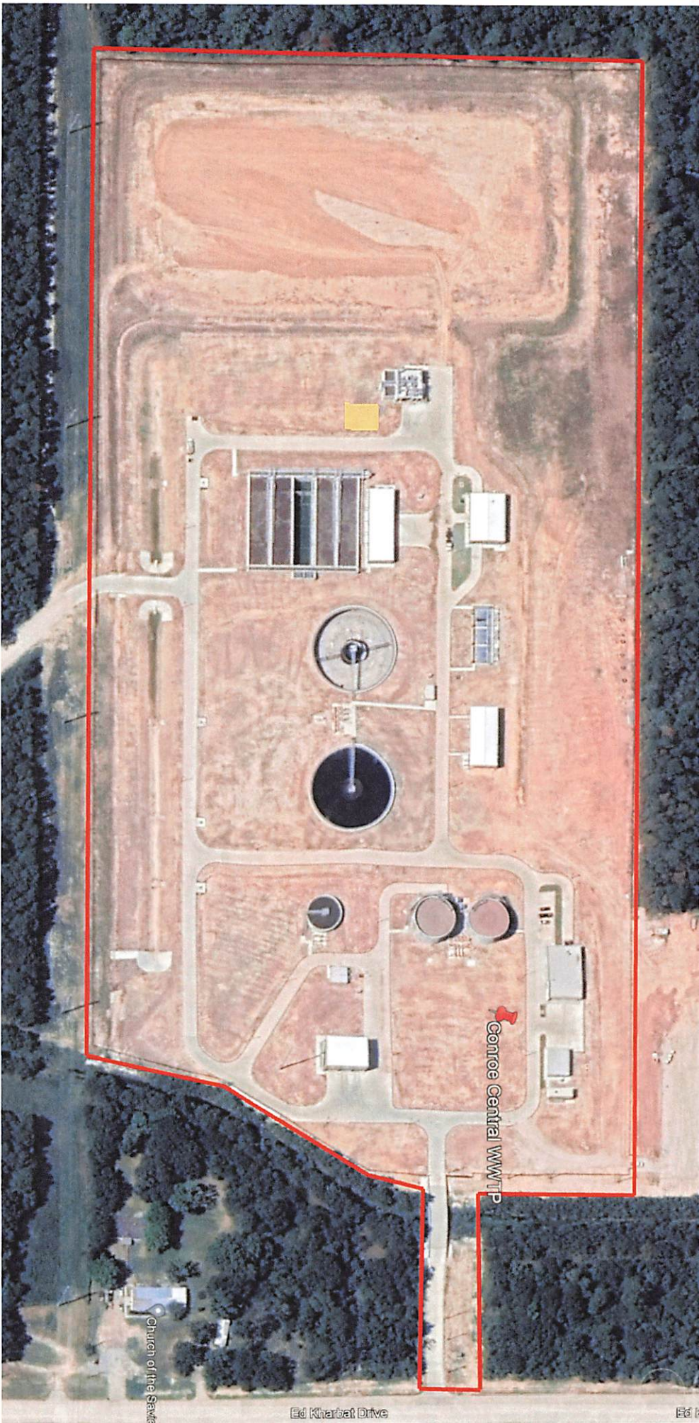
Conroe Central Wastewater Treatment Plant 1890 Ed Kharbat Dr Approx. 25 acres
