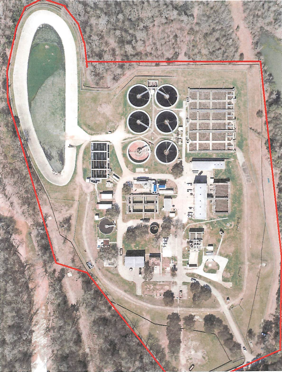
Southwest Wastewater Treatment Plant 2400 Sgt Ed Holcomb Blvd S Approx. 25 acres
