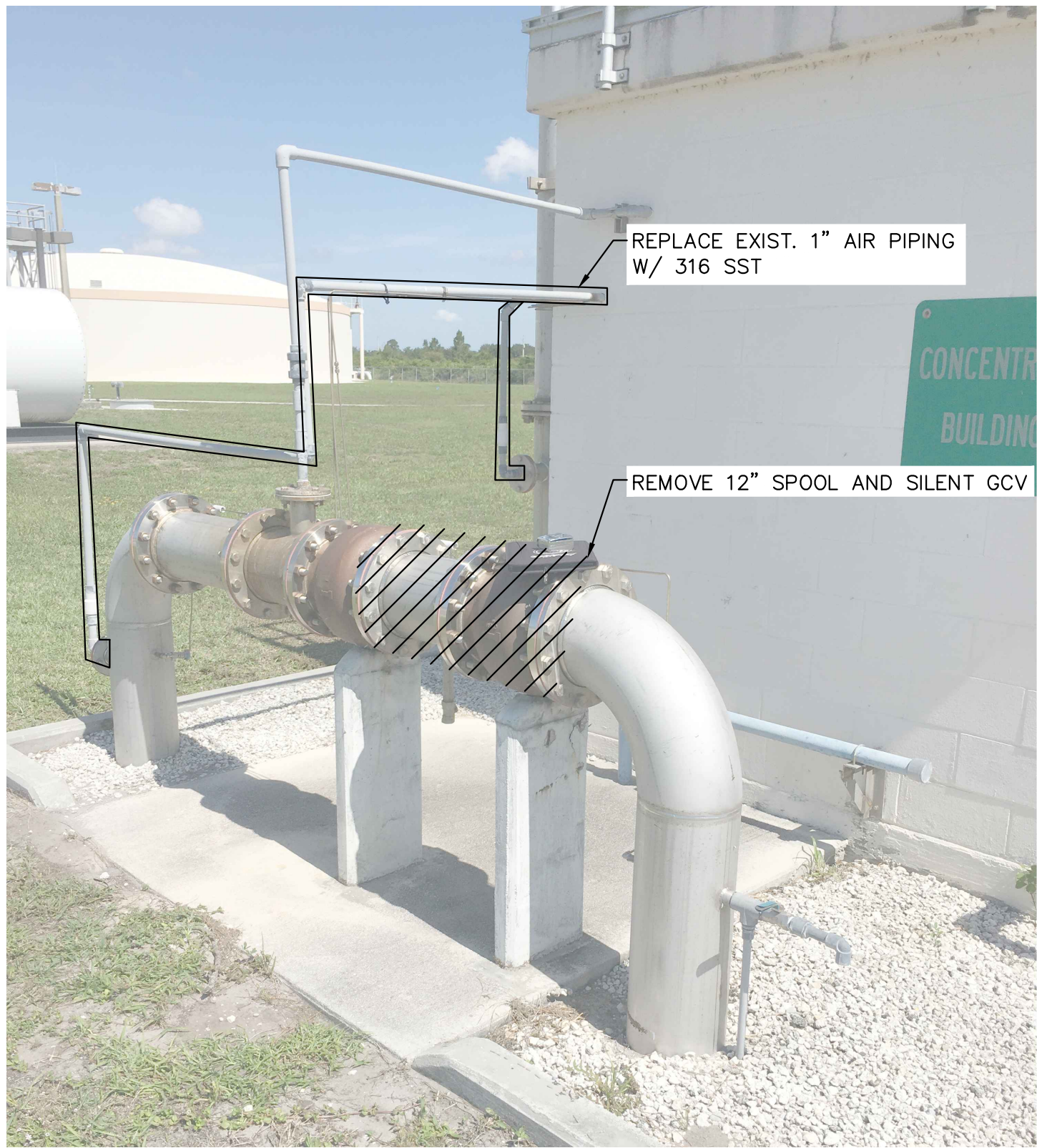
PHOTO #1-ABOVE GROUND PIPING TO REMAIN N.T.S.
