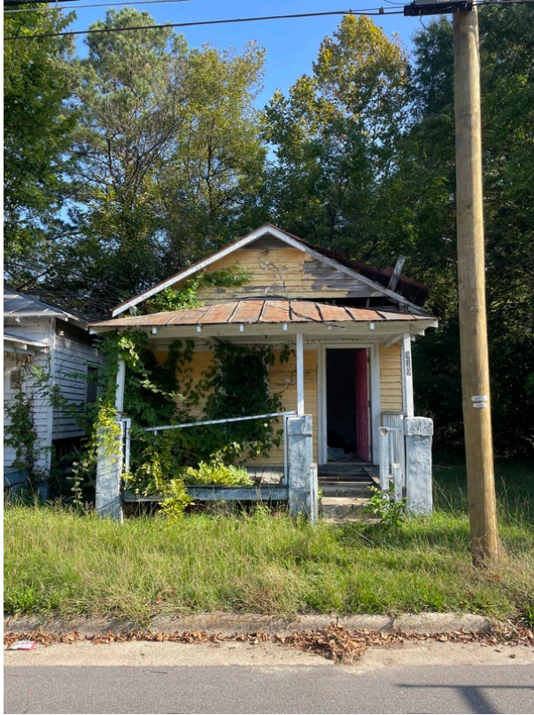
View of the residential structure located at 929 Carolina Street
