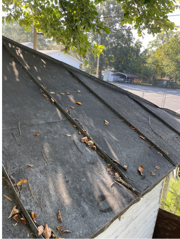
View of asbestos-containing Silver Paint Coating (HA 927-3)
