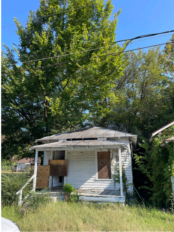
View of the residential structure located at 927 Carolina Street
