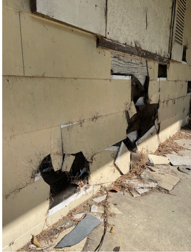
View of asbestos-containing Transite Siding (HA 209-1)
