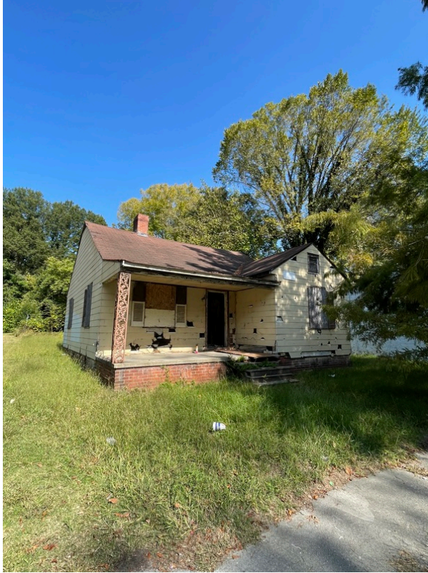
View of the residential structure located at 209 Maplewood Avenue
