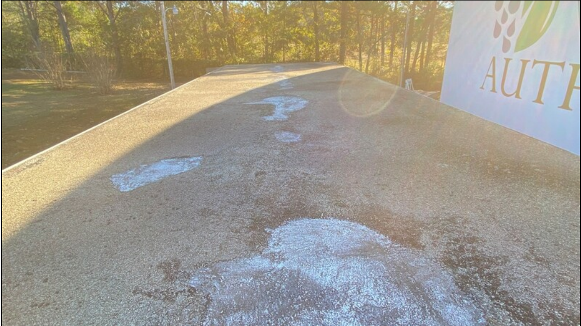
7 - View of the roof of Building 1
