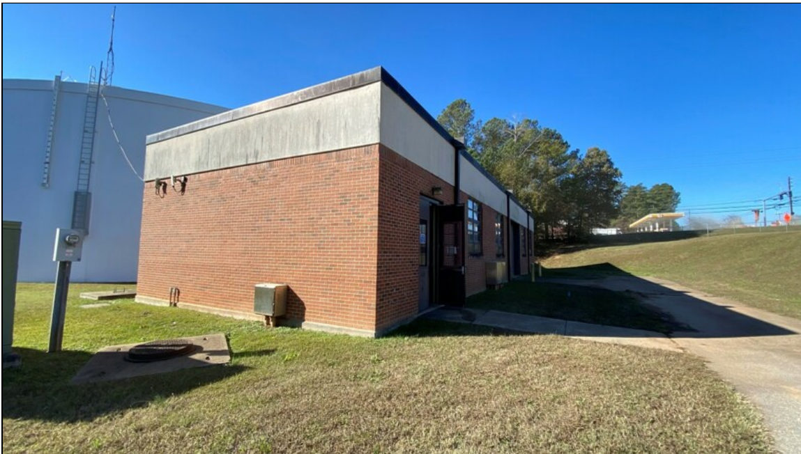
2 - View of Noah's Ark Building 2
