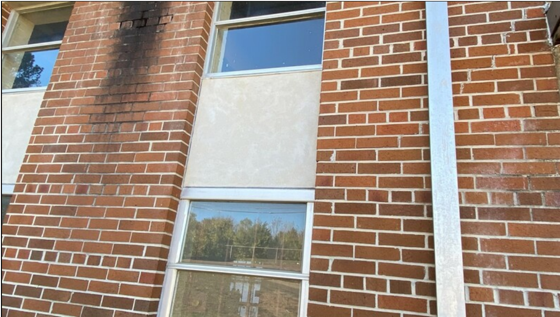
5 - View of the wall panels
