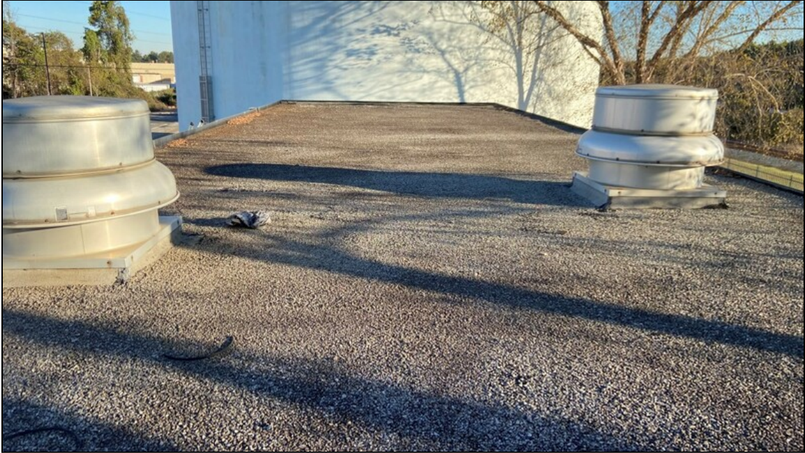
7 - View of the roof
