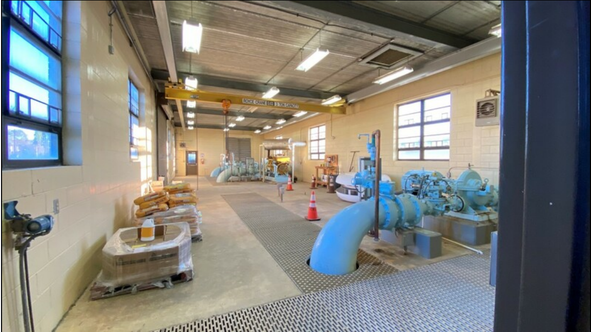
5 - View of the interior of the building
