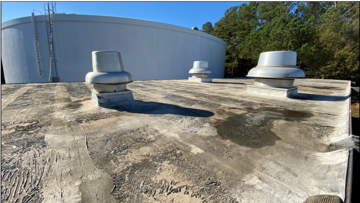
8 - View of the roof of Building 2
