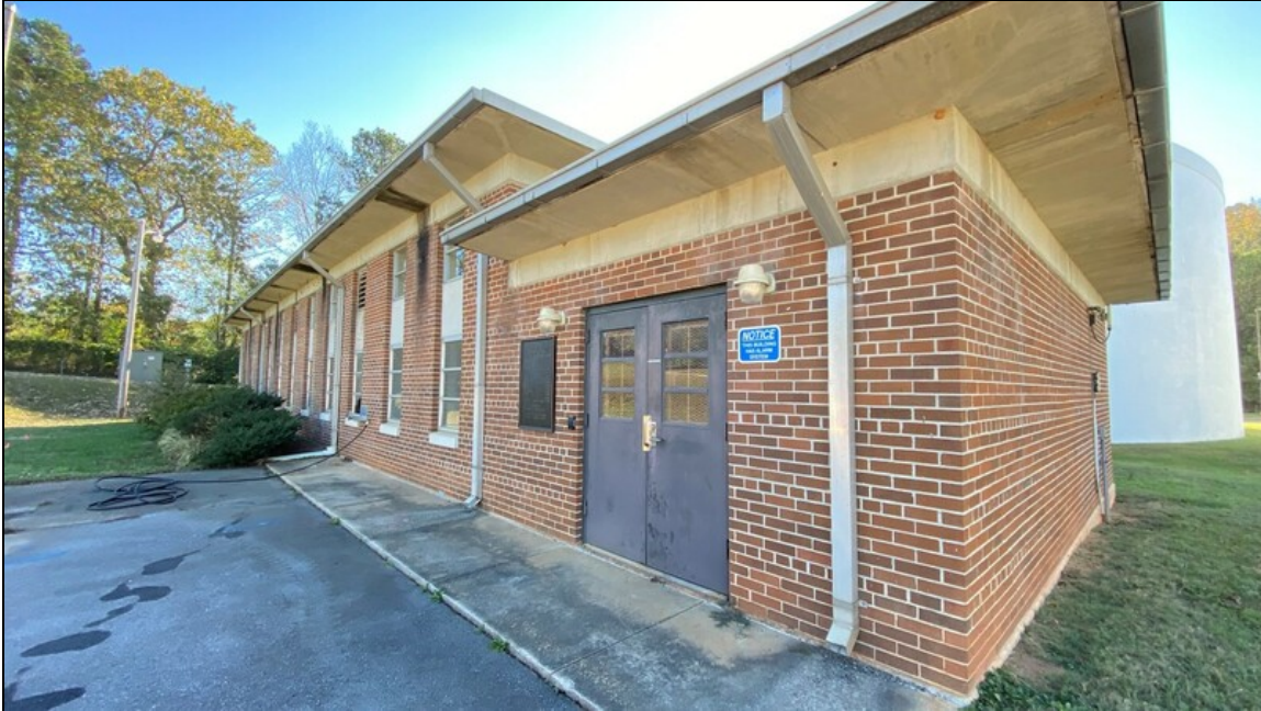
1 - View of Noah's Ark Building 1
