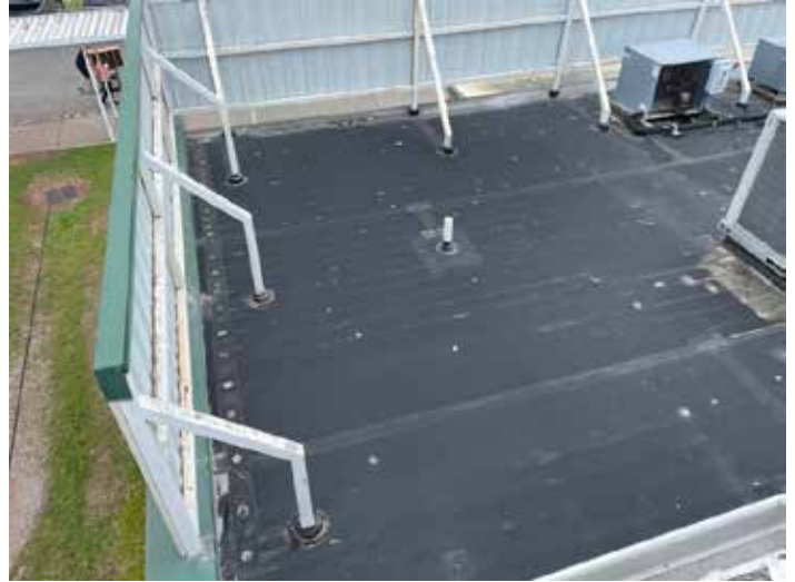
Overview of the EPDM section.
