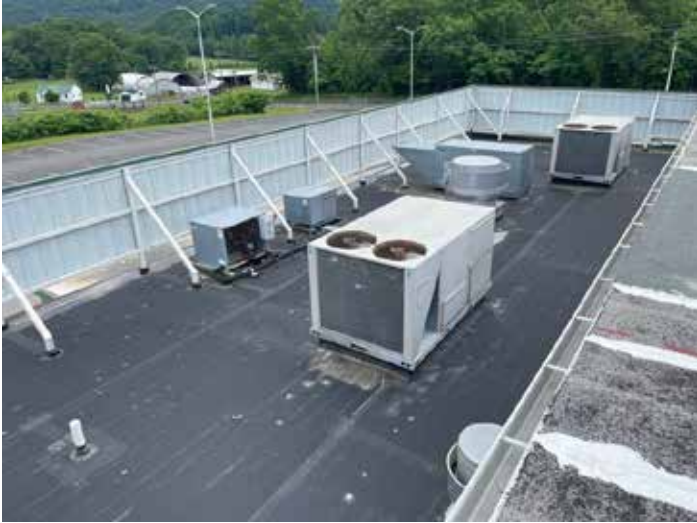
Overview of the EPDM section.
