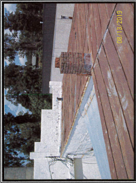
Photo #9 Northeast-facing view of Sheet Metal Roofing System over Areas 1 & 2 (Rusted)
