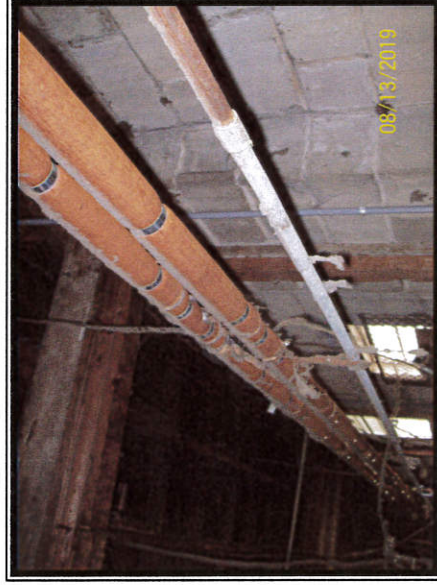
Photo #20 No Asbestos Detected in Any Pipe Wrap Materials
