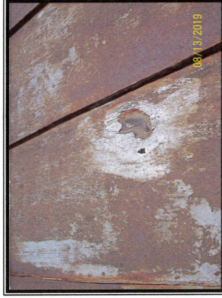
Photo #10 Asbestos Detected at >1% in Metal Roof Seam Caulk of Areas 1 & 2
