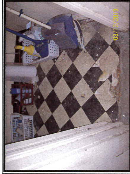
Photo #2 Asbestos Detected at >1% in Parquet Flooring; No Asbestos Detected in Mottled Gray Flooring
