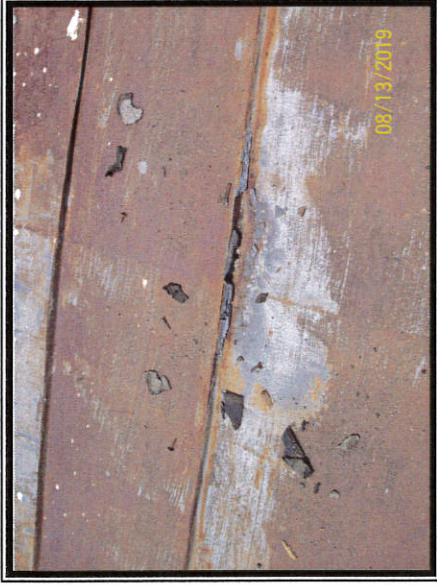
Photo #10 Asbestos Detected at >1% in Metal Roof Seam Caulk of Areas 1 & 2
