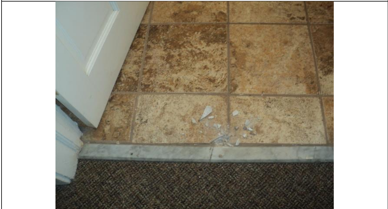
Homogeneous Material No. 12 – Non-ACM Mottled Dark Brown CT with Tan Grout and White Setting Base located in Bathroom 2-1
