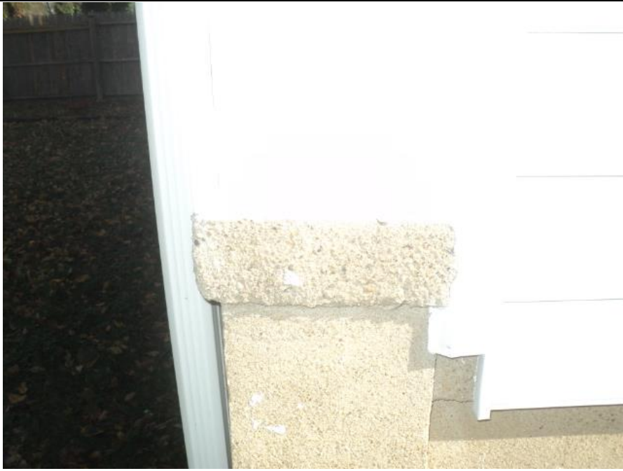
Homogeneous Material No. 17 – Non-ACM White Vinyl Siding Seam Caulk located on the Exterior Siding
