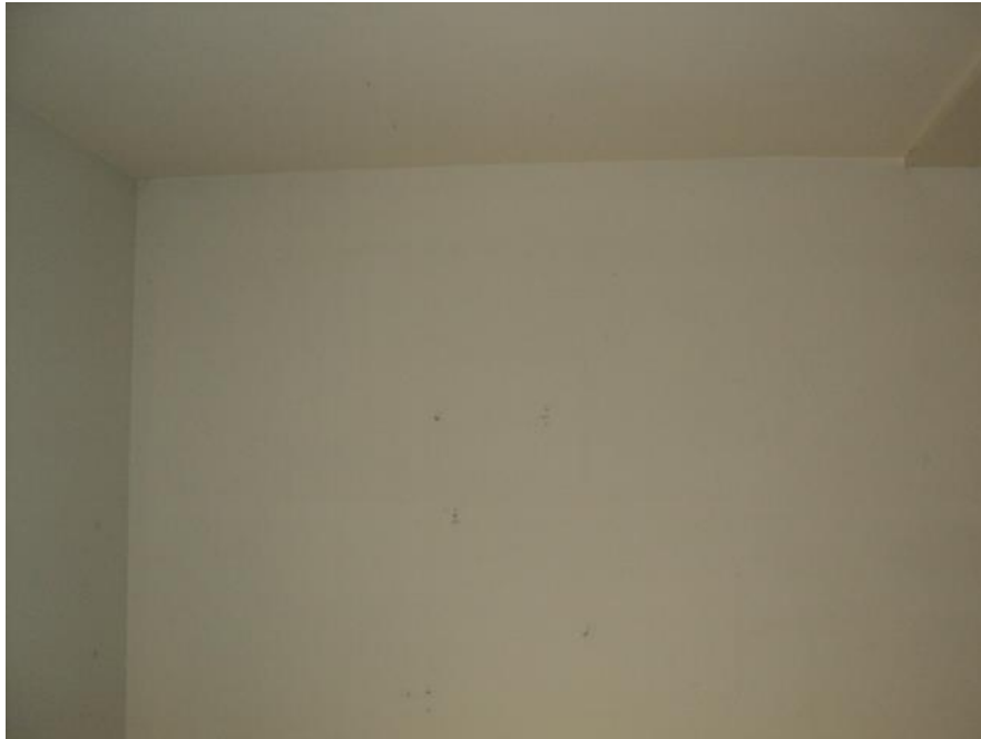
Homogeneous Material No. 2 – Non-ACM White Wall DW and Associated White JC located Throughout the Building including Dining Room, Bedroom 2-2 and Bedroom 3-2
