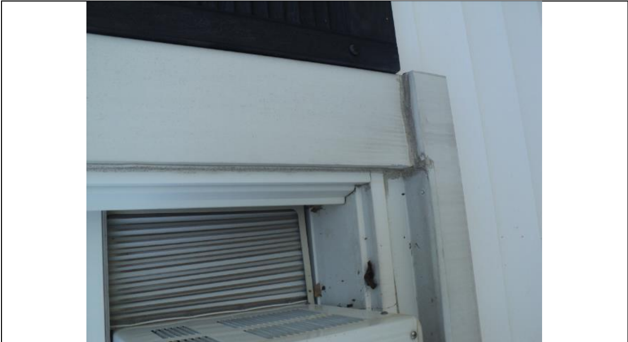
Homogeneous Material No. 15 – Non-ACM White Exterior Window Caulk located in the Exterior Windows
