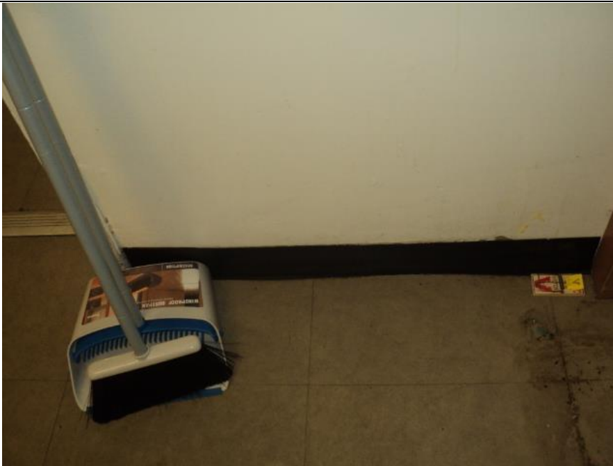
Homogeneous Material No. 6 – Non-ACM 4" Black Vinyl Cove Base with Cream Mastic Located in the Kitchen
