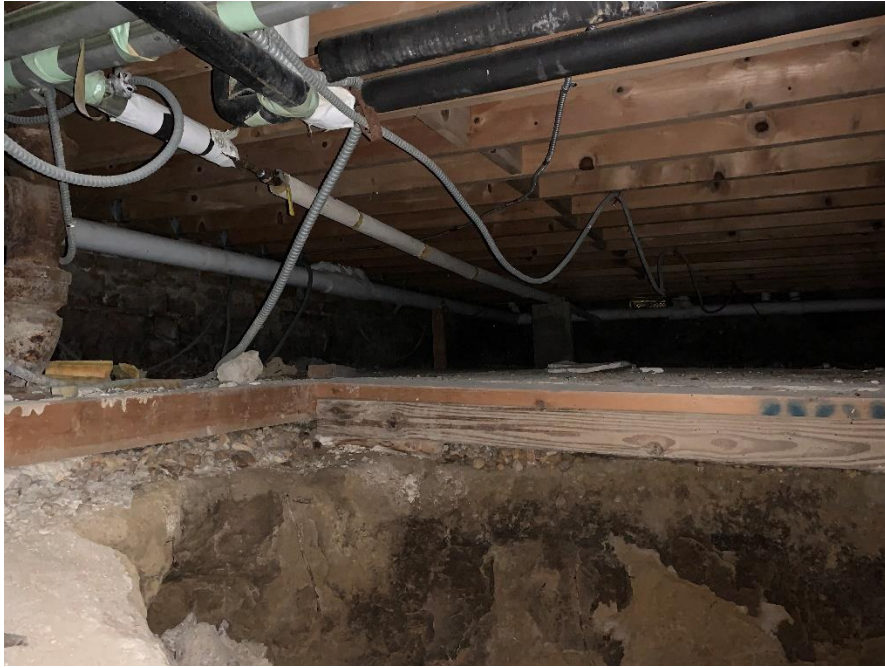
Non-ACM Fiberglass Insulation on Piping in Basement
