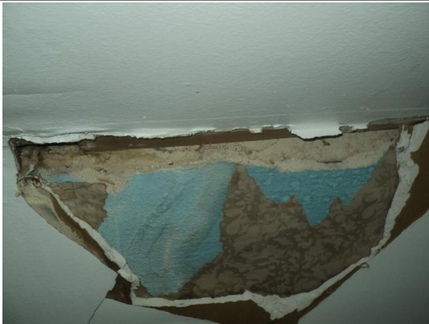
Homogeneous Material No. 14 – Non-ACM Tan Ceiling Plaster located in Bedrooms 3-1 and 3-2
