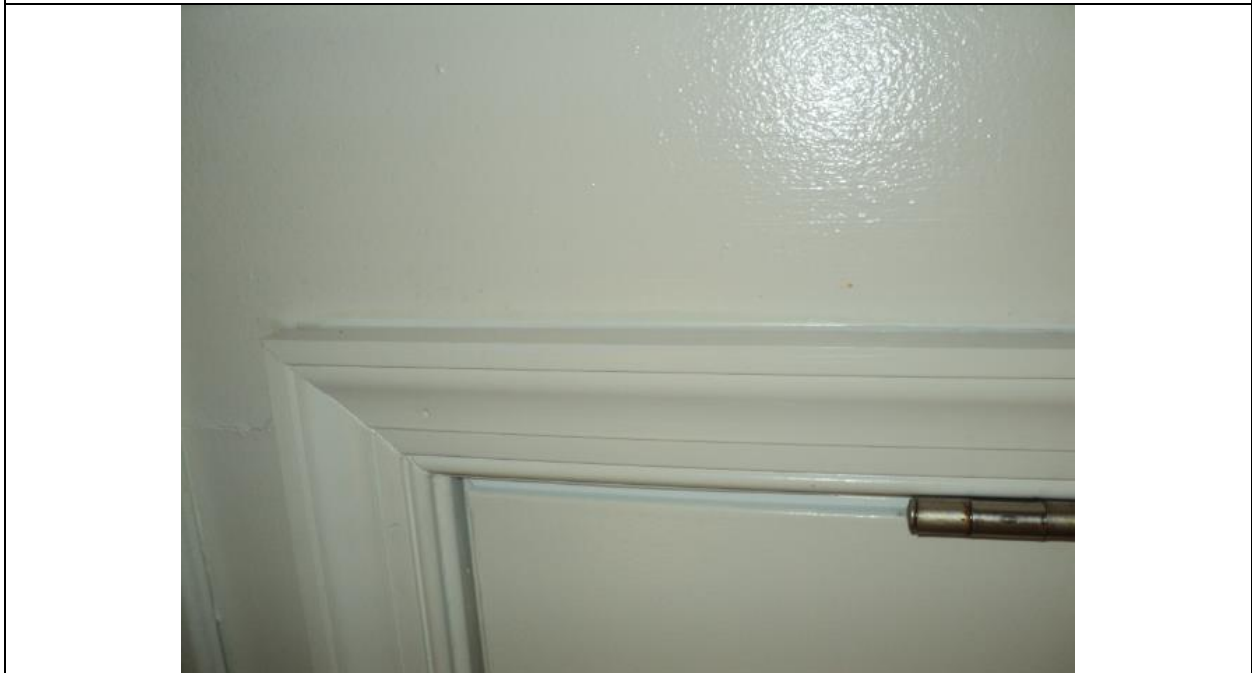
Homogeneous Material No. 4 – Non-ACM White Interior Door Caulk located in the Kitchen and Bedroom 1-3
