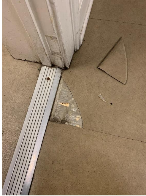
Homogeneous Material No. 1 – Non-ACM Tan 18” by 18” VFT with Cream Mastic located in the Kitchen and Laundry Area
