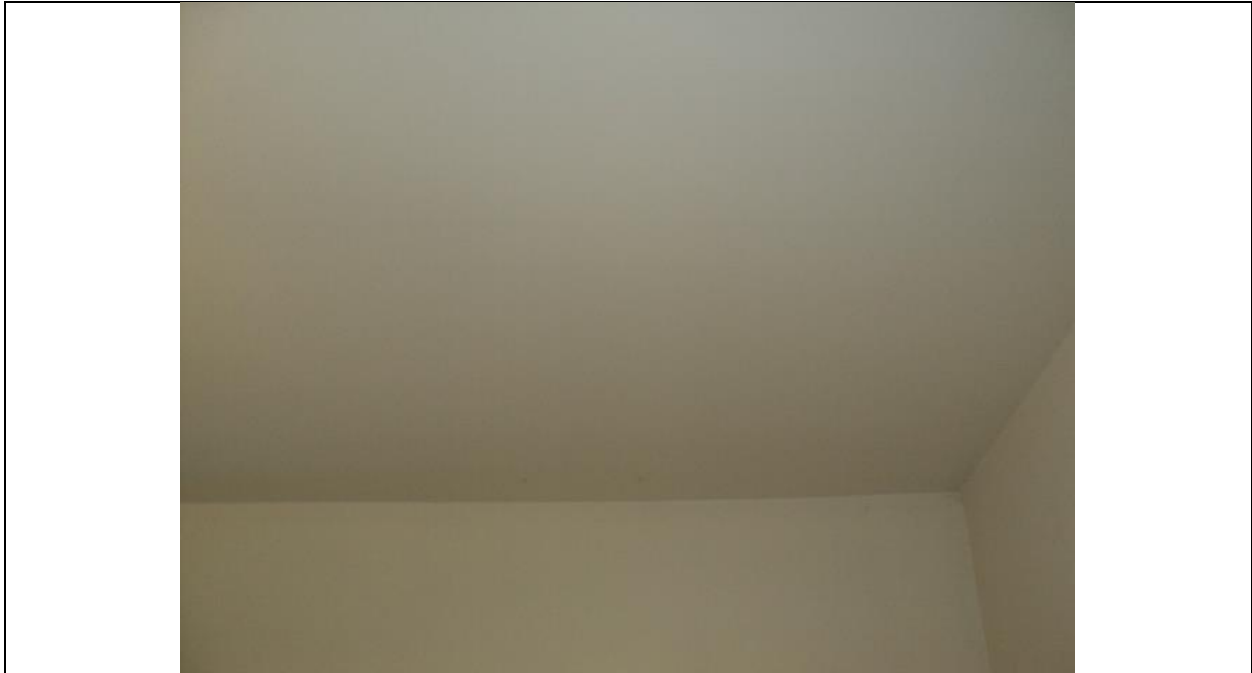
Homogeneous Material No. 3 – Non-ACM White Ceiling DW and Associated White JC located Throughout the Building including Dining Room, Bedroom 2-2 and Bedroom 3-2
