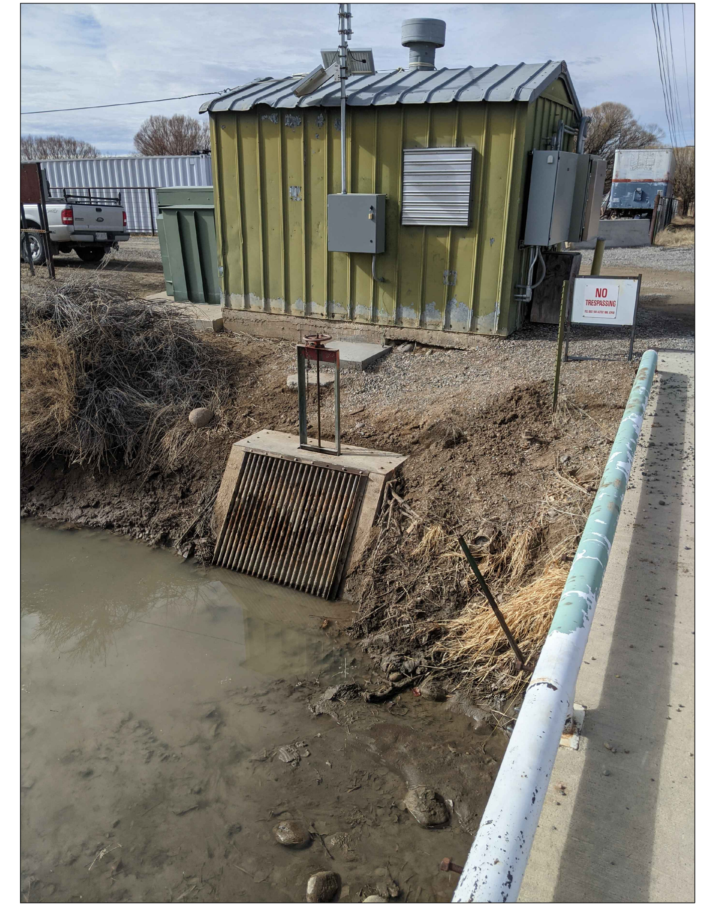
Pump House - Looking West
