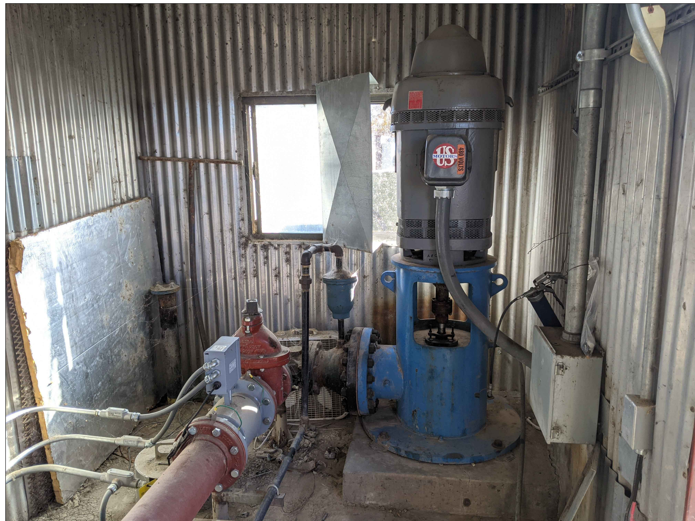
Pump House - Showing Existing Pump
