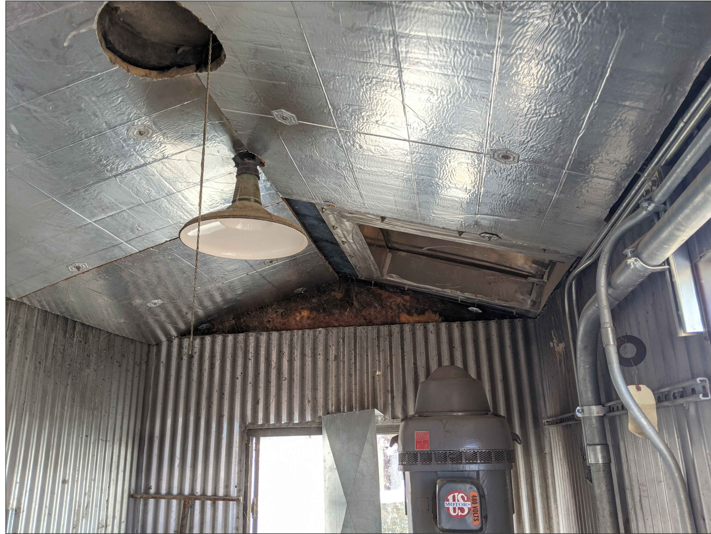
Pump House - Showing Roof Hatch
