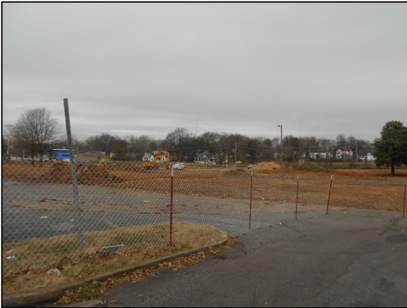
Five Points III, cleared site
