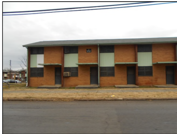
Existing building from Bethel Avenue.
