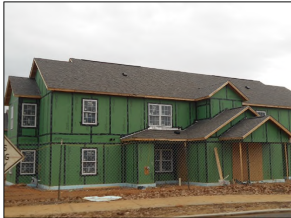
Five Points II, under construction west of site
