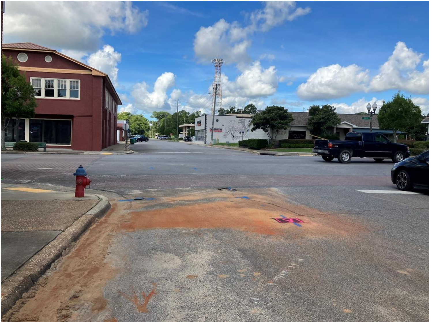
Figure 5C. Location A - Oakdale Ave side of Crestview Plumbing & Hardware - 297 Main St
