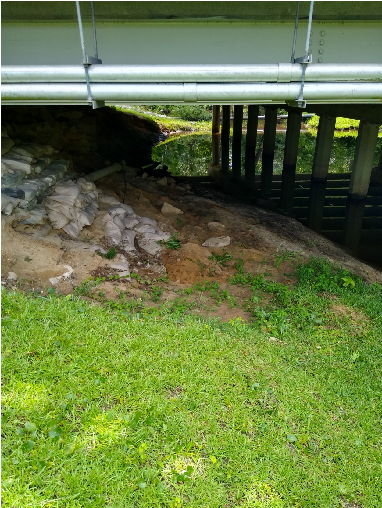
Figure 5 View of Hwy 70 Bridge and Slocum Creek from North side
