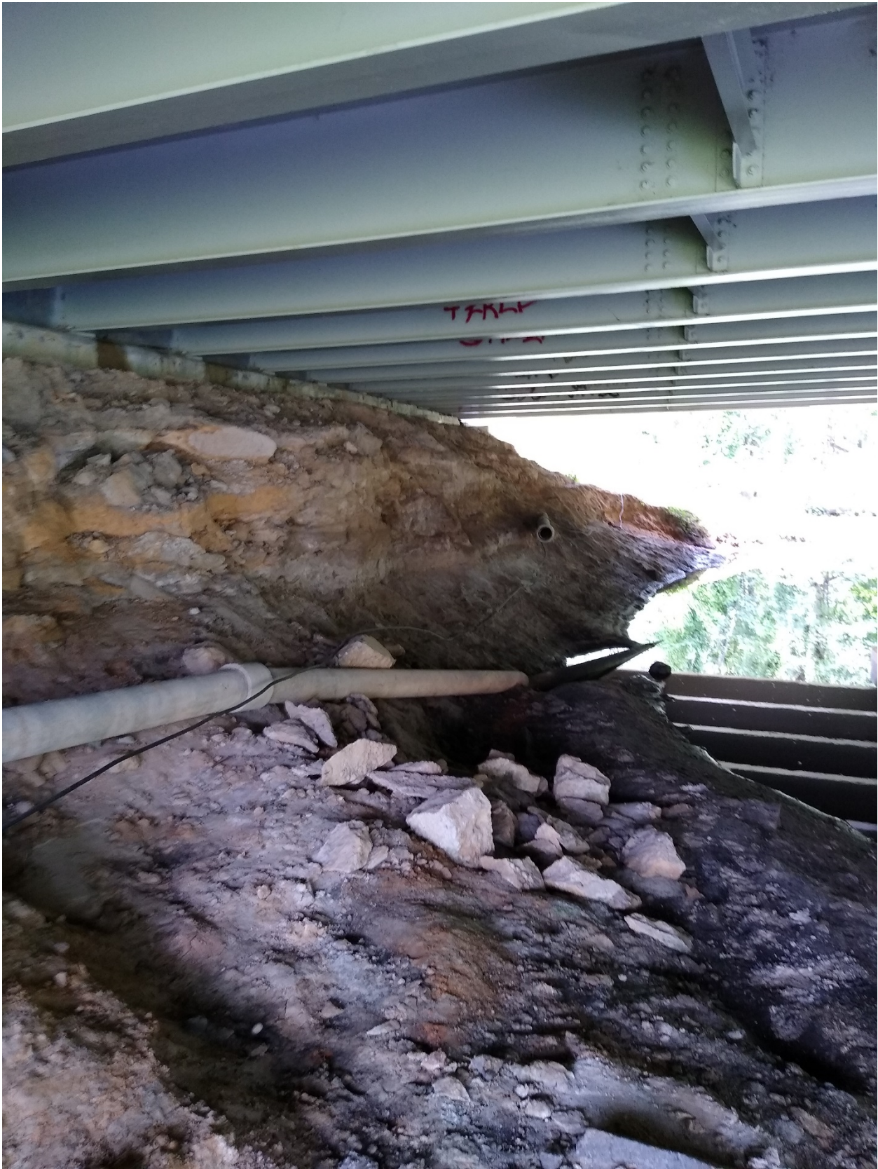
Figure 4 View of pipe and Slocum Creek from North side
