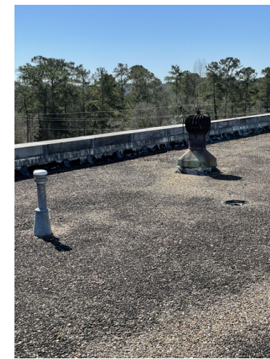
EXISTING ROOF DRAIN 3
