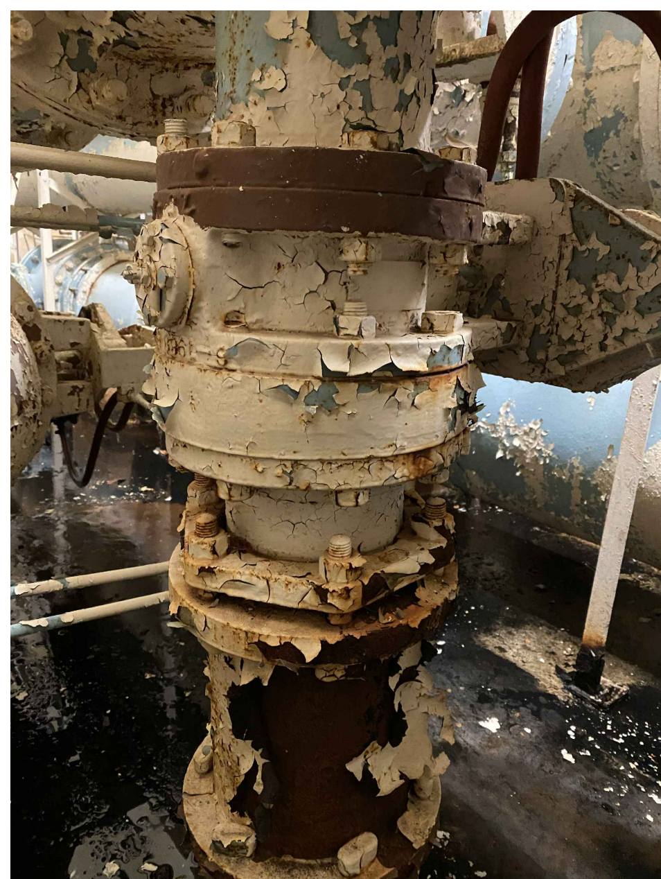
6" REWASH VALVE AND ACTUATOR
