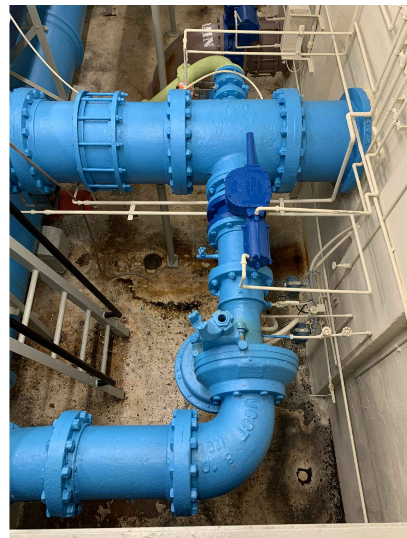
8" FILTERED VALVE, VENTURI & CONTROLLER
