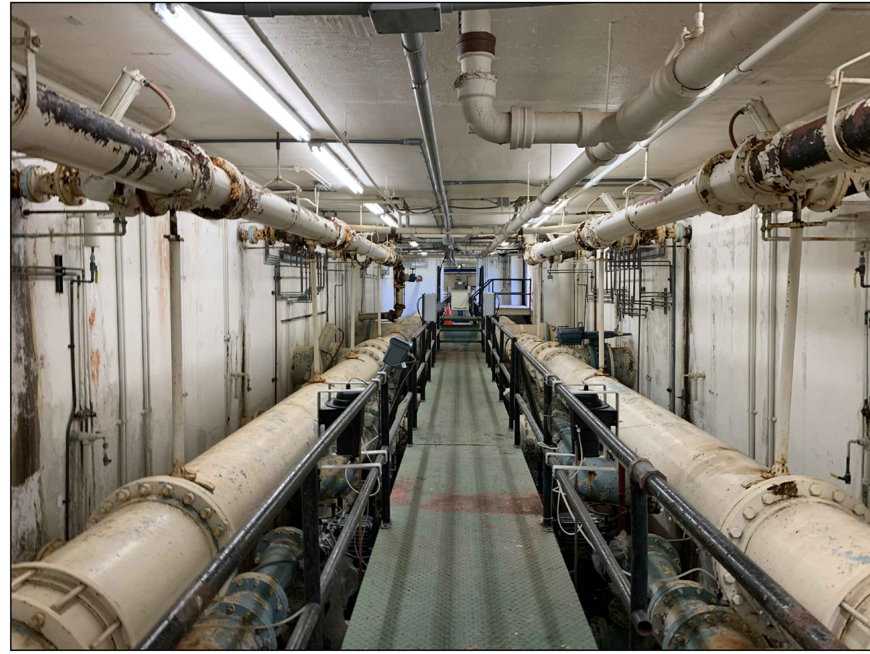
TURBIDITY METER CONTROLLER
