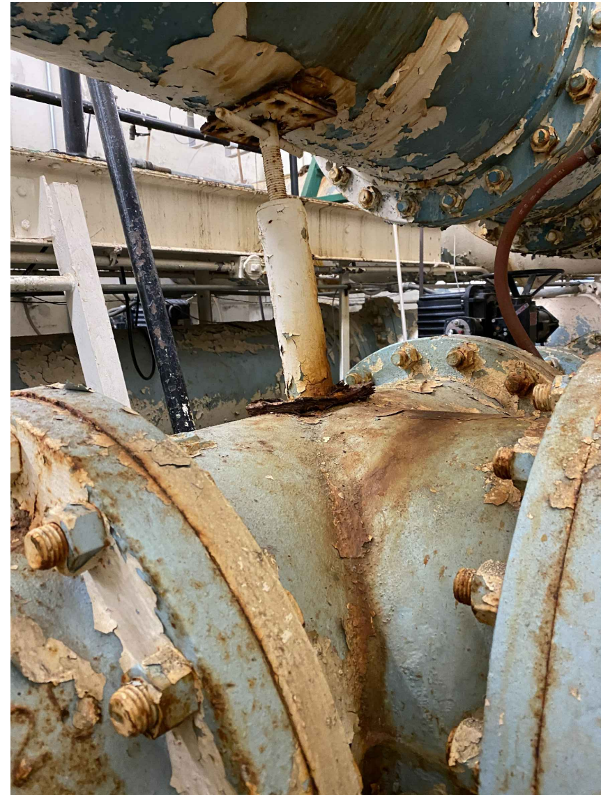
EXISTING PIPE SUPPORTS
