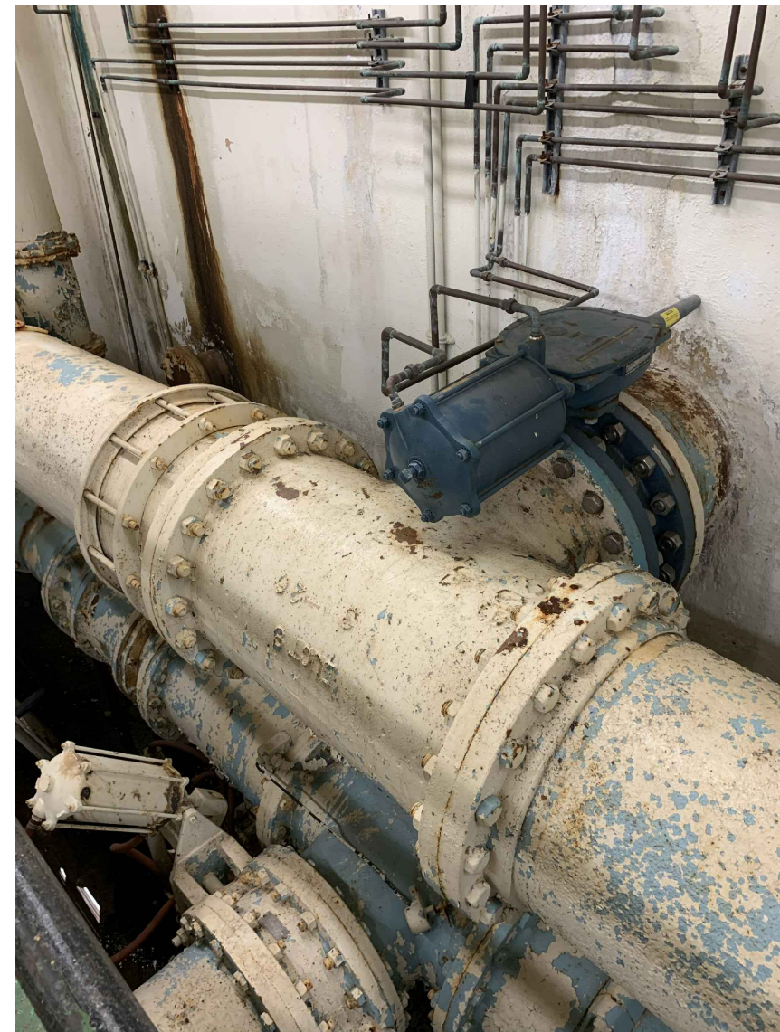
20" SETTLED VALVE & COUPLING
