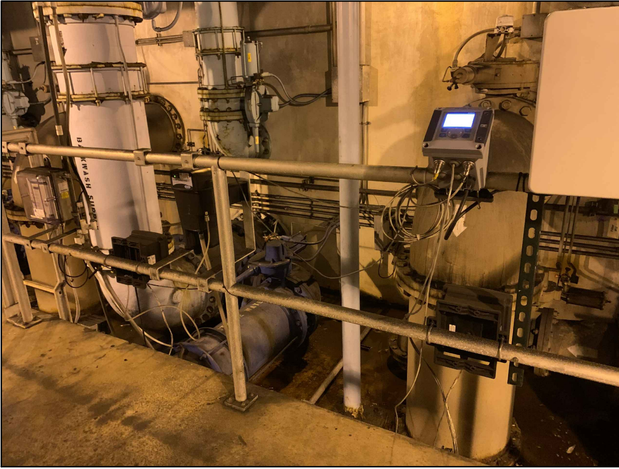
TURBIDITY SYSTEM & CONTROLLER
