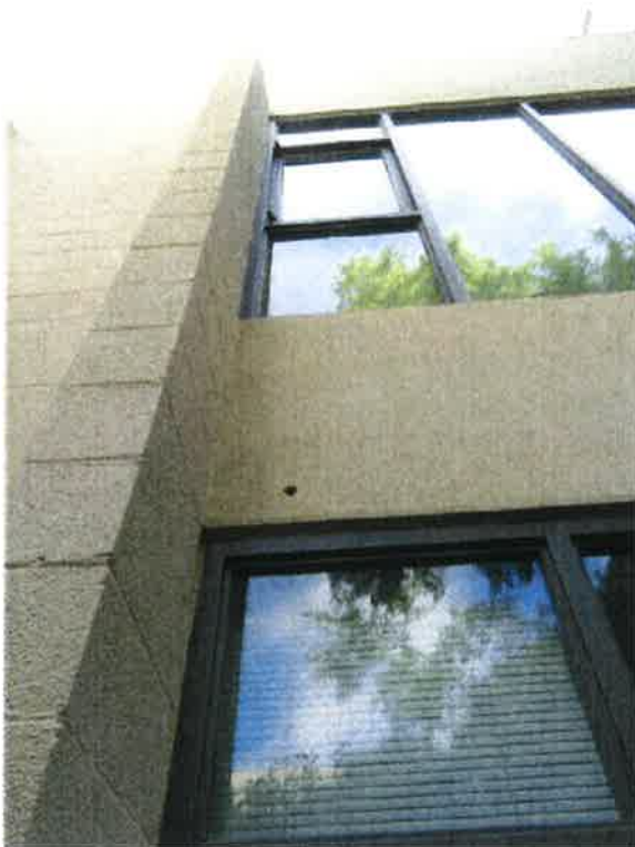
2118 Milvia Street – existing wire glass in steel frames at north elevation to be replaced
