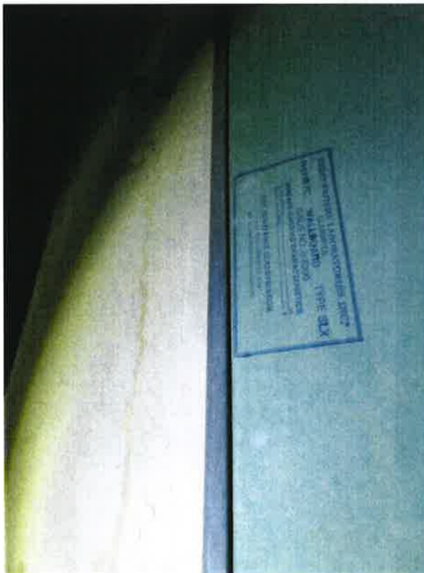
2118 Milvia Street – existing elevator shaft wall construction
