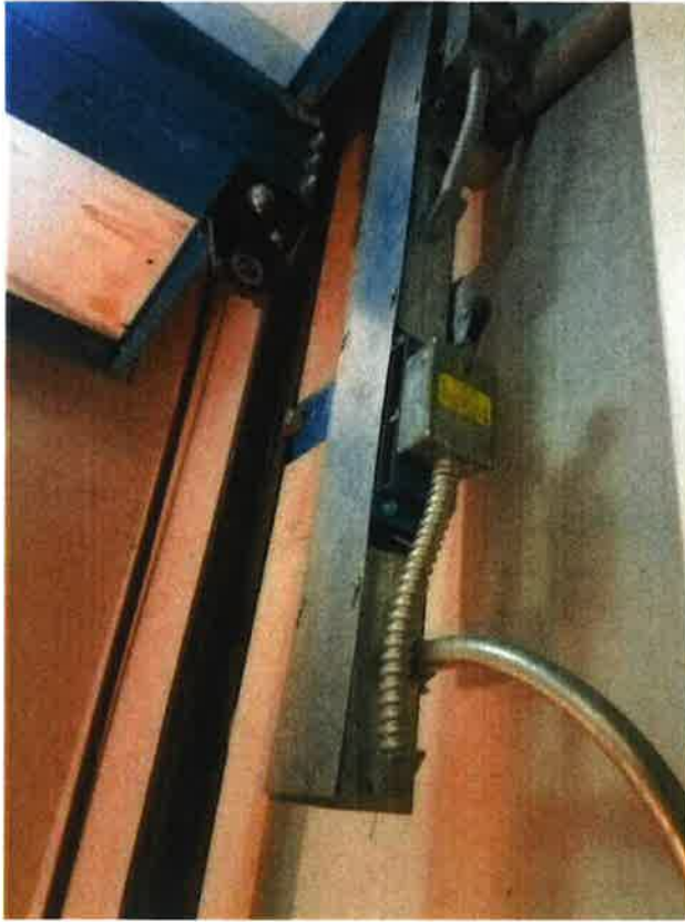
2118 Milvia Street – existing elevator guiderail attachment
