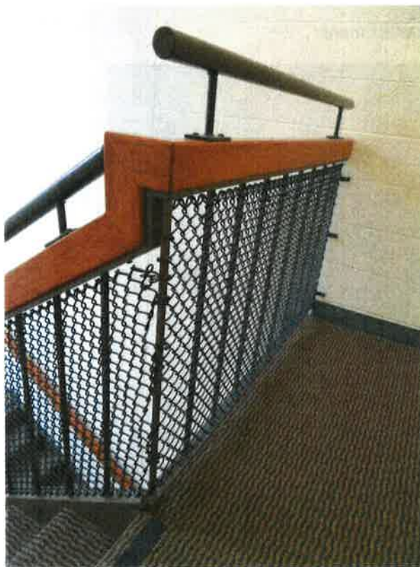
2118 Milvia Street – existing steel and concrete filled metal pan stair – guardrail to be replaced
