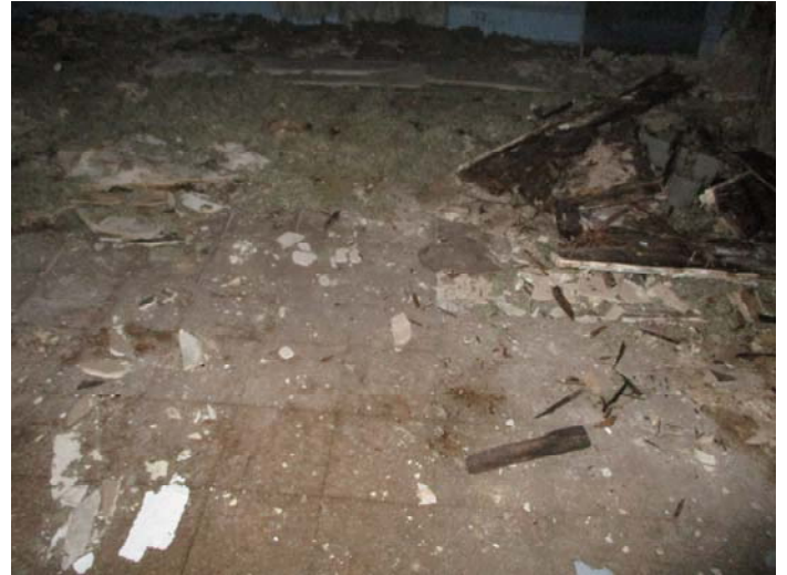
Photo 2 – 9"x9" brown streaked floor tile & mastic in the front left bedroom
