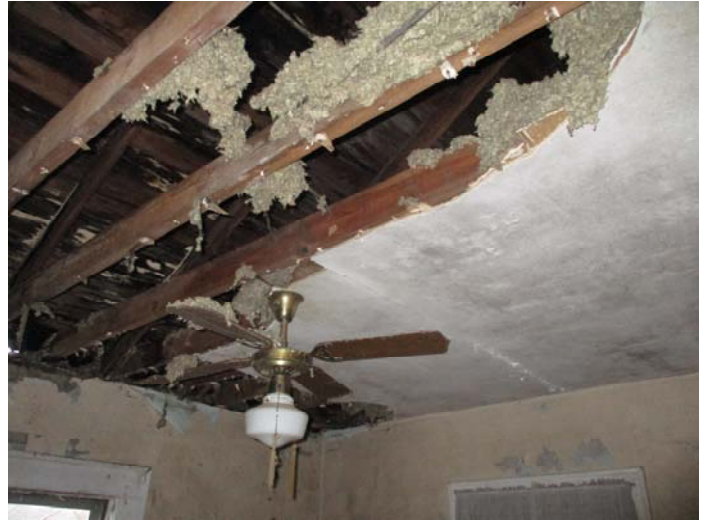
Photo 8 – Typical view of plaster with finish walls & ceilings throughout the residence
