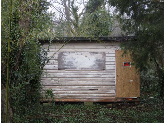
Photo 19 – Back shed with wooden construction & shingle and felt on the roof
