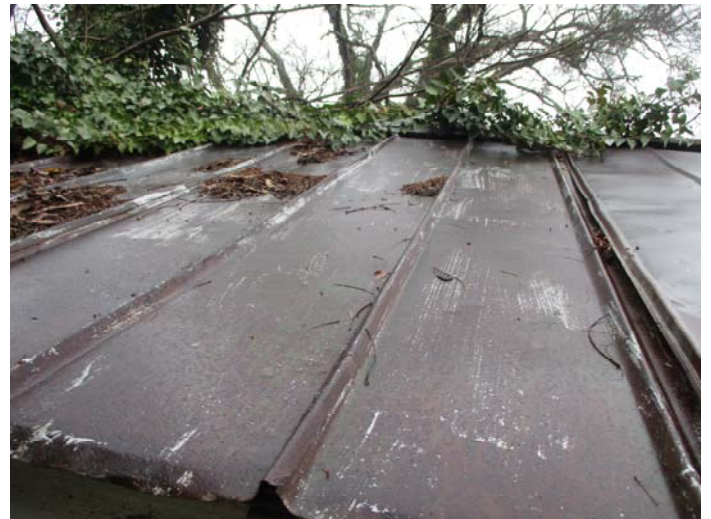
Photo 18 – Front shed with silver sealant on the metal roof
