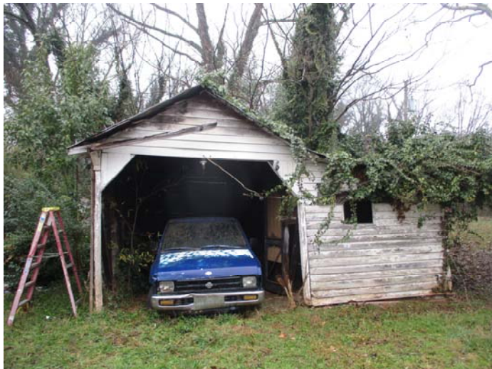
Photo 17 – Front shed with wooden construction & silver sealant on the metal roof
