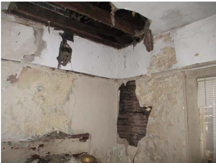
Photo 9 – Typical view of plaster with finish walls & ceilings throughout the residence
