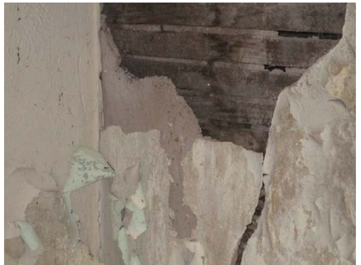
Photo 10 – Typical view of plaster with finish walls & ceilings throughout the residence
