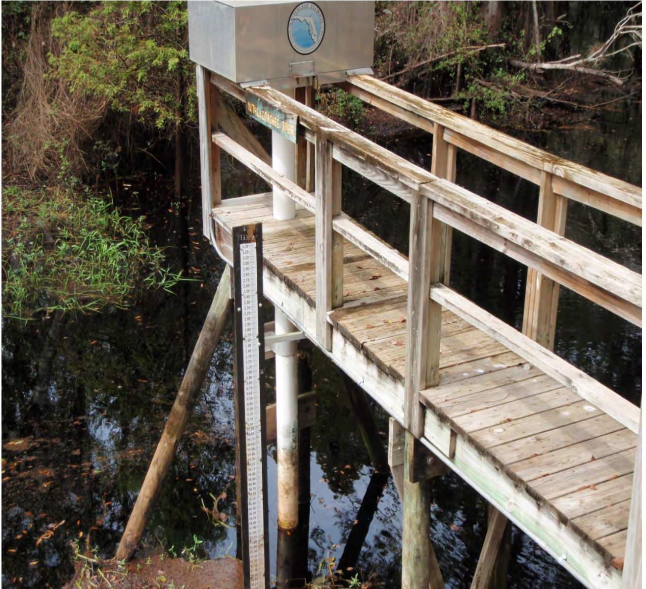
Figure 3: Stilling Well and Staff Gauge Facility
