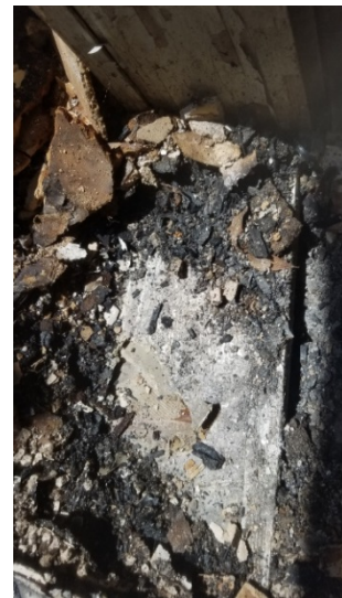
Photo 6 – Bathroom flooring in the addition.
