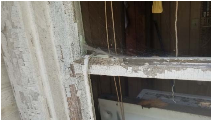
Photo 3 – Window caulk and glaze.
