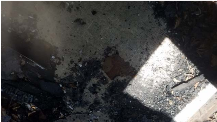
Photo 9 – Tan flooring at rear entrance.
