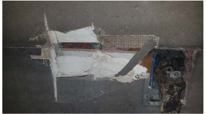
Photo 2 – Drywall, joint compound and tape.
