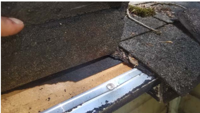
Photo 5 – Roof shingle and felt.
