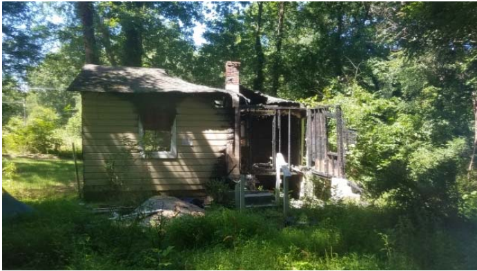
Photo 1 – 112 Owens Street in Spartanburg, South Carolina.
