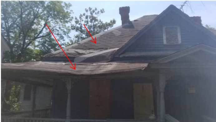
Photo 9 – Main and porch roofs.
