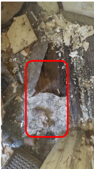
Photo 5 – Back porch grey flooring.
