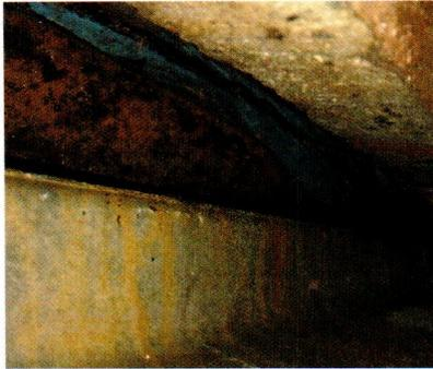
*Figure 1: Soil infiltration due to leaked joint*
