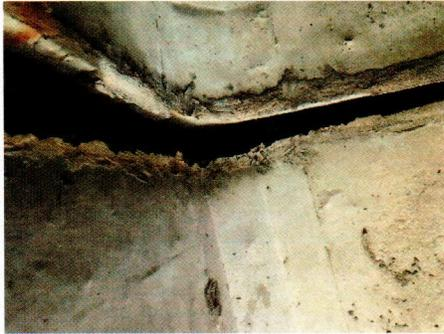
*Figure 4: Separated joint*
