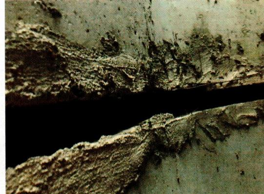
*Figure 5: 5 1/2\" separation of joint*
