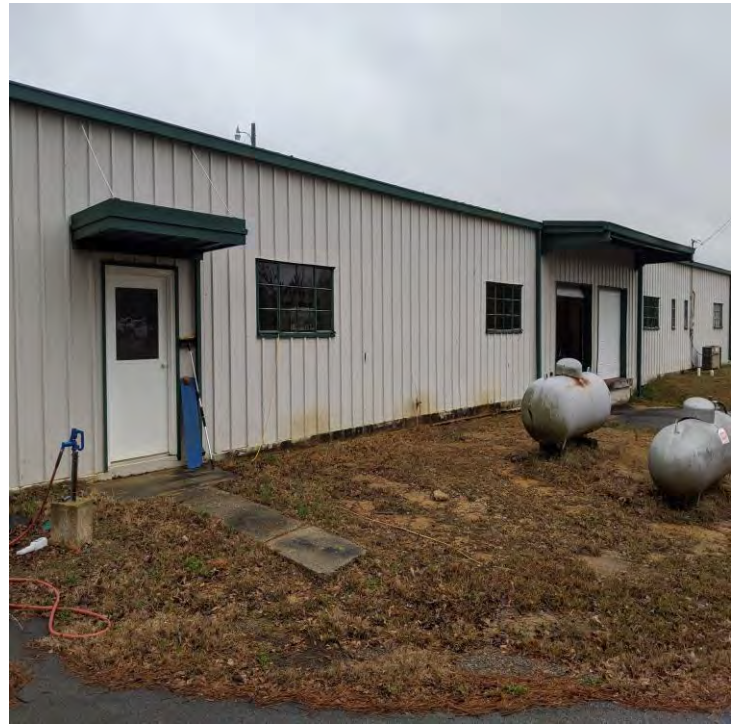
West Face of Structure
