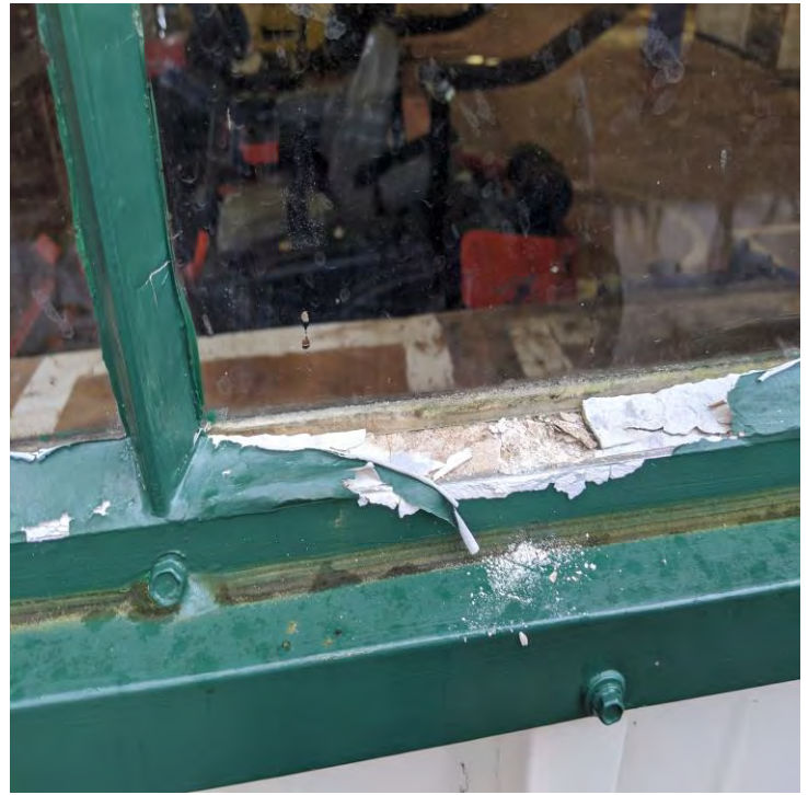
West Warehouse Window Glazing Sample # 22
