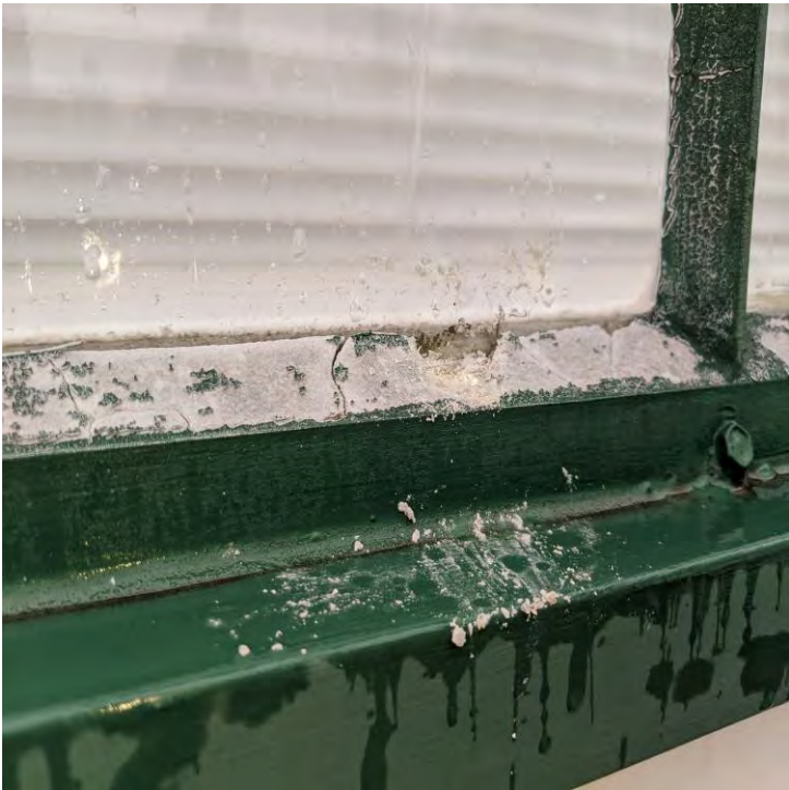
South Office Window Glazing Sample # 21
