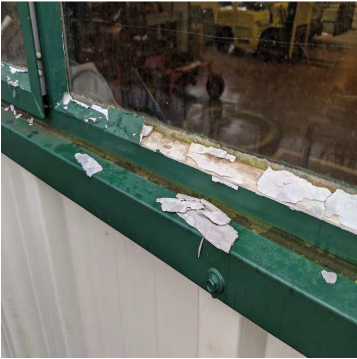
North Warehouse Window Glazing Sample # 19
