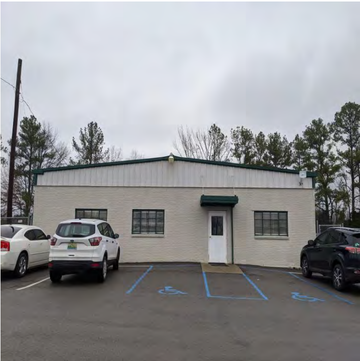
South Face of Structure
