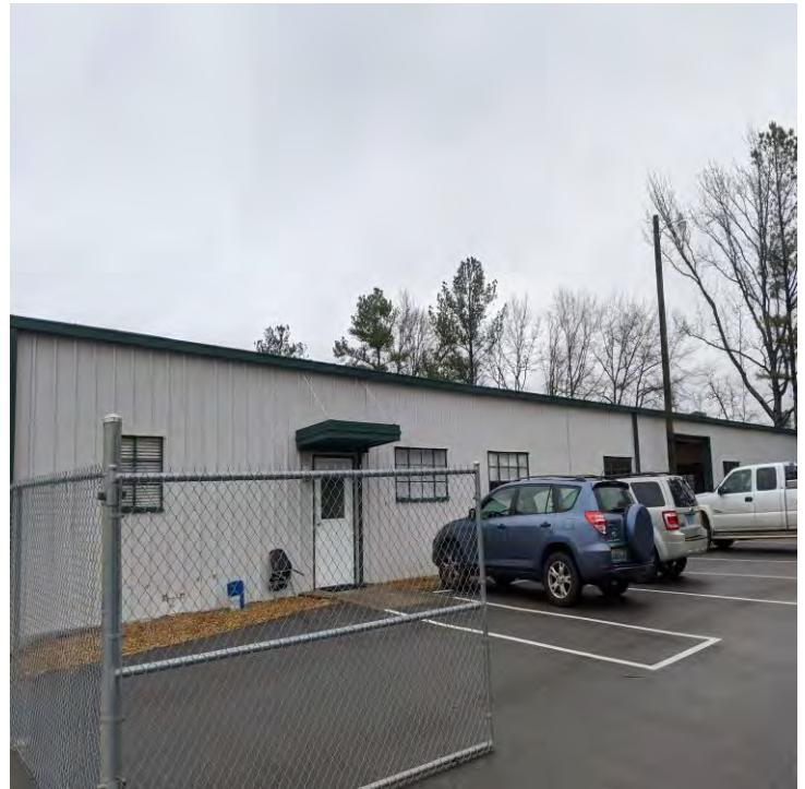
East Face of Structure
