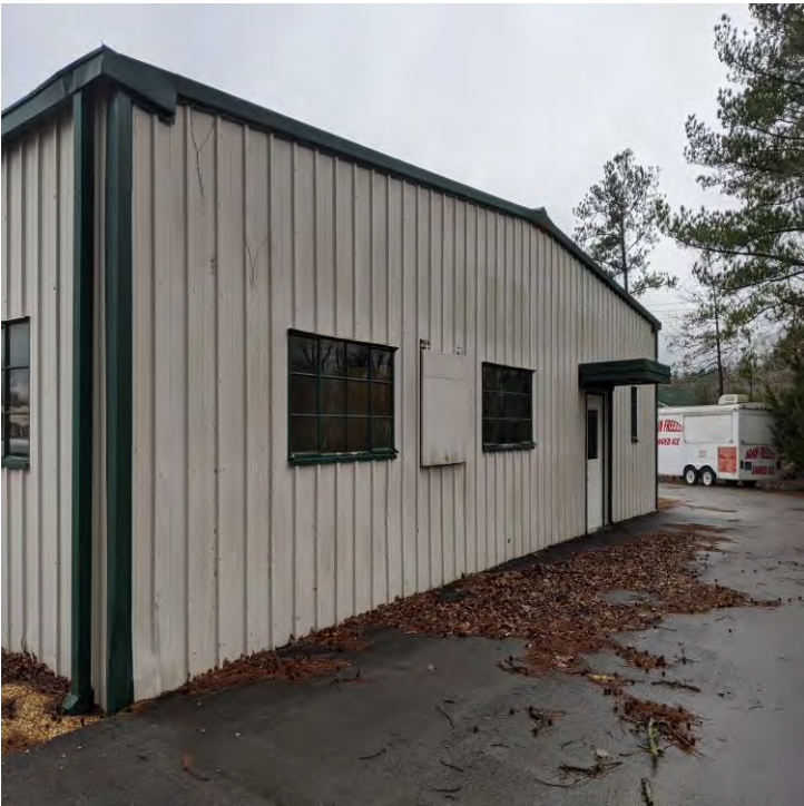
North Face of Structure
