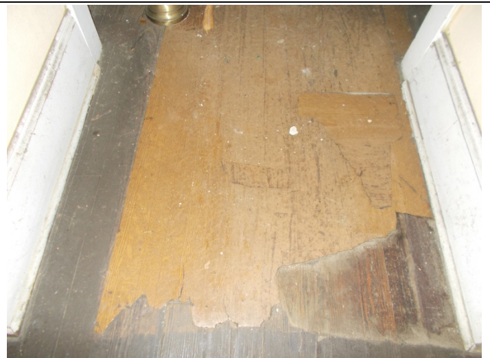
Photo 12 – Brown wooden plank pattern vinyl floor with no mastic in the hallway
