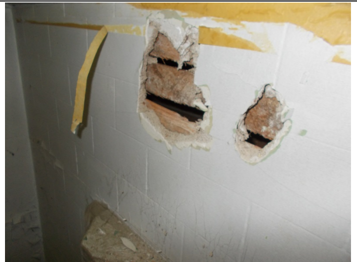
Photo 8 – Brick pattern plaster with finish in the bathroom lower 1/2 of walls
