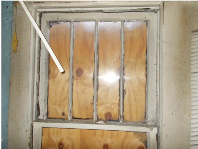
Photo 7 – Wooden window glazing
