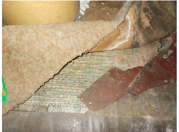
Photo 14 – Tan & blue pattern vinyl floor with no mastic in the back left bedroom under carpet
