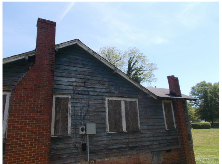
Photo 4 – 3 chimneys with mastic/tar & caulk on the right side of house
