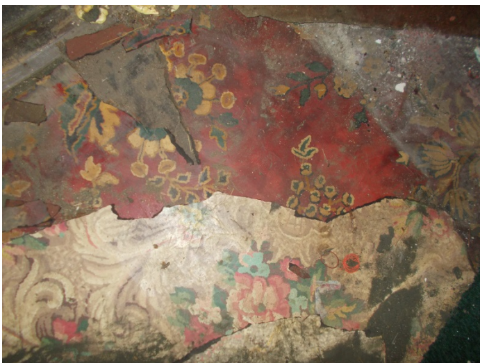
Photo 17 – Pink flower pattern vinyl floor over red & black plant pattern vinyl floor (no mastics) in the Front left bedroom (2nd & 3rd layers)
