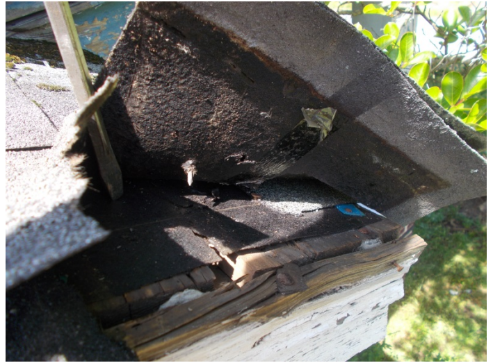
Photo 2 – Roof shingles and felt
