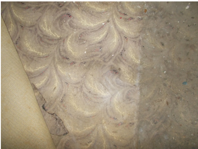
Photo 15 – Green & yellow pattern vinyl floor with no mastic in the back right bedroom & front right living room (top layers)
