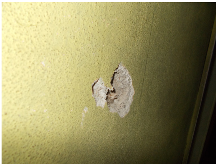
Photo 9 – Plaster with finish throughout
