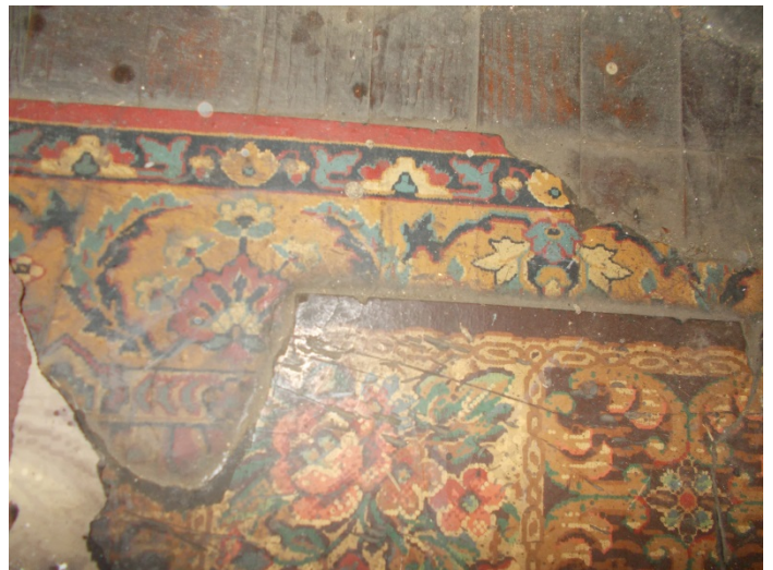
Photo 16 – Rose pattern vinyl floor over floral pattern vinyl floor (no mastics) in the back right bedroom (2nd & 3rd layers)
