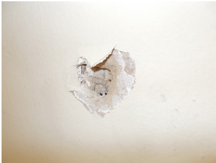
Photo 7 – Plaster with finish throughout
