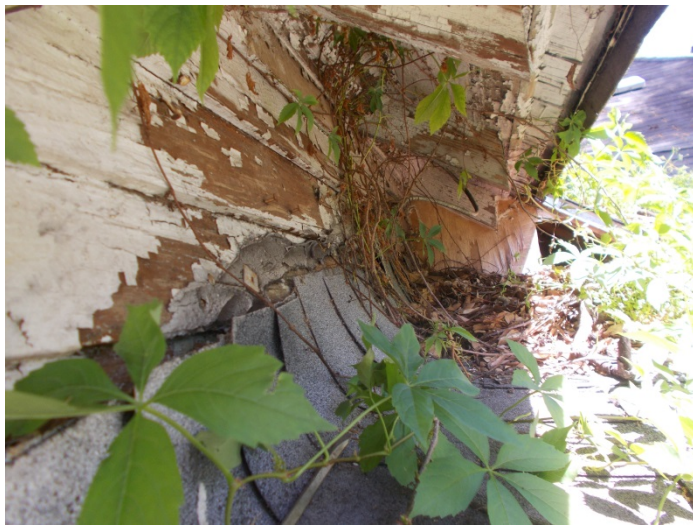
Photo 3 – Roof flashing with mastic/tar
