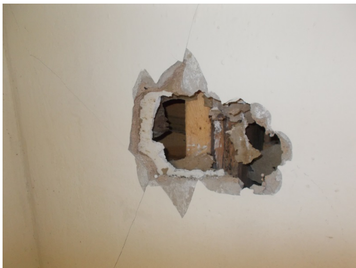
Photo 11 – Plaster over drywall
