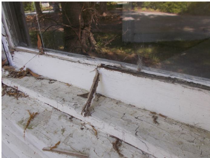
Photo 5 – Wooden window caulk
