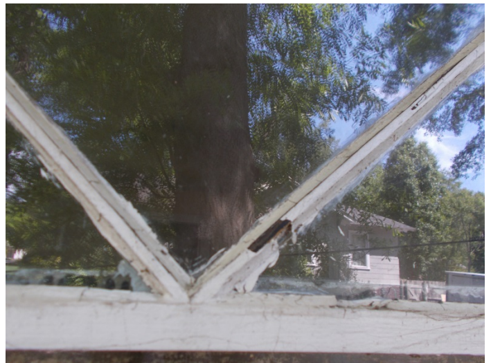
Photo 4 – Wooden window glazing
