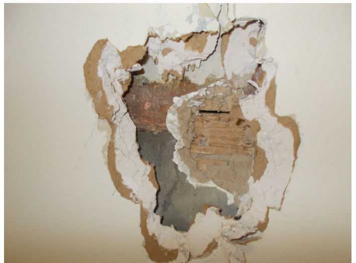
Photo 10 – Drywall over plaster
