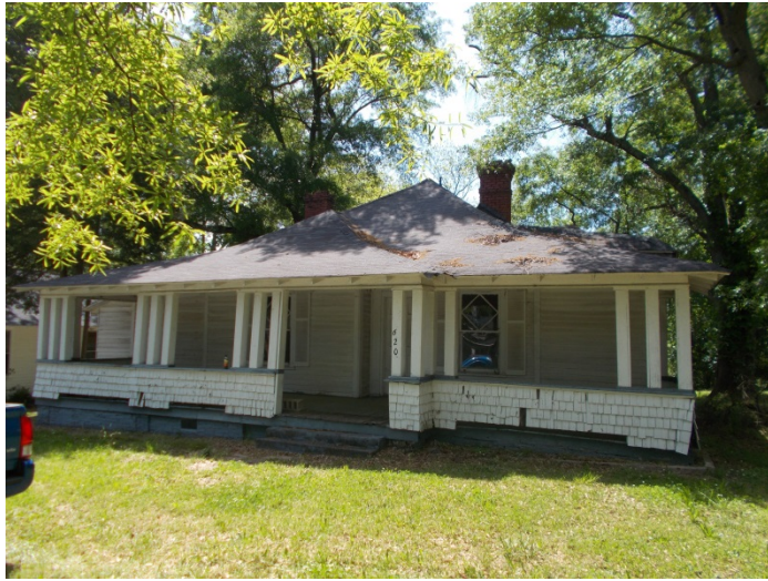
Photo 1 – 620 South Irwin Avenue in Spartanburg, South Carolina
