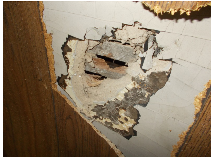
Photo 14 – Wall material with felt over plaster in the kitchen
