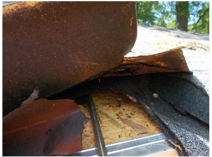
Photo 2 – Roof shingles and felt
