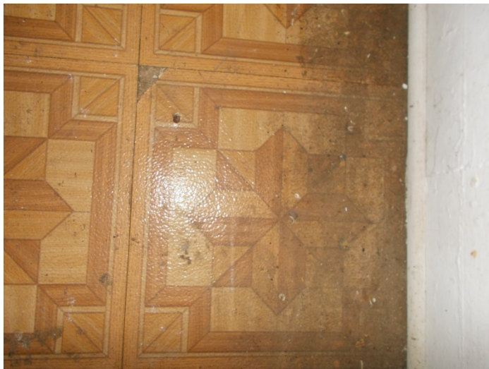
Photo 17 – 12" x 12" wooden pattern self-stick floor tile & mastic in the Kitchen (2nd layer); back entry (2nd layer) & back entry hallway
