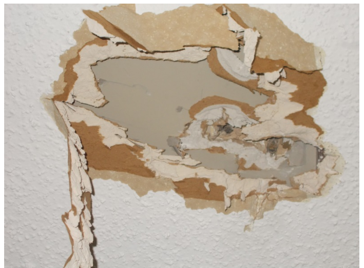
Photo 12 – Drywall over plaster
