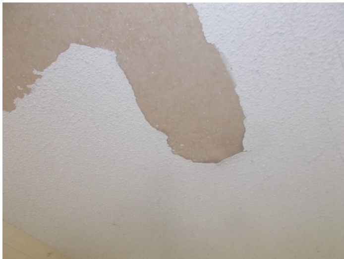
Photo 9 – Popcorn ceiling texture in the front left room, living room, dining room, kitchen, front bathroom & back-middle left bedroom
