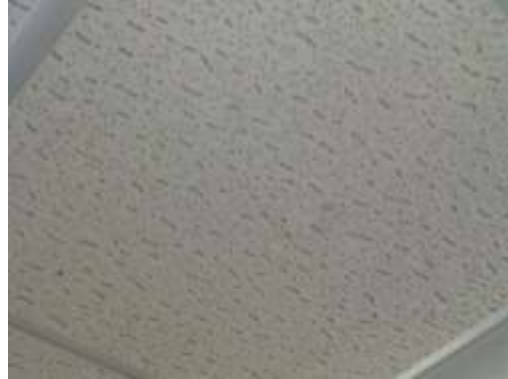
HOMOGENEOUS AREA 10 2' X 2' CEILING TILE
