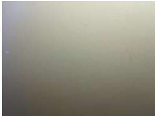
HOMOGENEOUS AREA 04, 04A PLASTER/SKIM COAT
