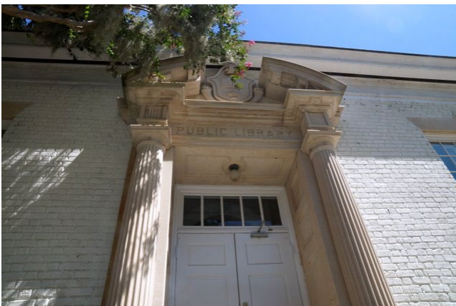
Exterior lighting at front door
