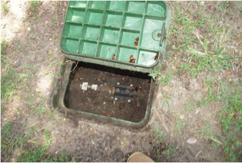
Water service to building
