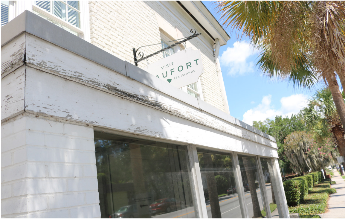
Figure 32: Beaufort Carnegie Library Building, East Elevation. Overview of addition and cornice.
