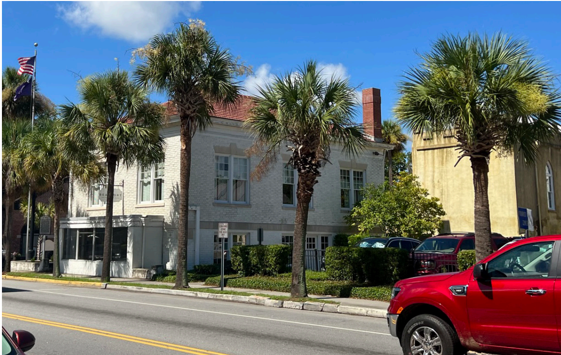
Figure 26: Beaufort Carnegie Library Building, Northeast Corner: The masonry is in fair condition on the back elevation.
