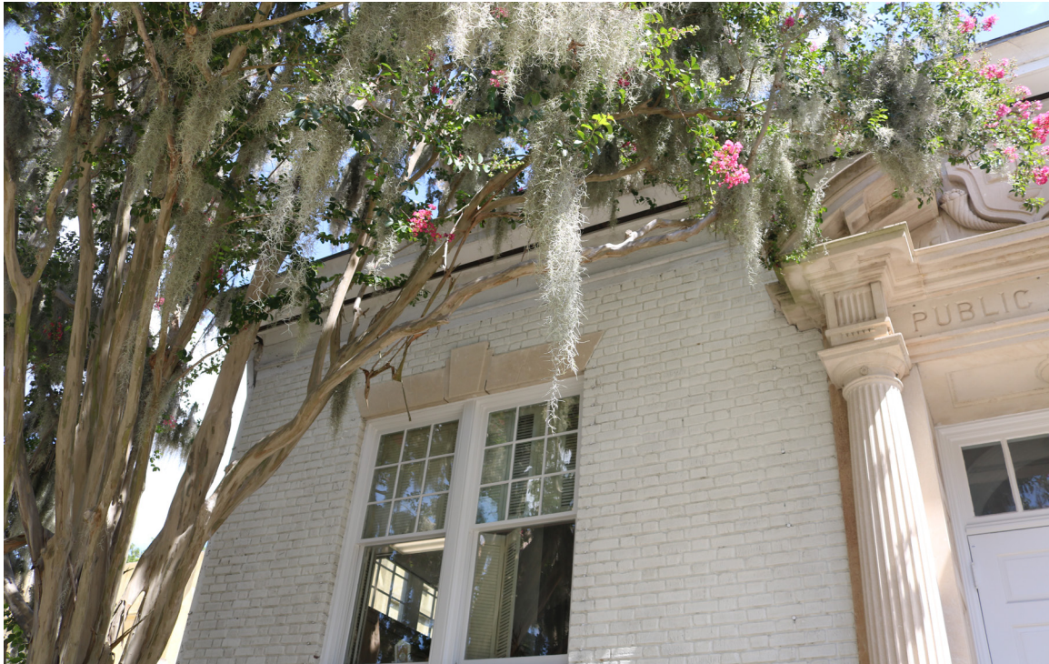
Figure 21: Beaufort Carnegie Library Building, South Elevation, West Side: The branches of the crepe myrtle are in direct contact with the masonry and the roof. The tree should be sensitively trimmed away from the historic building.
