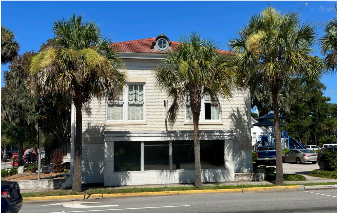
Figure 30: Beaufort Carnegie Library Building, East Elevation and East Entrance.
