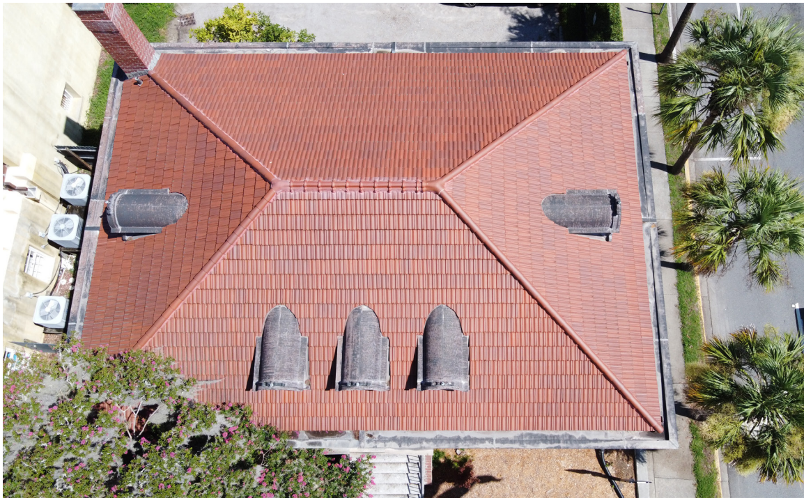
Figure 34: Beaufort Carnegie Library Building, Overview of the Ludowici French tile roof.
