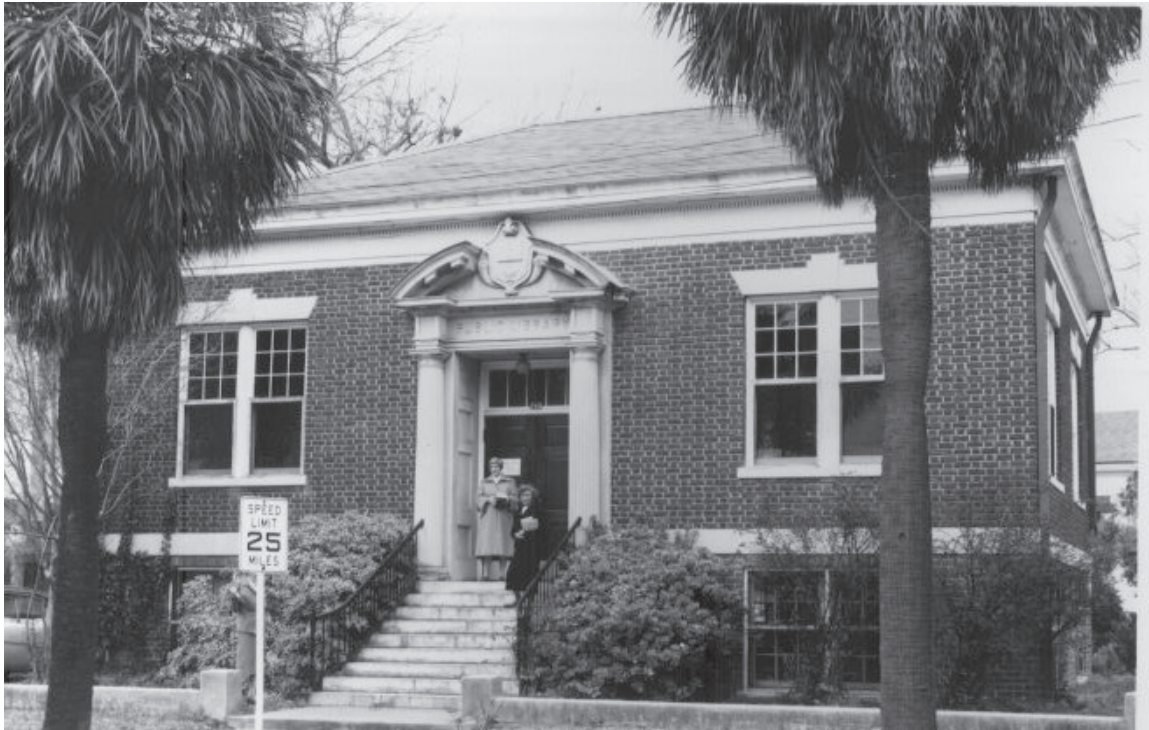
Figure 12: Post 1964 photo of the building after the removal of the tile roof and ocular dormers.
