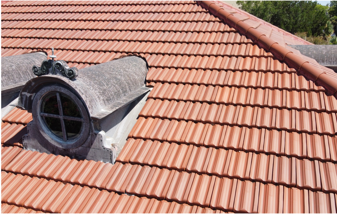
Figure 36: Beaufort Carnegie Library Building, South Elevation Dormers: East Side.
