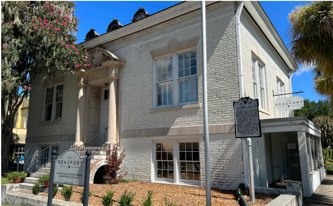
Figure 14: Beaufort Carnegie Library Building, South Elevation: Overview of the painted masonry.
