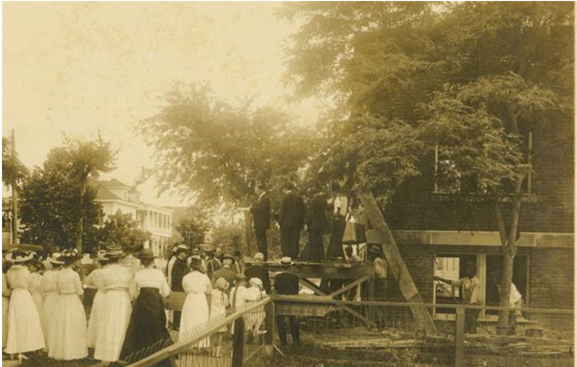
Figure 6: June 1917 construction photograph. The image captures the north side of the building looking south.
