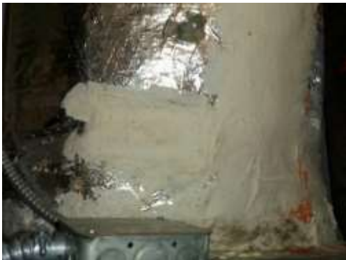
HOMOGENEOUS AREA 03 HVAC DUCT MASTIC (WHITE)
