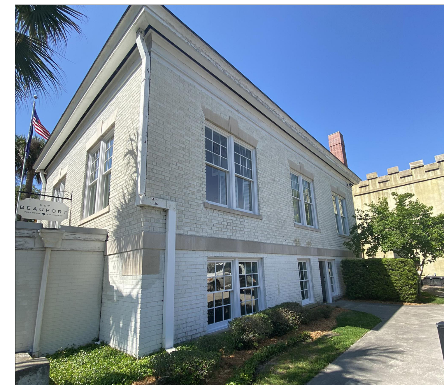
EXISTING CONDITIONS- NORTHEAST ELEVATION
