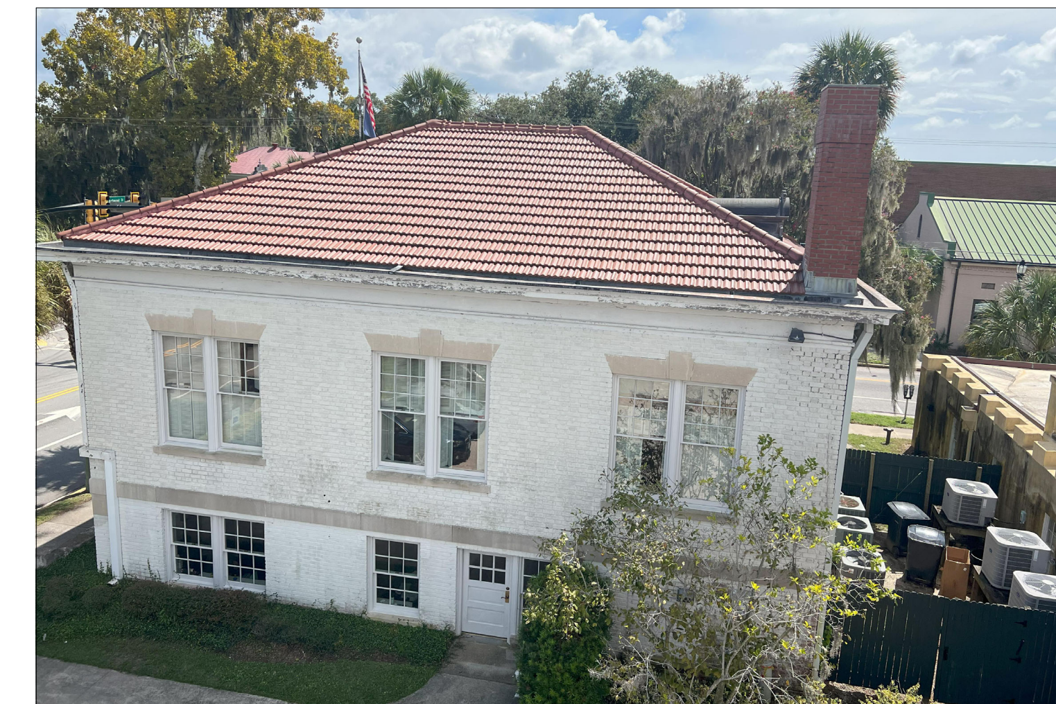
EXISTING CONDITIONS- NORTH ELEVATION & ROOF
