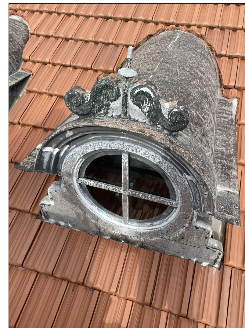
EXISTING CONDITIONS- DETAILED VIEW OF DORMER FRONT AT SOUTH ELEVATION.
