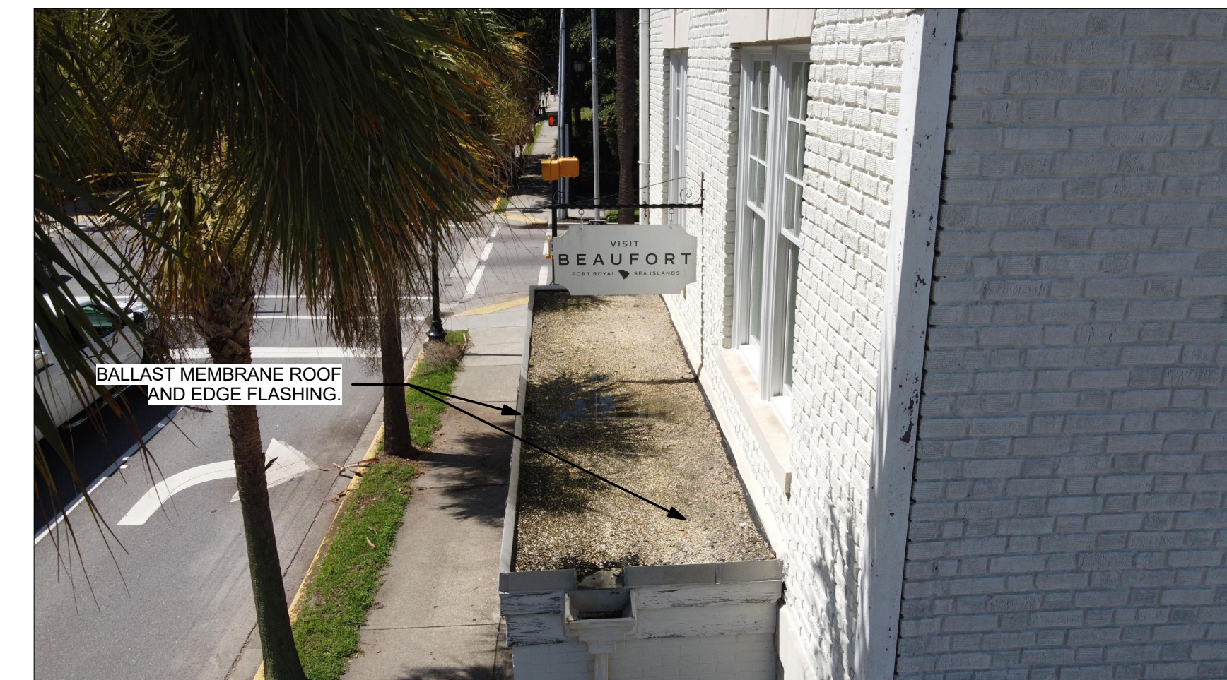
EXISTING CONDITIONS- EAST ELEVATION ADDITION ROOF.
