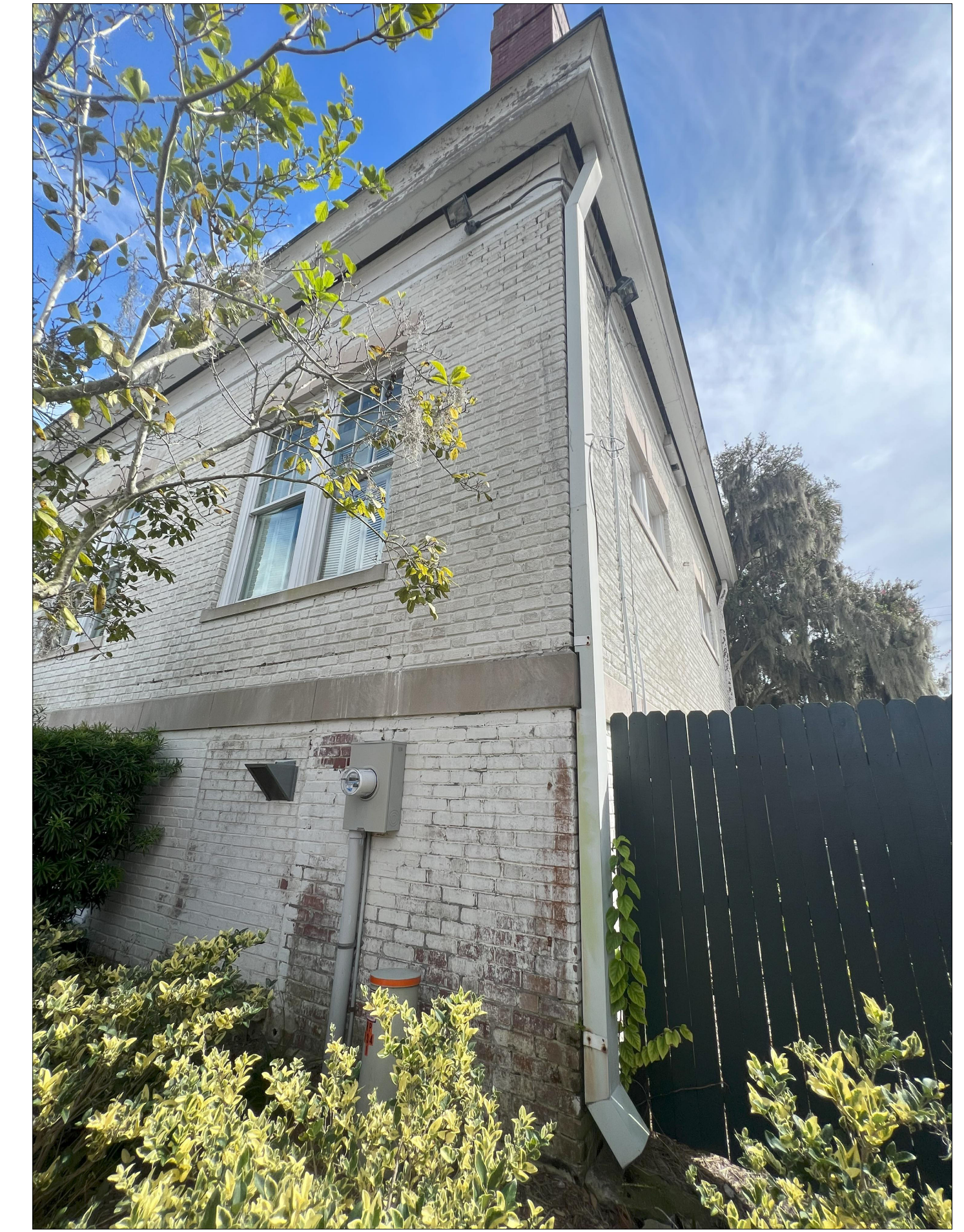
EXISTING CONDITIONS- NORTHWEST CORNER DOWNSPOUT.
