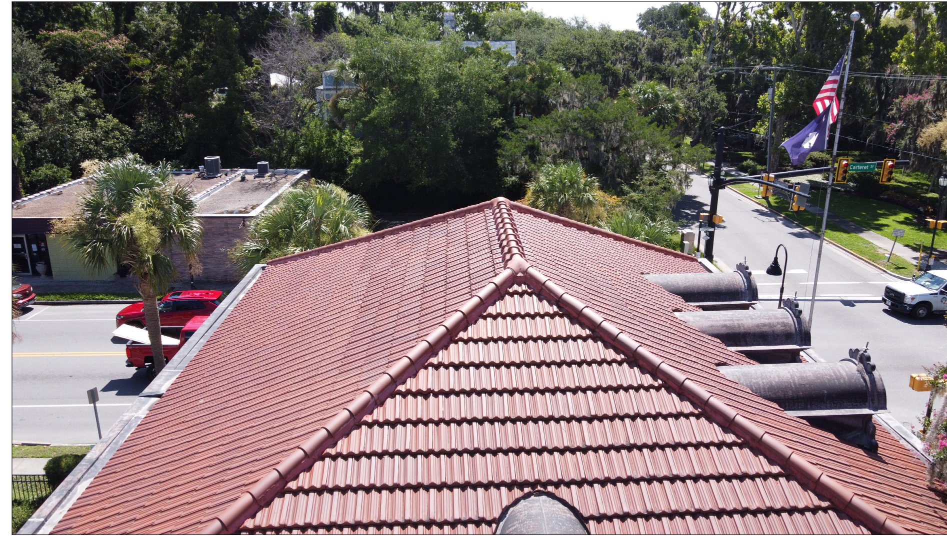
EXISTING CONDITIONS- VIEW OF ROOF LOOKING EAST.
