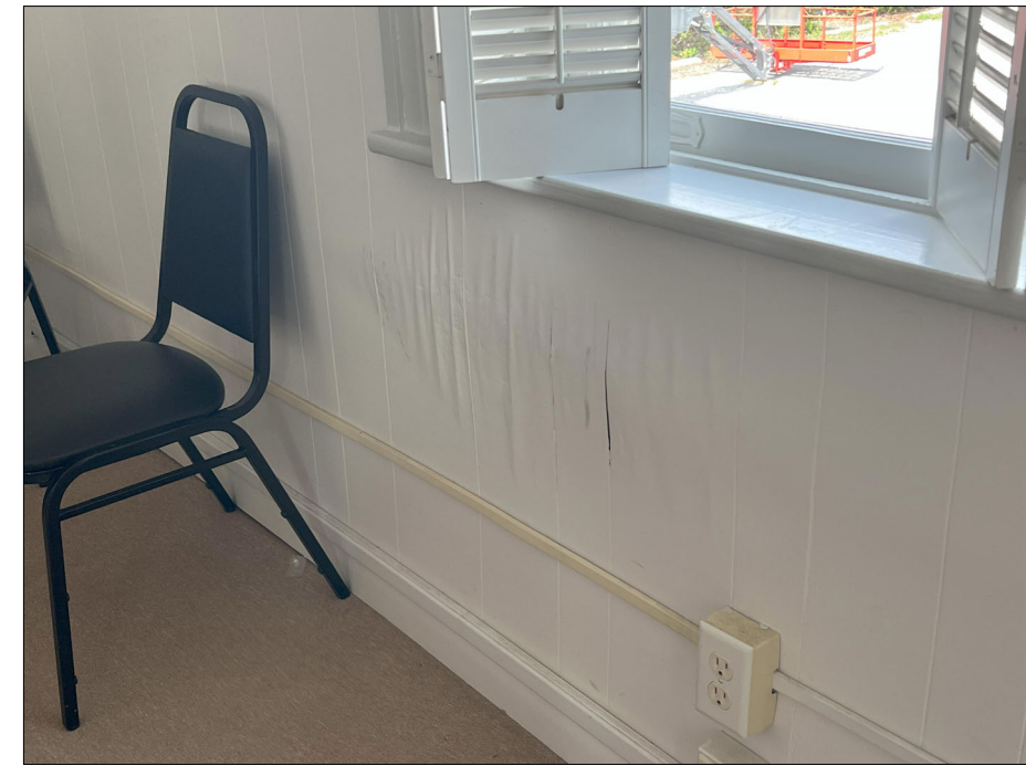
DETAIL PHOTO OF WATER DAMAGE BELOW WINDOWS 20 & 21.
