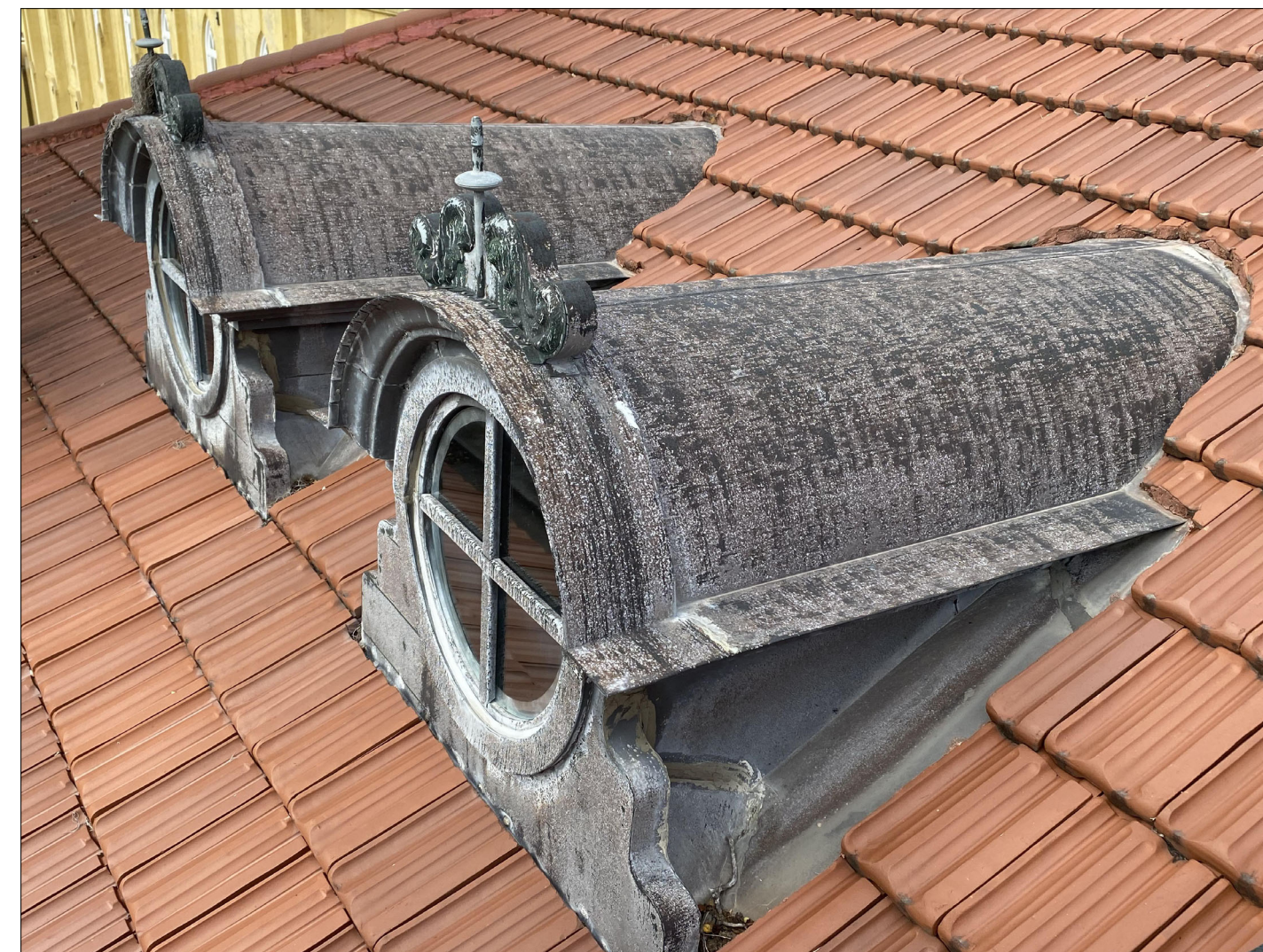
EXISTING CONDITIONS- DETAILED VIEW OF SOUTH ELEVATION DORMERS FROM THE SIDE.
