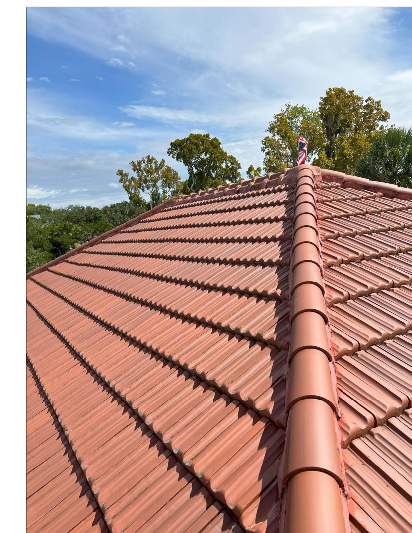
EXISTING CONDITIONS- DETAILED VIEW OF RIDGE TILES.
