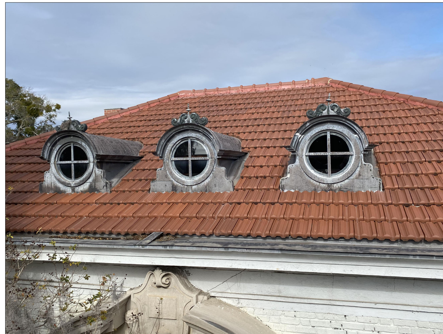
EXISTING CONDITIONS- VIEW OF SOUTH ELEVATION DORMERS.
