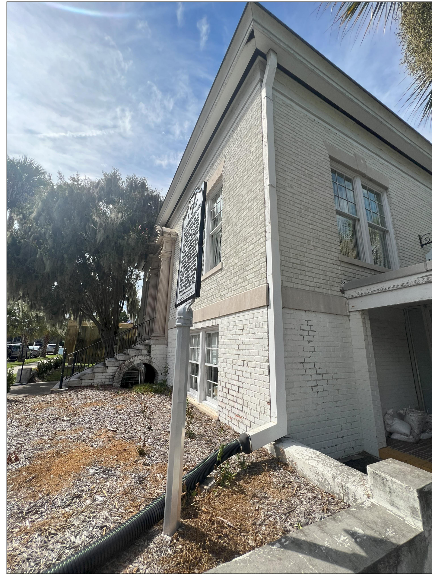
EXISTING CONDITIONS- SOUTHEAST CORNER DOWNSPOUT.
