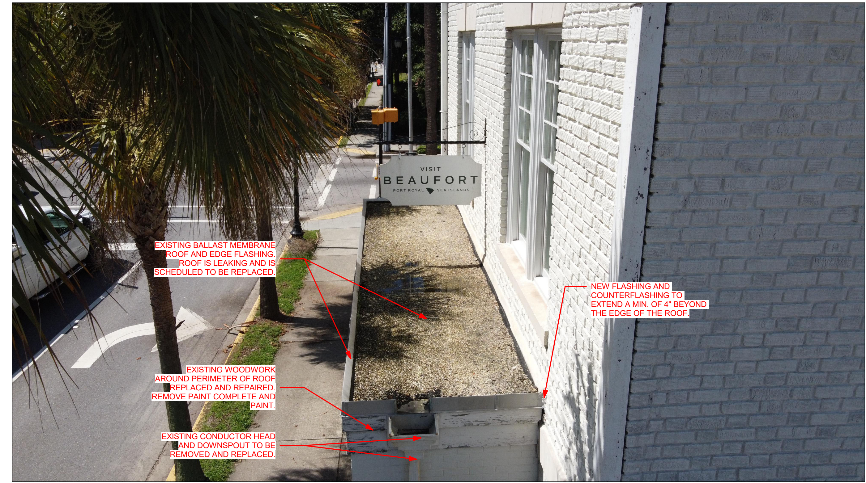
EXISTING CONDITIONS- EAST ELEVATION ADDITION ROOF
