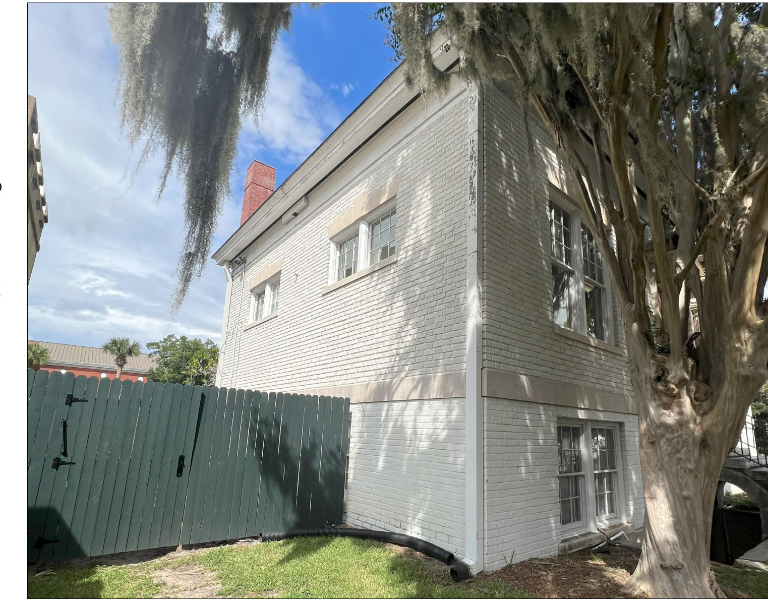
EXISTING CONDITIONS- WEST ELEVATION
