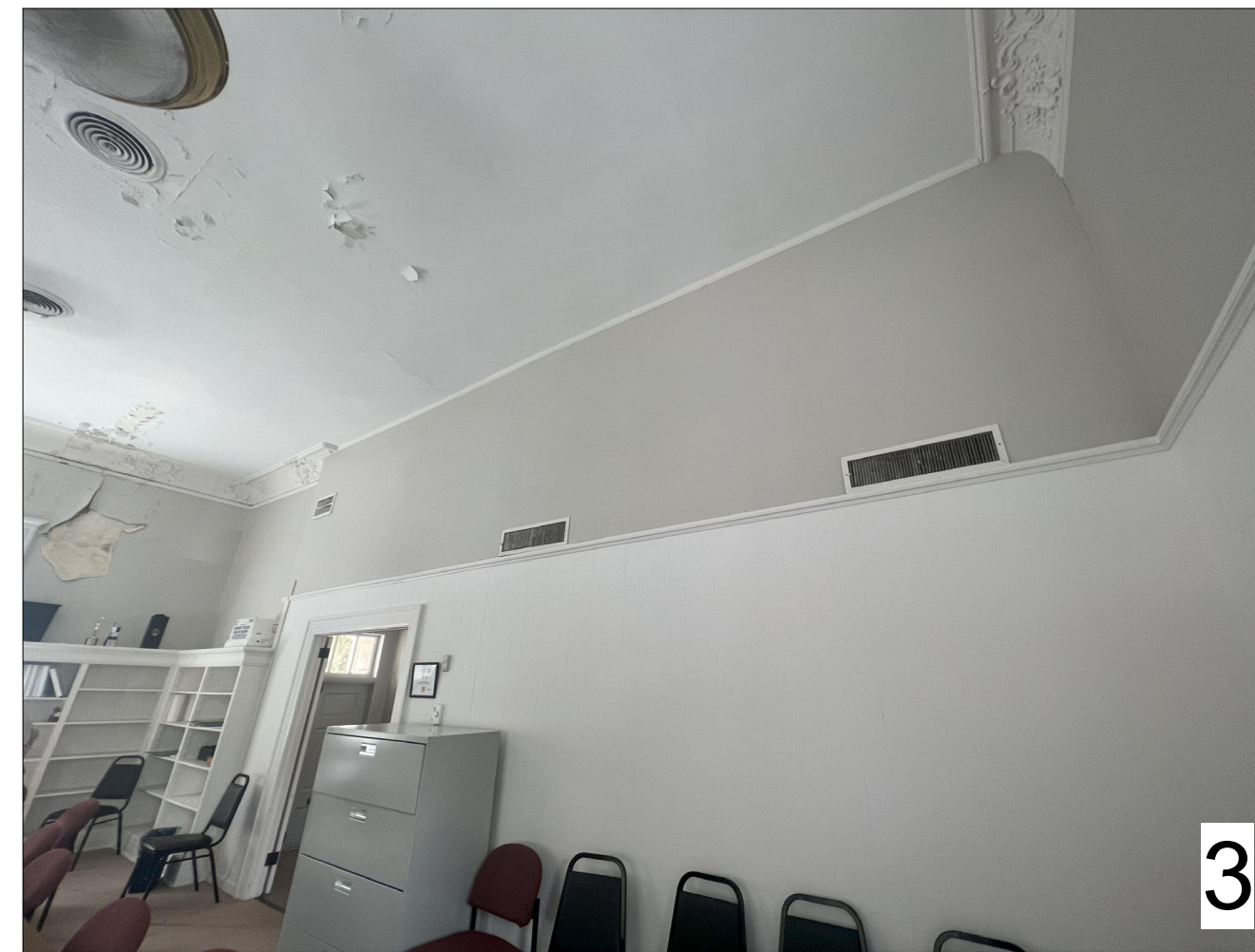
EXISTING CONDITIONS- CONFERENCE ROOM
