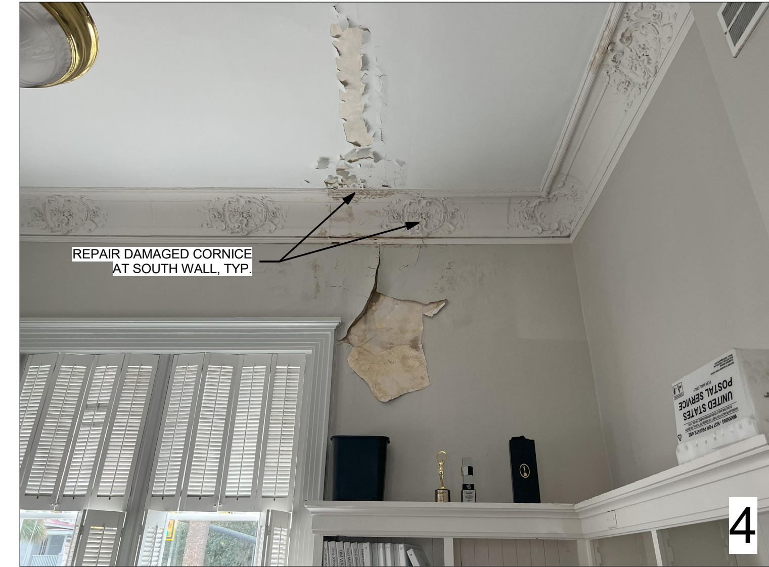
EXISTING CONDITIONS- CONFERENCE ROOM CEILING
