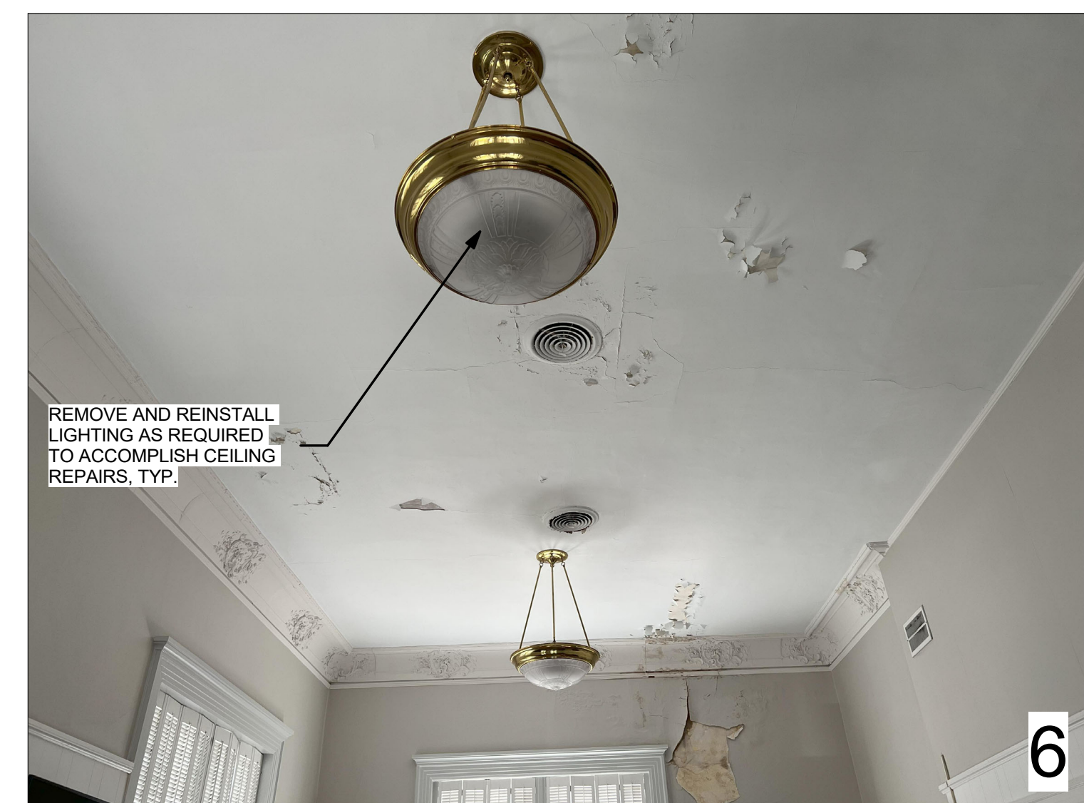
EXISTING CONDITIONS- CONFERENCE ROOM CEILING
