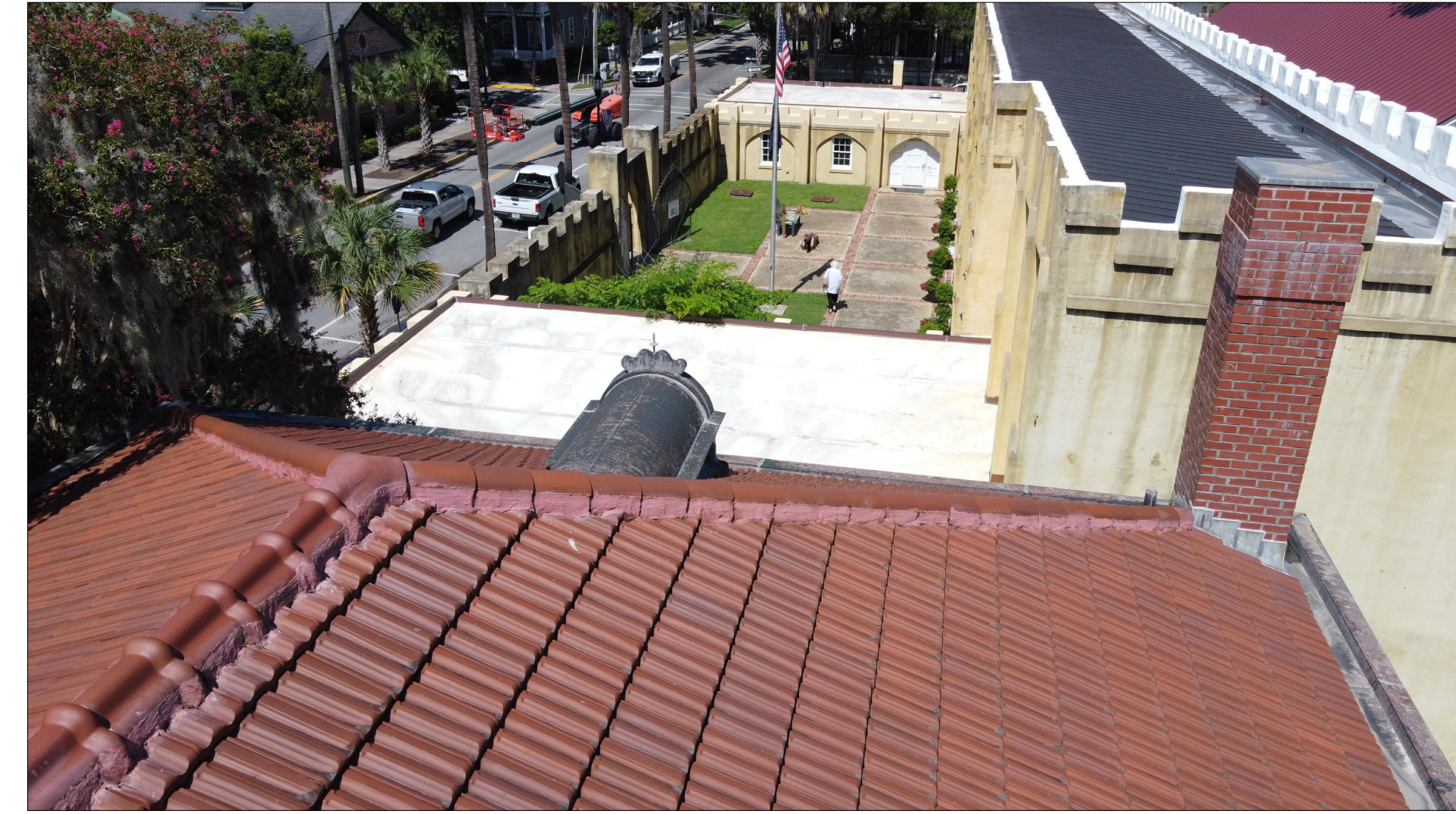
EXISTING CONDITIONS- DETAILED VIEW OF ROOF RIDGE AND HIP.
