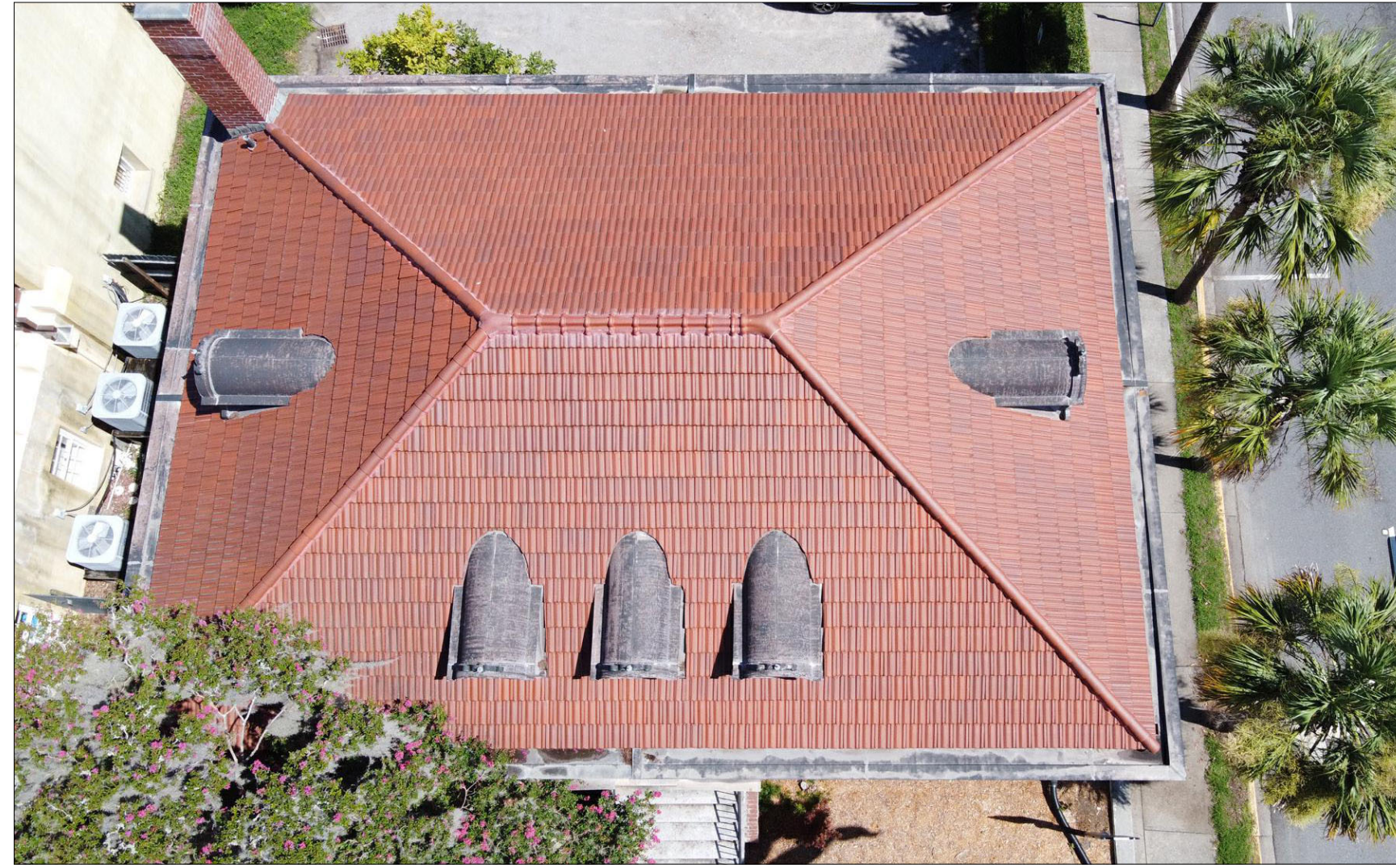
EXISTING CONDITIONS- OVERALL VIEW OF ROOF FROM ABOVE.
