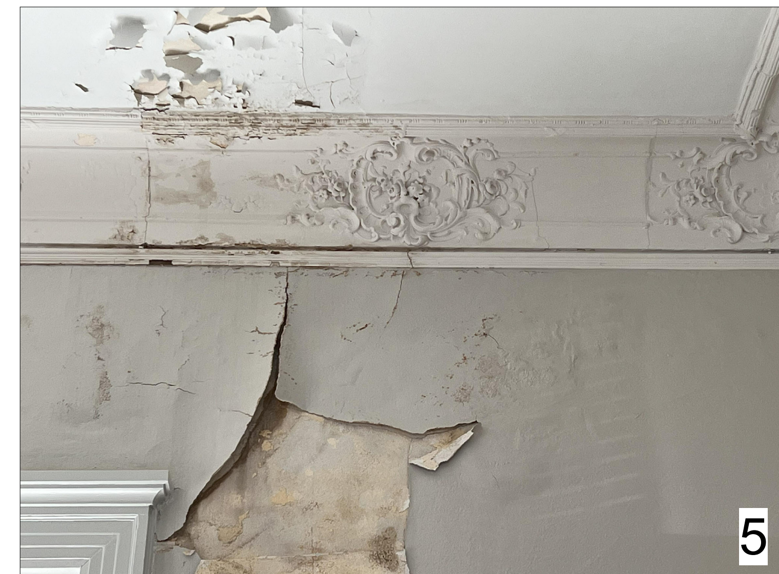
EXISTING CONDITIONS- CONFERENCE ROOM CEILING
