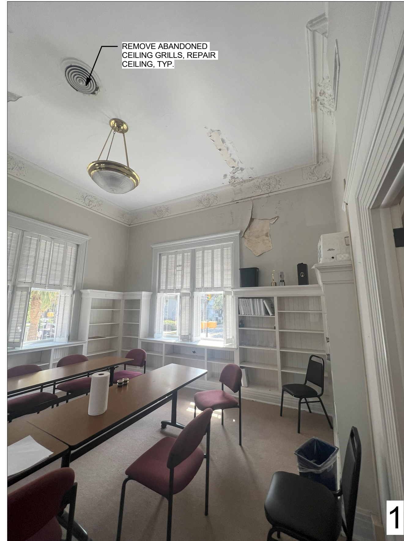
EXISTING CONDITIONS- CONFERENCE ROOM
