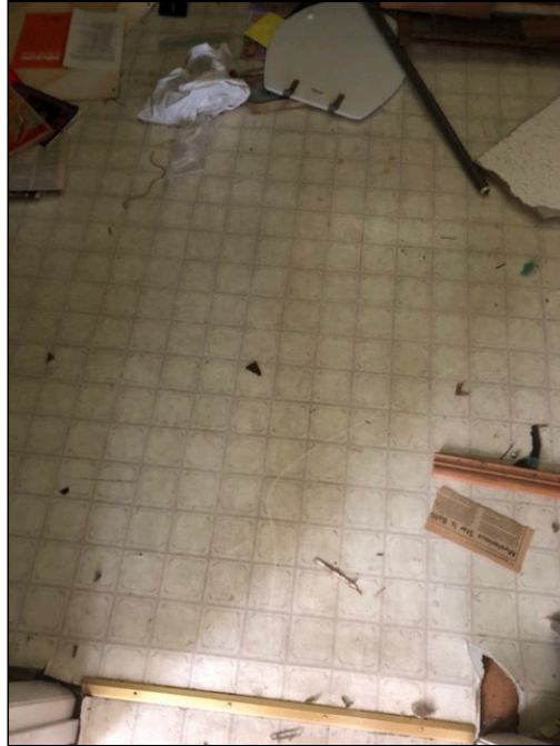
15 - Image of white 3" x 3" square pattern linoleum & mastic
