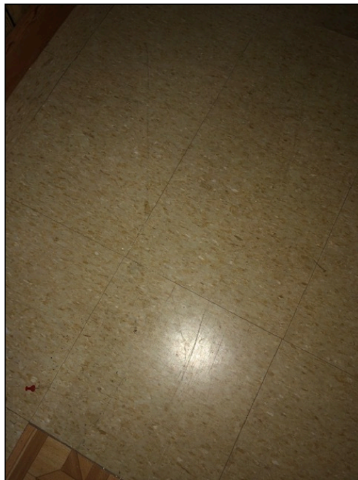
4 - Image of beige 12" x 12" Vinyl Floor Tile (VFT) & Mastic: (Sample ID 15-01,02,03)
