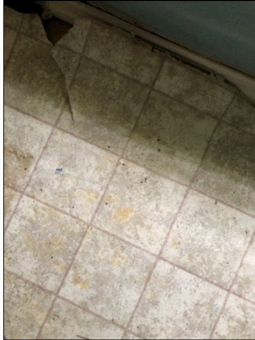
13 - Image of white square pattern linoleum & mastic
