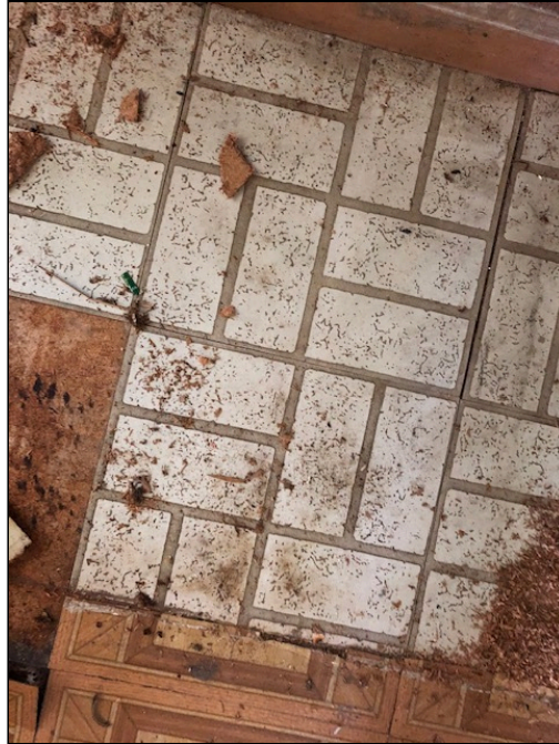
3 - Image of white brick pattern linoleum & mastic: (Sample ID 09-01,02,03)
