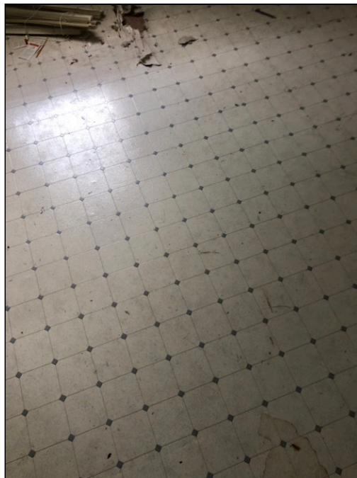
14 - Image of white & blue square pattern linoleum & mastic
