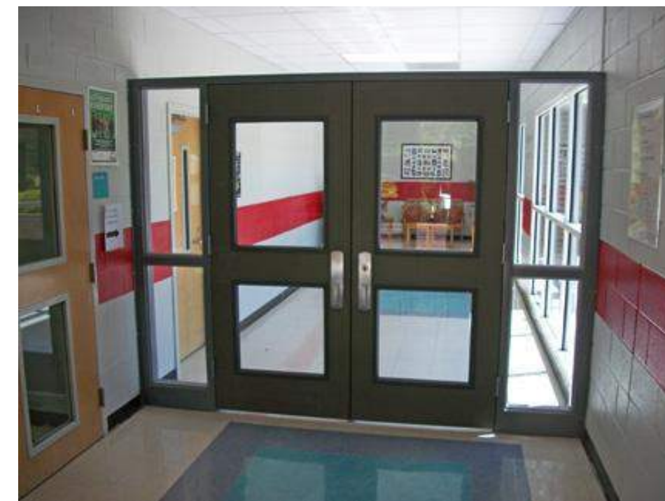
DOUBLE SECURITY DOOR ASSEMBLY (SIMILAR TO ABOVE) (COLOR TO BE SELECTED BY OWNER)
