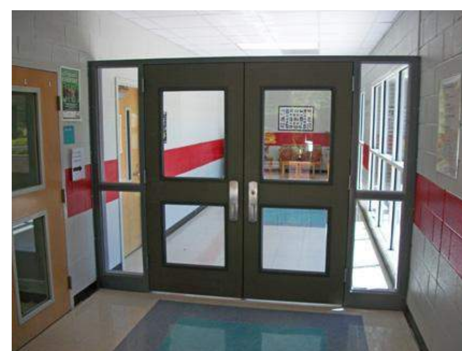
DOUBLE SECURITY DOOR ASSEMBLY (SIMILAR TO ABOVE)
