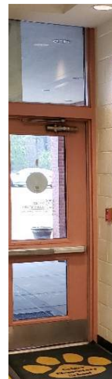
EXISTING ENTRANCE DOOR
