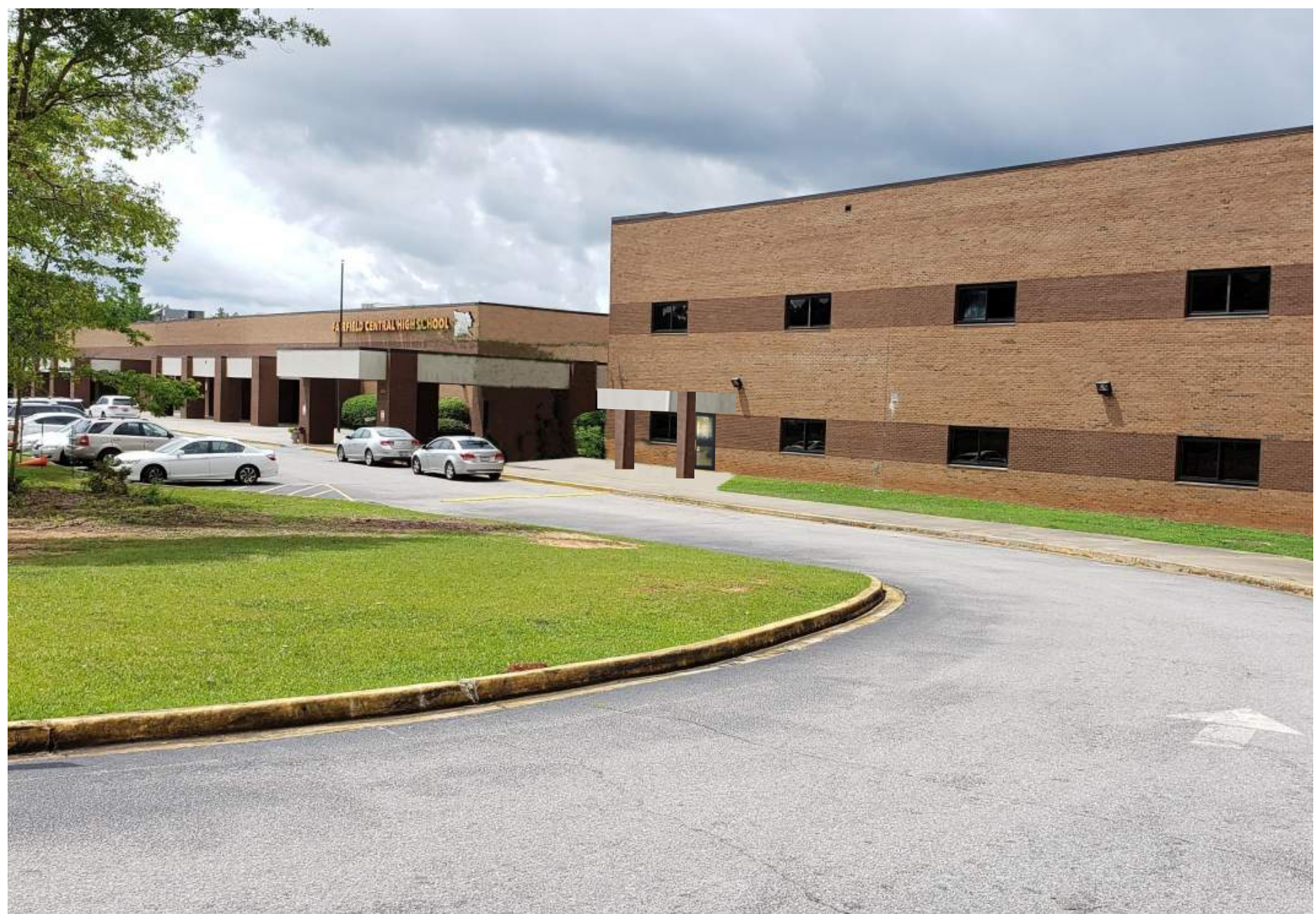
NEW VISITOR'S ENTRANCE
