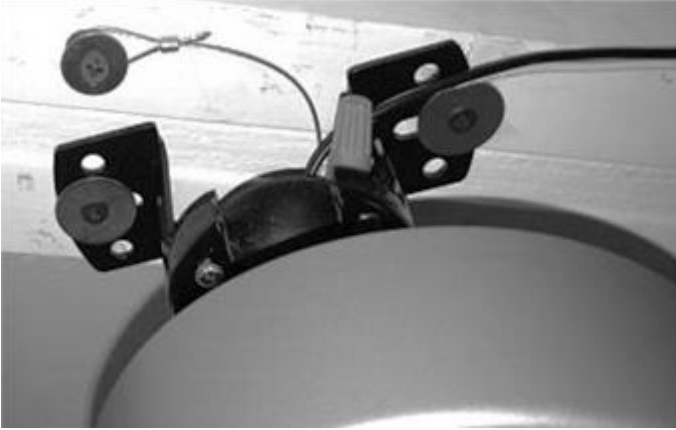
Photo 5: Safety cable attached near hanger
