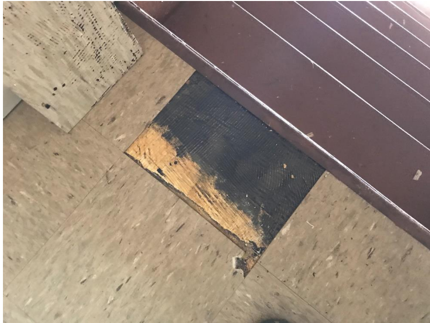
Photograph 7: View of 12x12 floor tile and black mastic.
