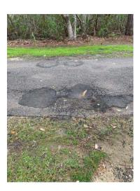
Site 006. Photo Taken: 11/10/2020 8:33 AM Site 6, 8'x6', collapsed pipe, 35' length, 18" diam
