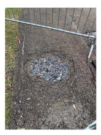
Site 005. Photo Taken: 11/10/2020 8:27 AM Site 5, 8'x6', collapsed pipe, 35' length, 18" diam
