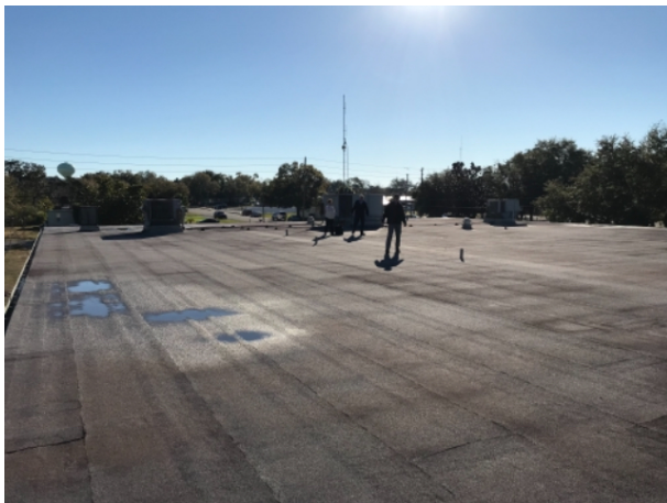
Observation Roof overview- NW corner looking East
