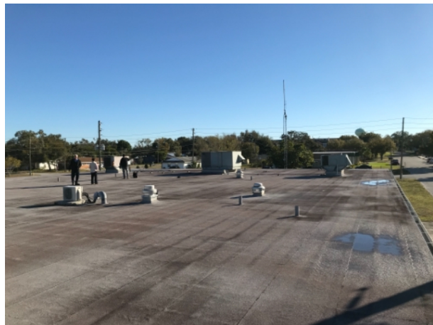
Observation Roof overview- SW corner looking East
