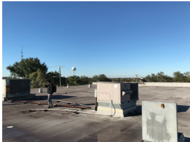
Observation Roof overview- NE corner looking West
