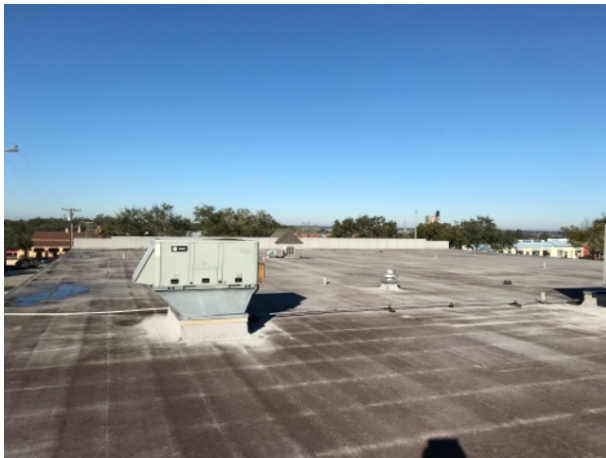
Observation Roof overview- SE corner looking West
