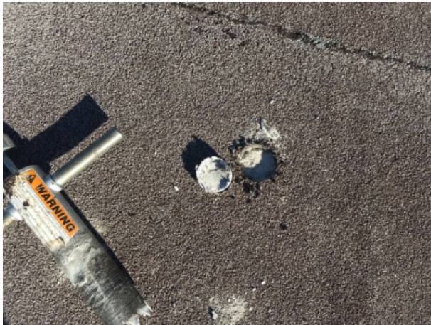
Observation Core cut- Modified Roof over Gypsum deck
