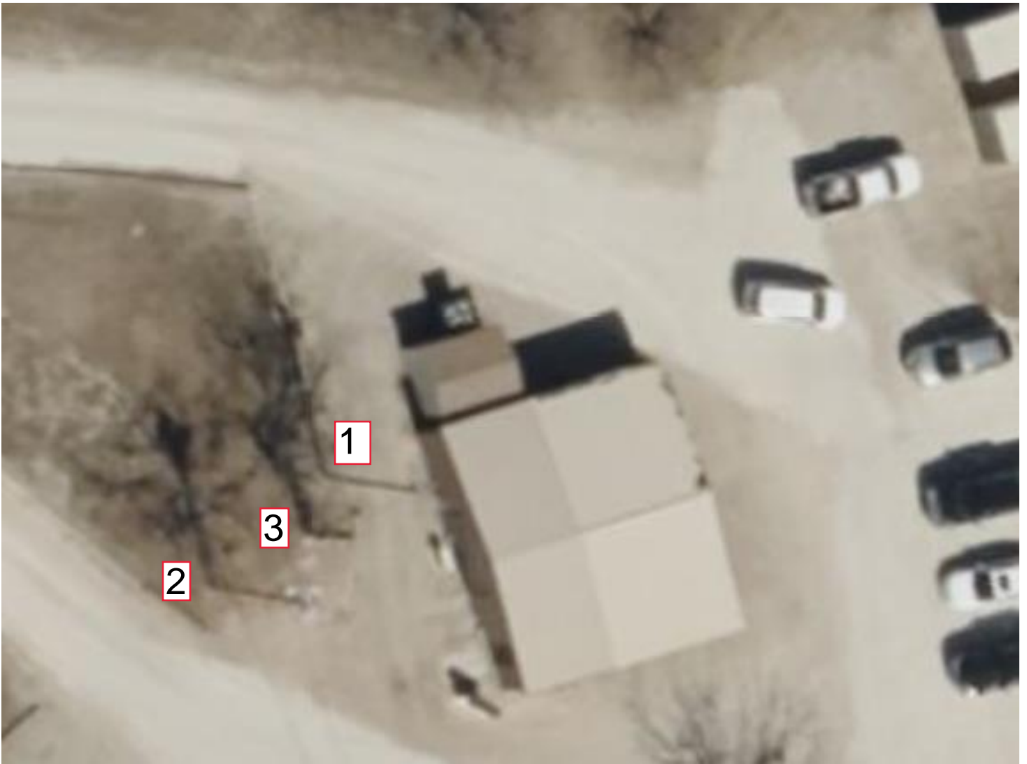
FIO - Construct New FOB North - Existing Power Poles
