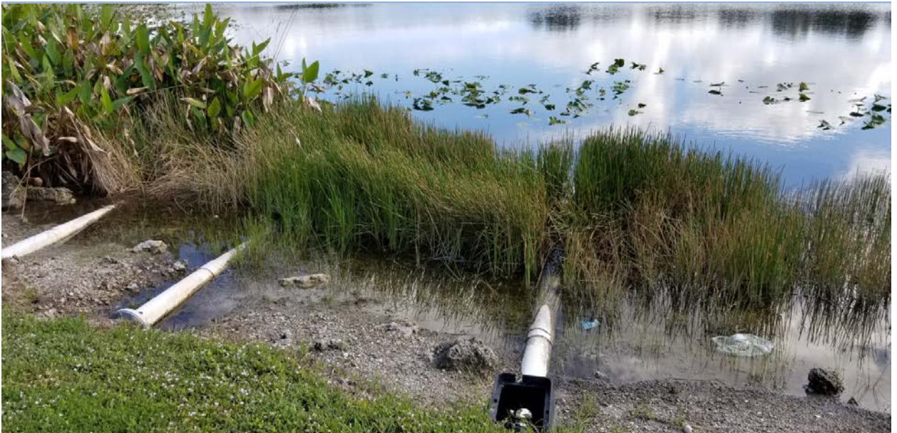
Figure 3 - Suction Lines for Existing pump stations 'A1' and 'B1' to be removed
