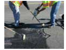
Fig. 5 Squeeze out sealer and spread with roller.
