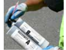
Fig. 4 Prepare sealer cartridges for use in sealer gun.
