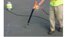
Fig. 3 After moving material aside, remove moisture from substrate
