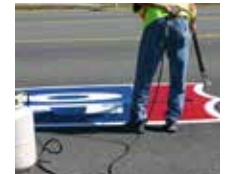
Fig. 7 Heat PreMark material
