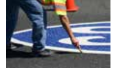
Fig. 2 Position marking to draw outline of application area
