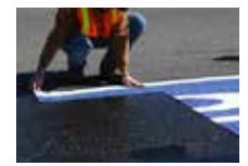
Fig. 6 Position PreMark® material according to diagram provided.
