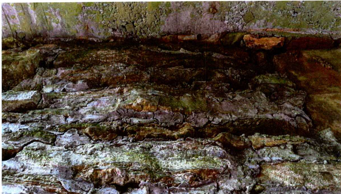
Photo 22. Cracking Through of Stones and Grout at South End of West Abutment, Looking Up
