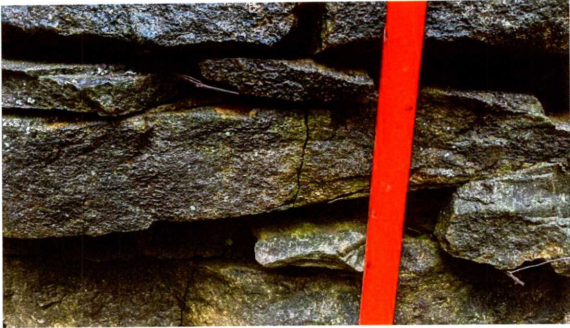
Photo 23. Stones Cracking at Southeast Quadrant. Wall also has sections of grout falling out.
