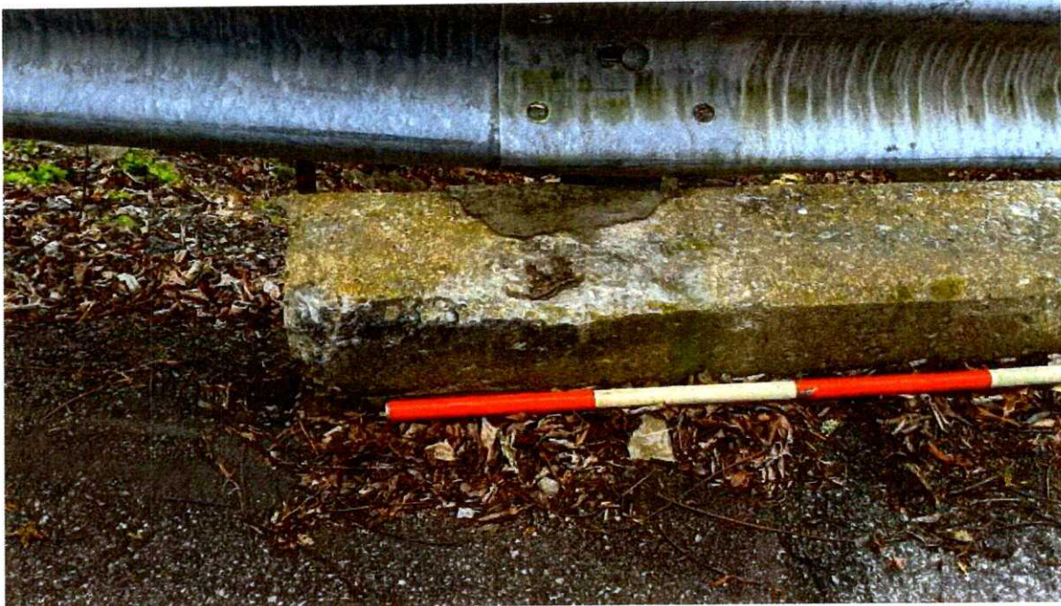
Photo 29. Spall and Patch at Southeast End of Curb
