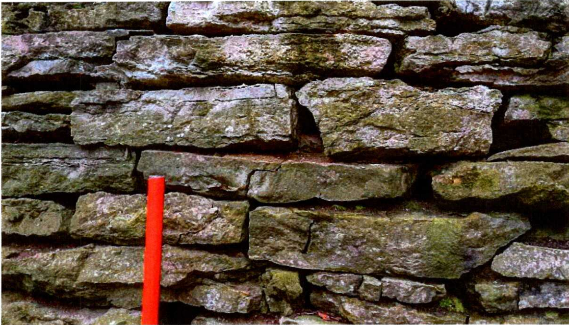
Photo 13. Cracking of Masonry Stones at Northwest Wall
