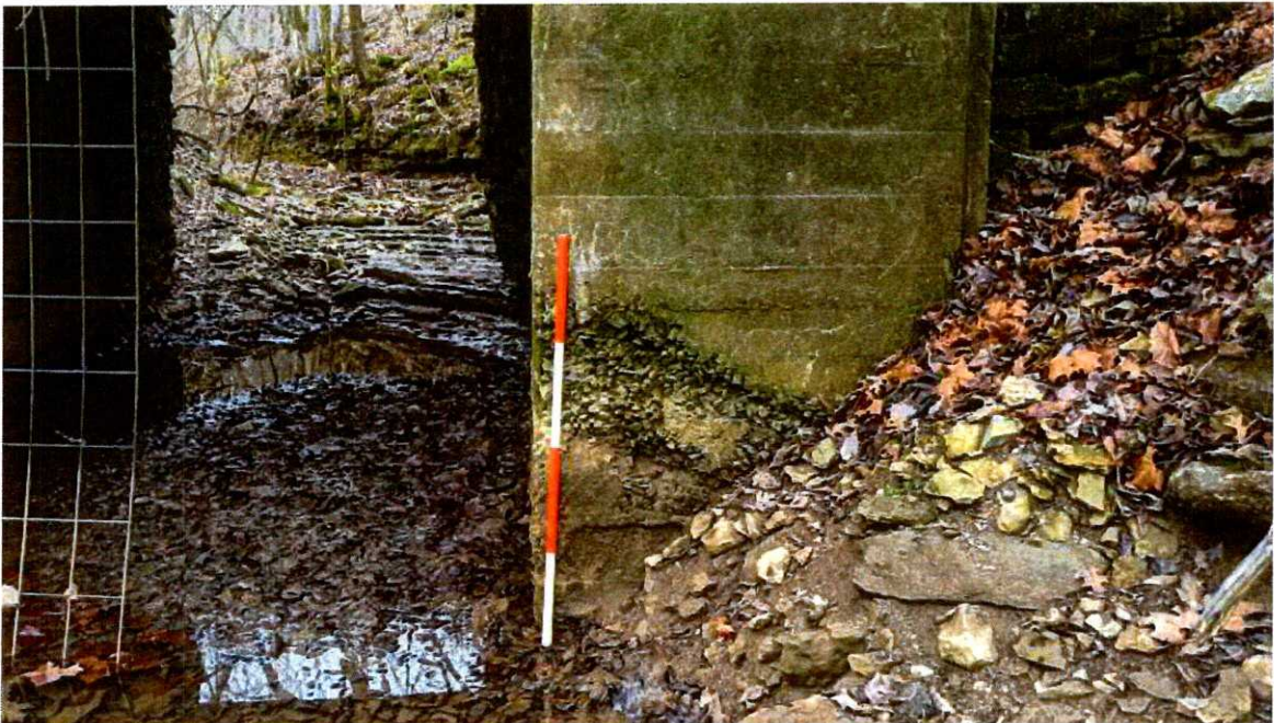
Photo 16. Honeycombing at North Face of West Abutment
