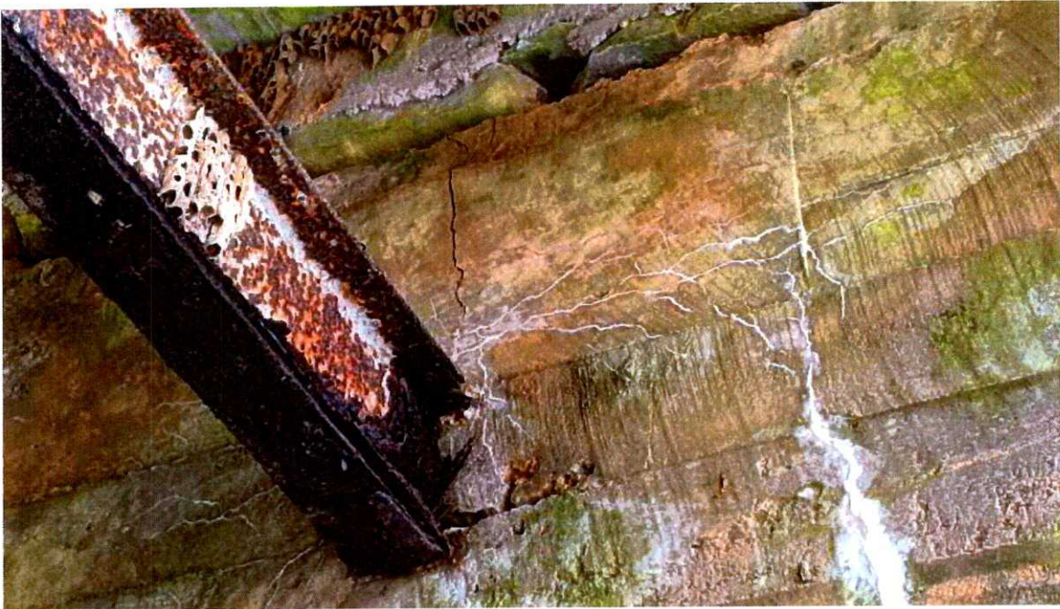
Photo 25. Vertical Crack at Top of West Abutment Leading to Middle Brace
