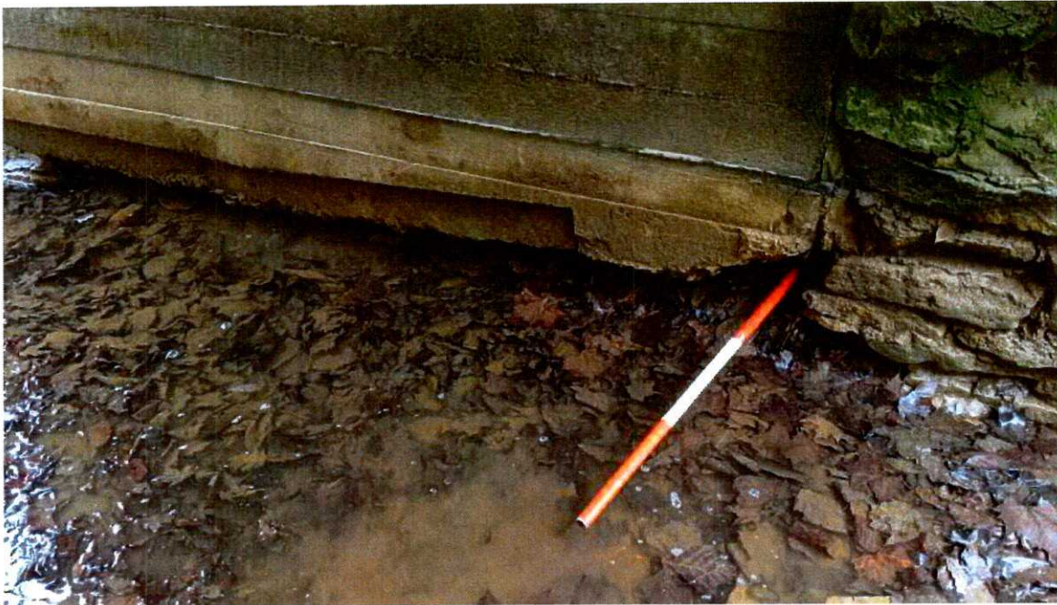
Photo 19. Undermining Along East Abutment, Up to 12" Along Section
