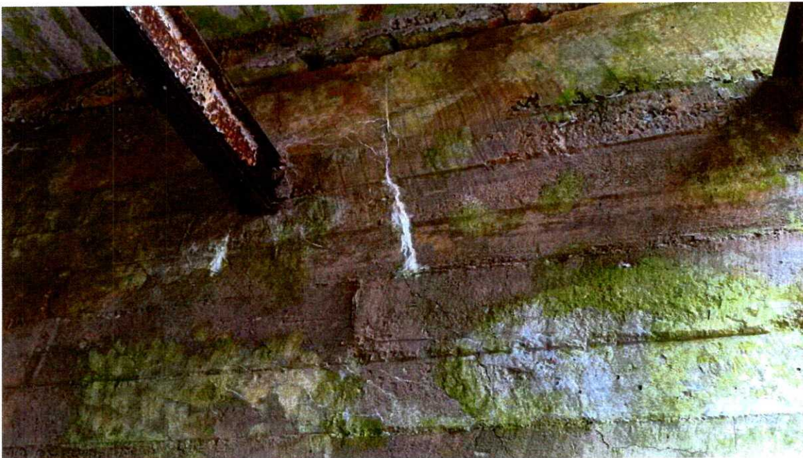
Photo 24. West Abutment, Middle Brace Corrosion with Section Loss and Adjacent Cracking with Efflorescence in Concrete.
