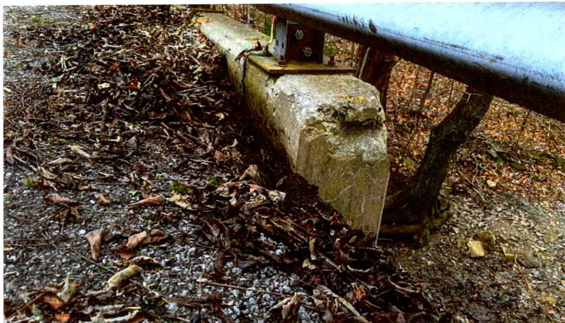
Photo 28. Spall at End of Curb at Northeast Corner and Debris Along North Gutterline
