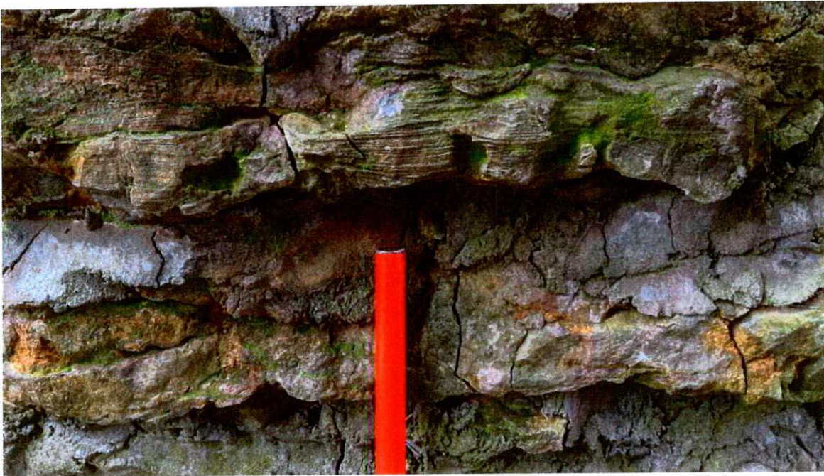
Photo 21. Cracking Through of Stones and Grout at South End of West Abutment
