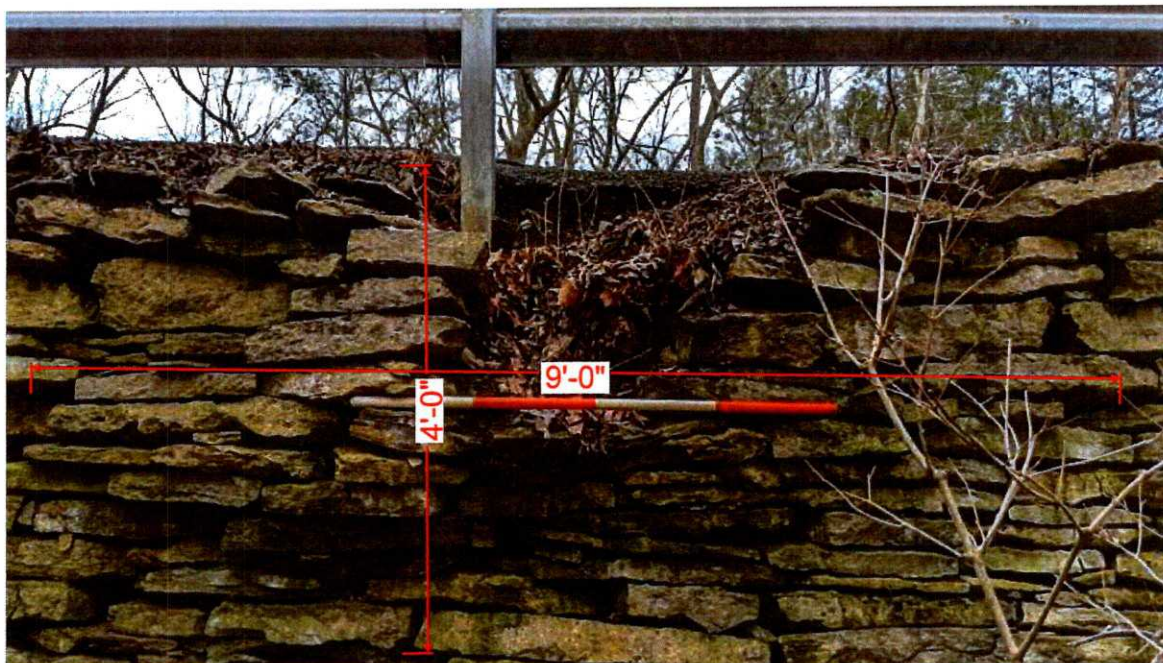
Photo 10. Masonry Wall Embankment at Northeast Quadrant Failing
