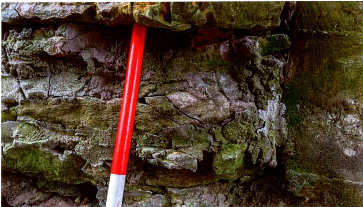
Photo 20. Cracking Through of Stones at South End of West Abutment
