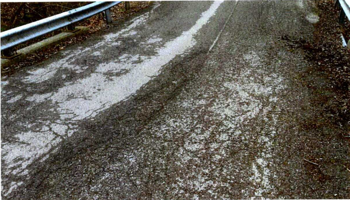
Photo 03. Asphalt Overlay - Minor Cracking
