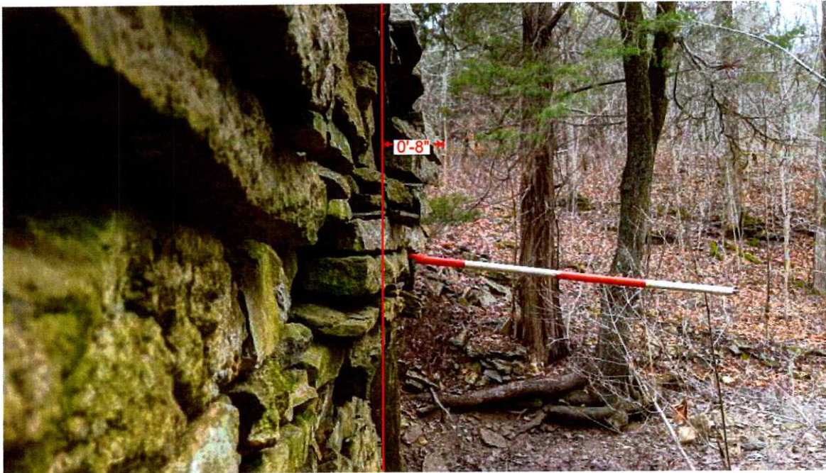
Photo 11. Masonry Wall Embankment at Northeast Quadrant Failing, Looking West Along Face of Wall.
