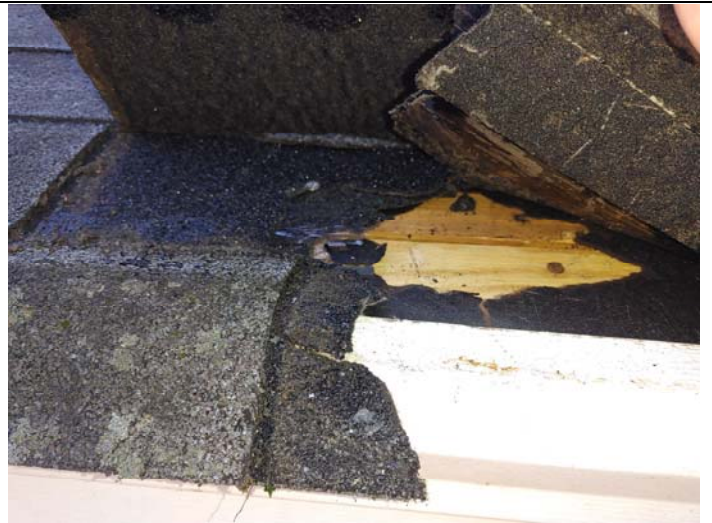
Photo 2 – Roof shingles (1 layer) & felt paper (1 layer)
