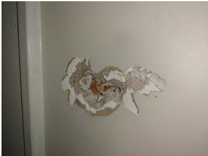
Photo 9 – Plaster with finish walls throughout
