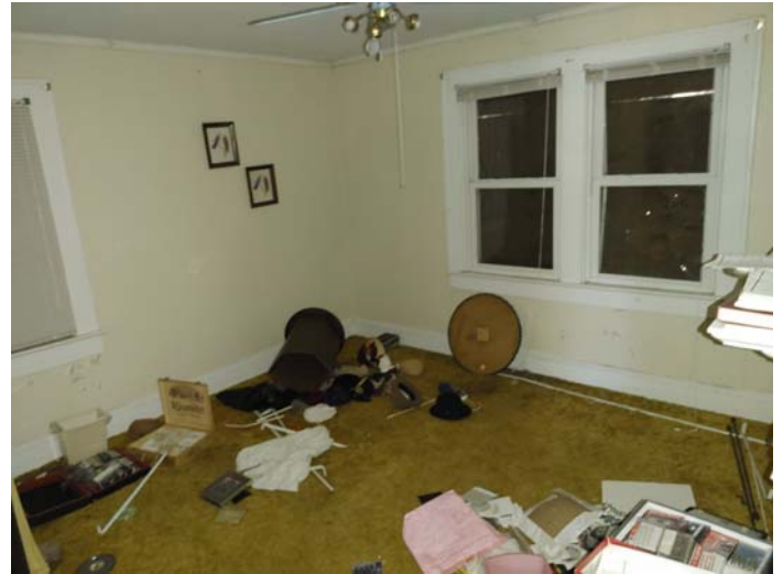
Photo 14 – Typical view of the house interior
