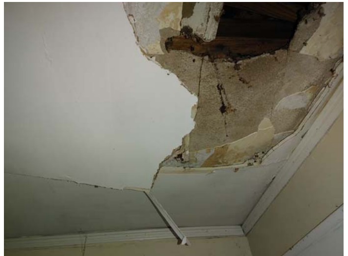
Photo 8 – Drywall with joint compound ceilings with plaster & finish located above
