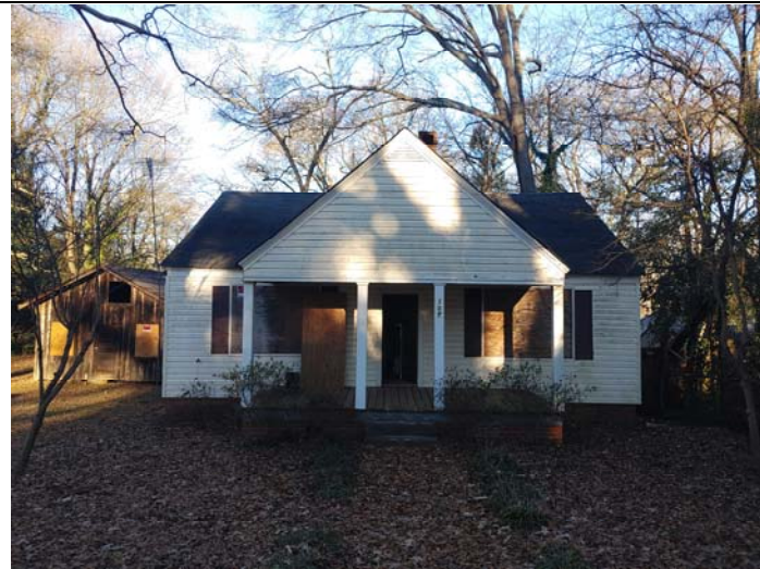
Photo 1 – 107 Amelia Street located in Spartanburg, South Carolina 29303
