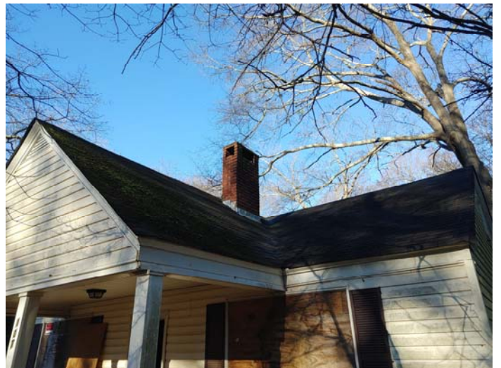
Photo 4 – View of 1 of 2 chimney's with tar – assumed positive
