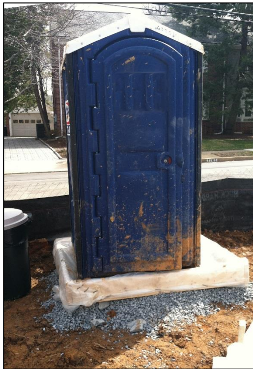
Portable toilet is located on level ground, and is inside secondary containment.
