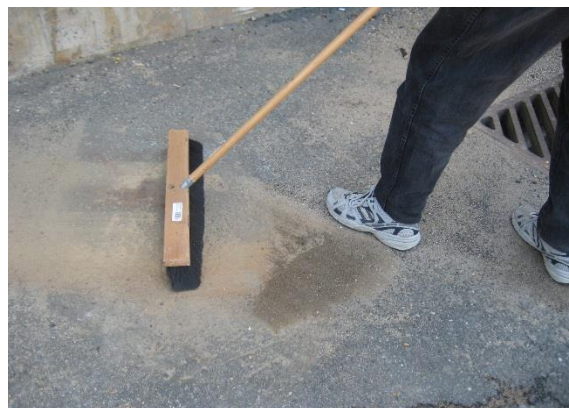
Example cleanup methods. Left photo: vacuuming. Right photo: sweeping debris away from the storm drain.
