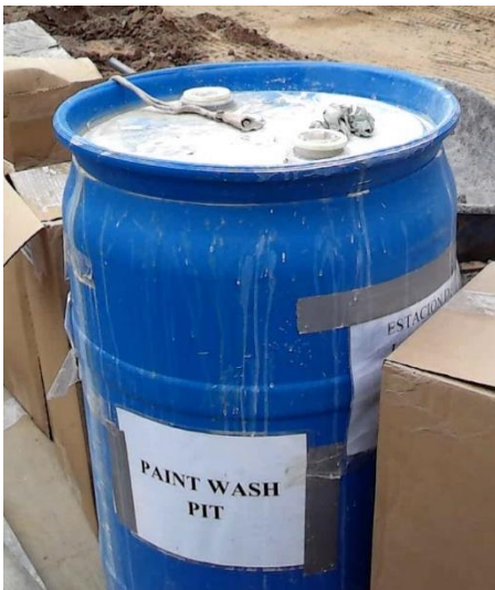
Example paint washout structure.
