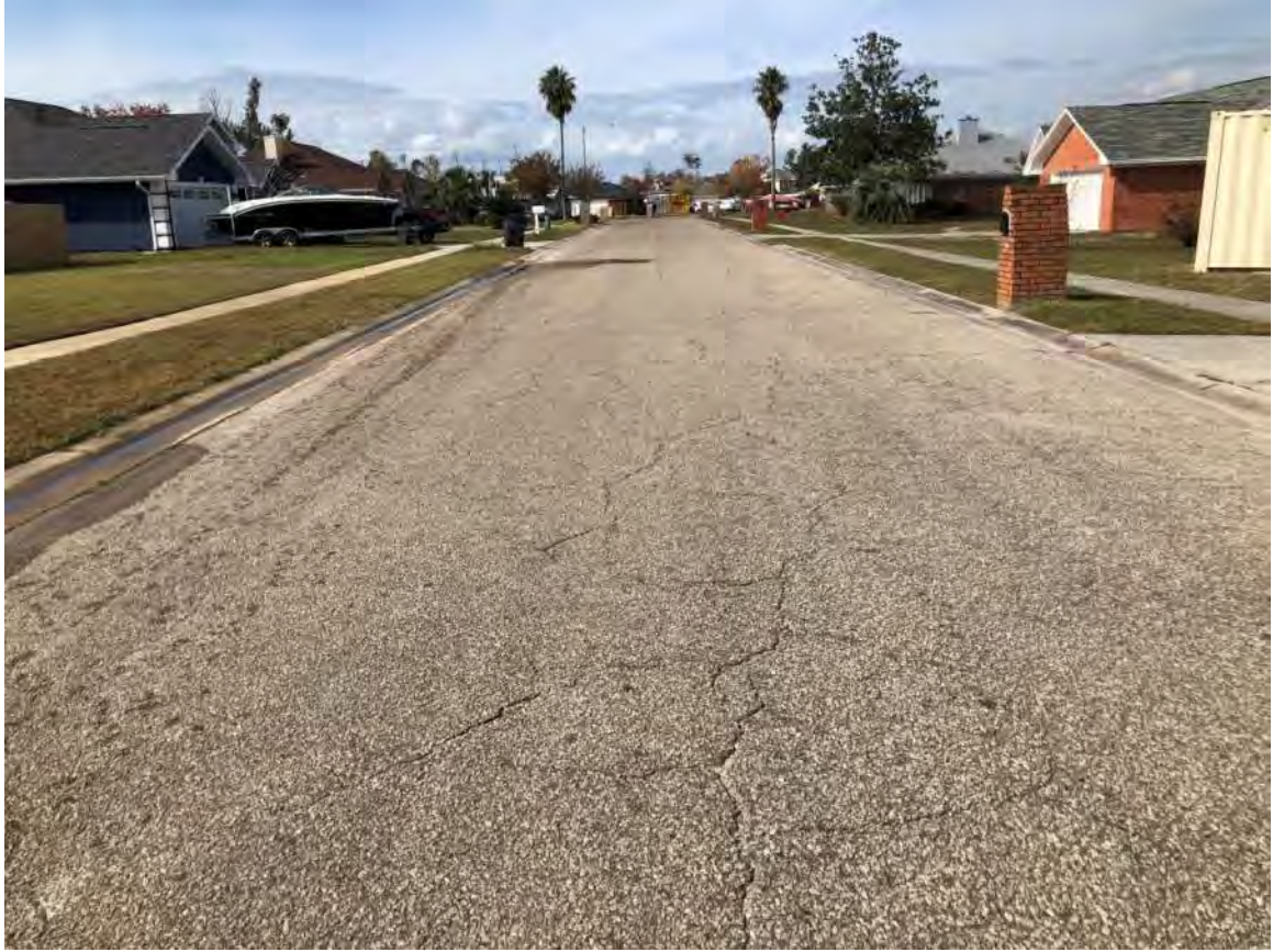
Ross Drive Core C-4 - General Roadway Conditions
