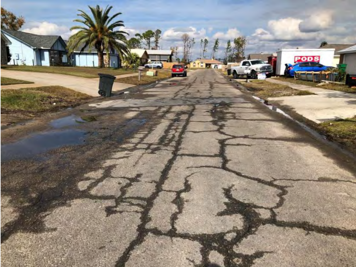
Ross Drive Core C-1 - General Roadway Conditions
