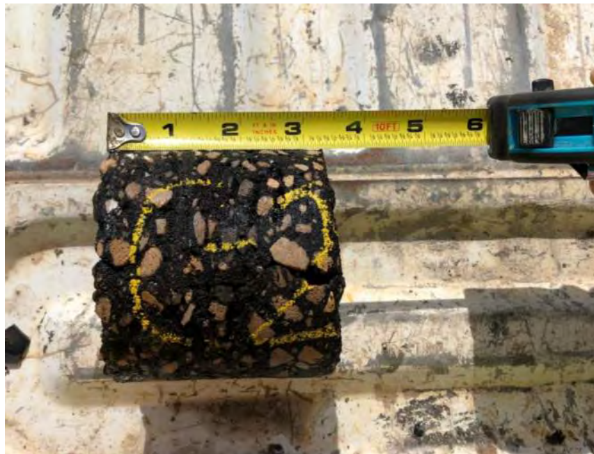
Core C-2 - Approximately 3¼ Inches of Asphaltic Concrete
