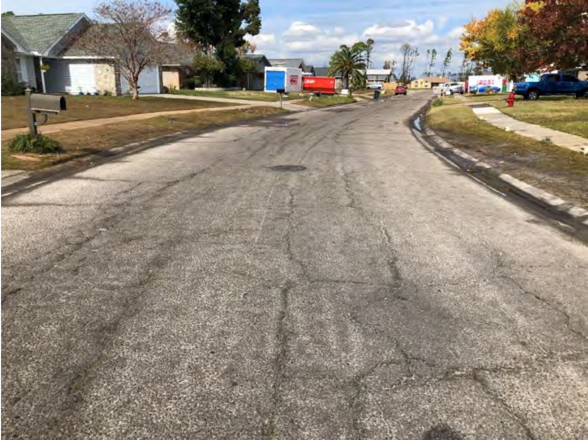
Ross Drive Core C-2 - General Roadway Conditions
