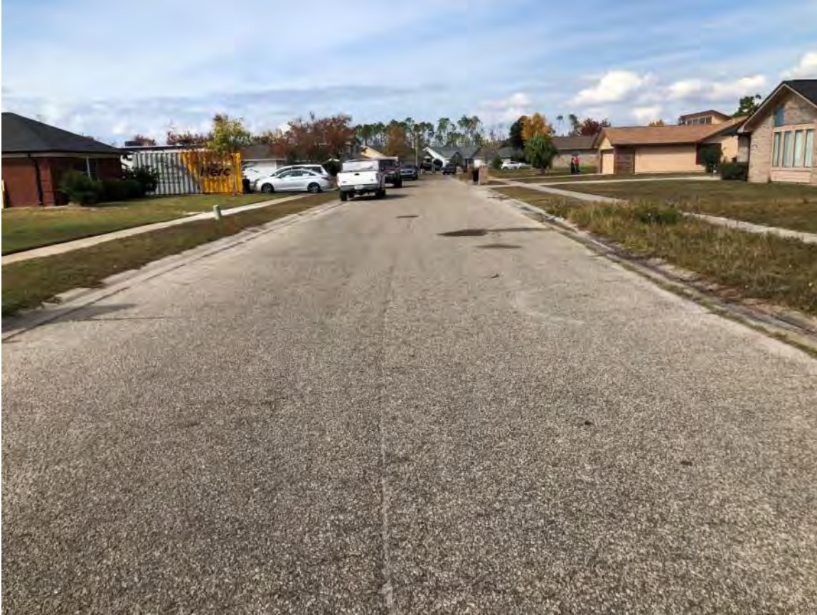
Ross Drive Core C-3 - General Roadway Conditions
