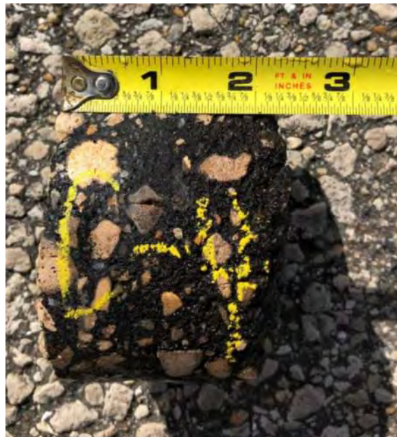
Core C-4 - Approximately 2\frac{1}{4} Inches of Asphaltic Concrete
