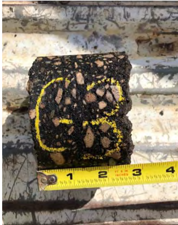
Core C-3 - Approximately 2\frac{5}{8} Inches of Asphaltic Concrete
