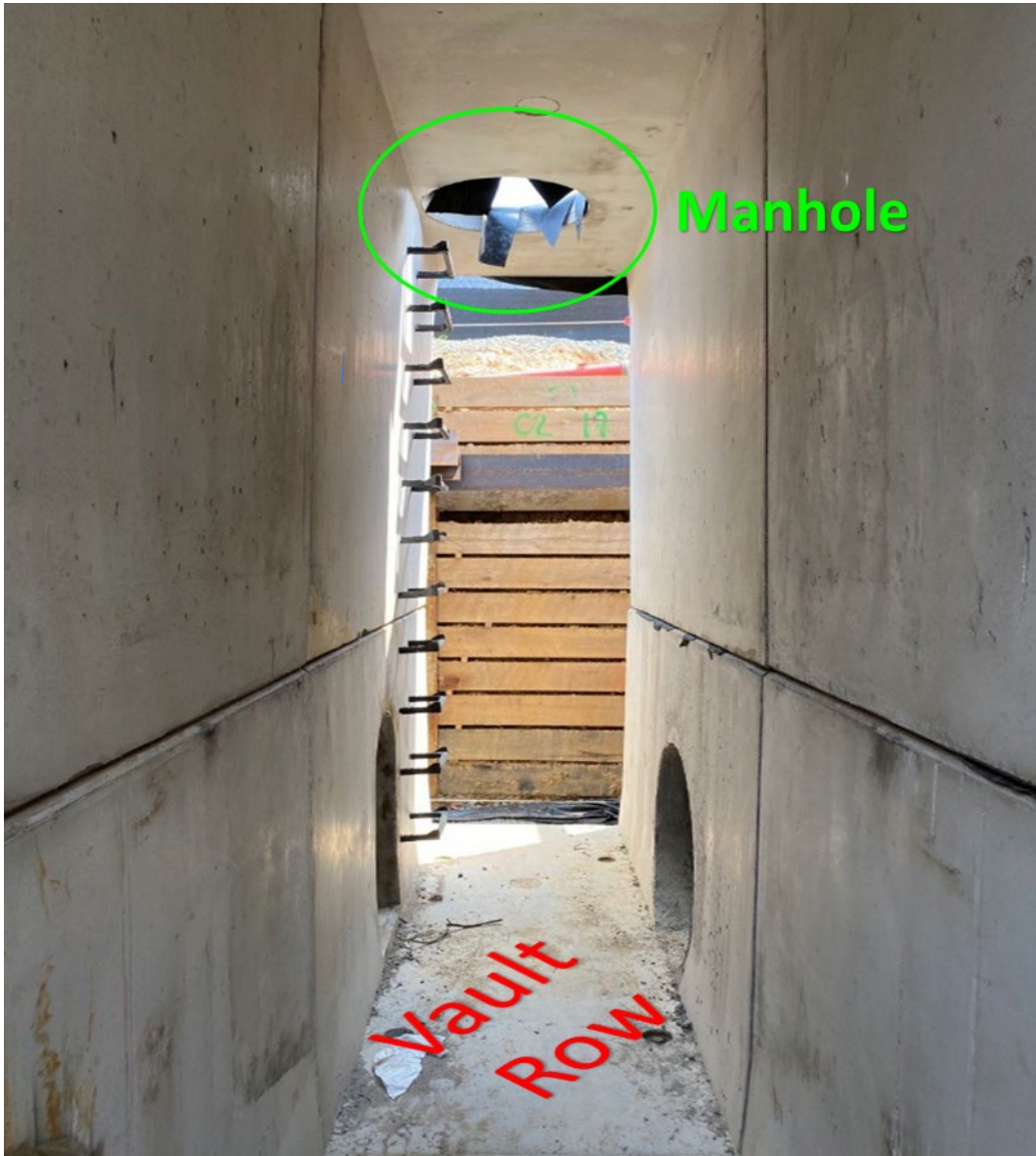
Figure 4. The underground detention vault access manhole
