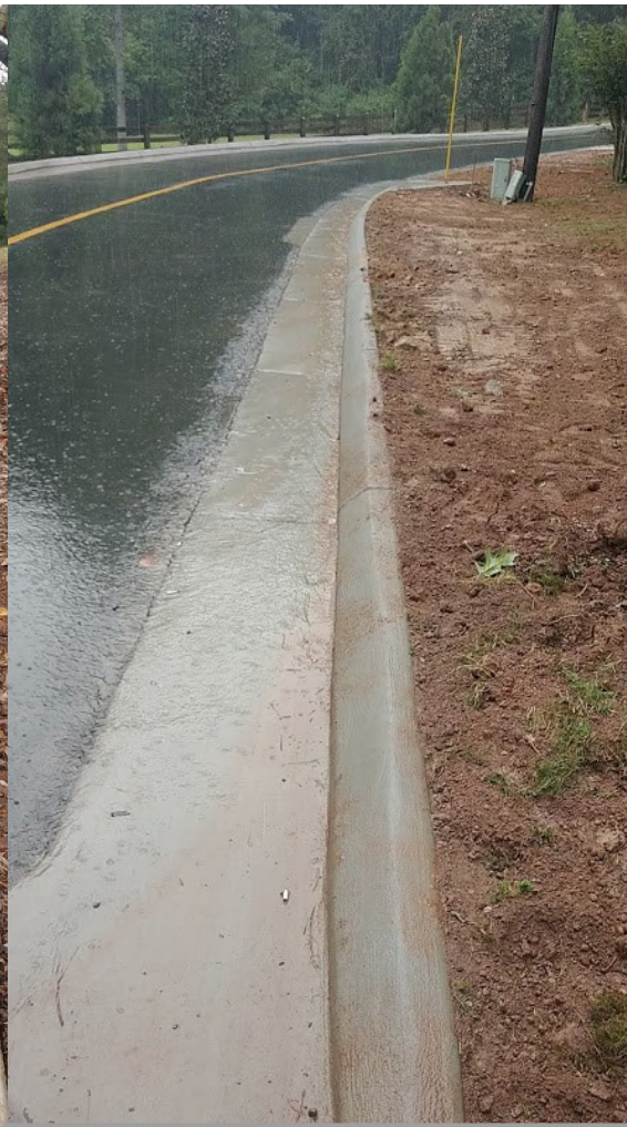
Grade and install approximately 1654' of two-foot 3500 psi concrete drivable surface 8" depth minimum on each side of the roadway with Type 7 curb and gutter.
