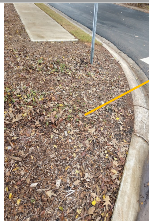
Install 1 ADA accessible ramp and extend existing sidewalk at the corner of Dobbs Rd and Melanie Ln approximately 12' x 5' area.
