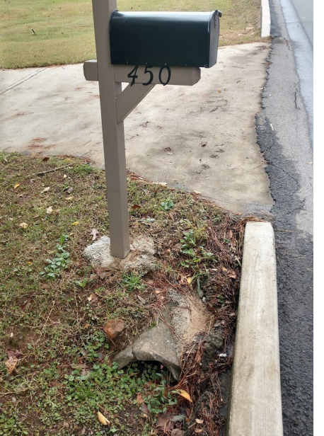
Install 80 linear feet of 18" HDPE stormwater pipe and remove existing head-wall.
