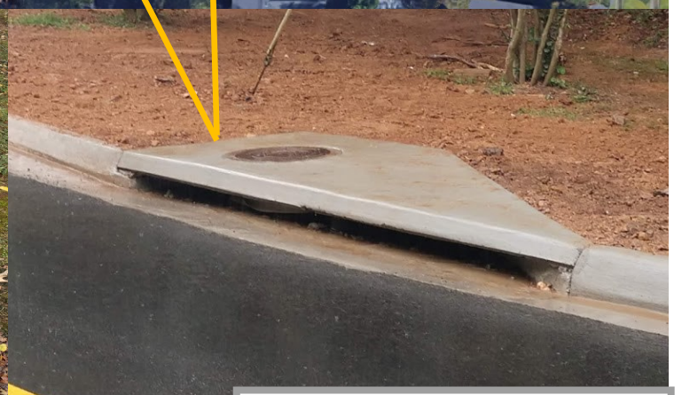
Construct 2 concrete poured in place or precast catch basins with throats and accessible tops to match existing on Dobbs Rd. To the west of 500 Dobbs Rd and at the site of the current headwall.
