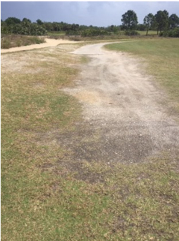
Item 5. Hole #16 demo 8 lf and new 75 lf
