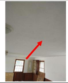
**Photo 1 HA 02:** Asbestos-Containing Textured Ceiling Material (Garage Ceiling)
