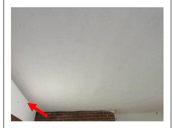
**Photo 4 HA 23:** Asbestos-Containing Joint Compound within the Drywall system (<0.09% by Composite with Point Count, 1.5% Chrysotile In Joint Compound Layer)
