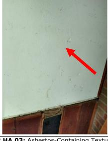
**Photo 2 HA 03:** Asbestos-Containing Textured Wall Material (Garage Walls)
