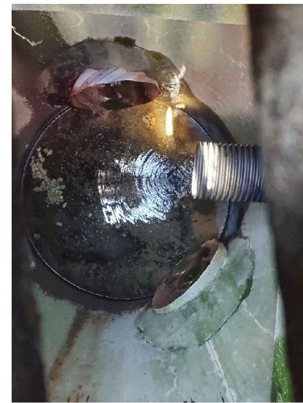
INSIDE EXISTING CATCH BASIN WITH HDPE PIPE
