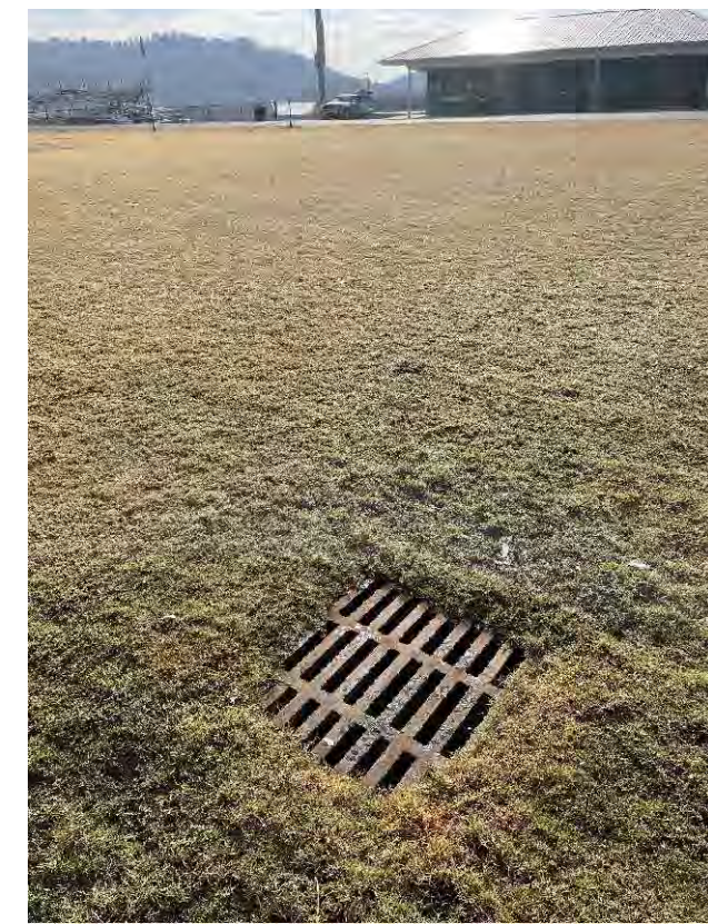
EXISTING CATCH BASIN - WEST END OF FIELD
